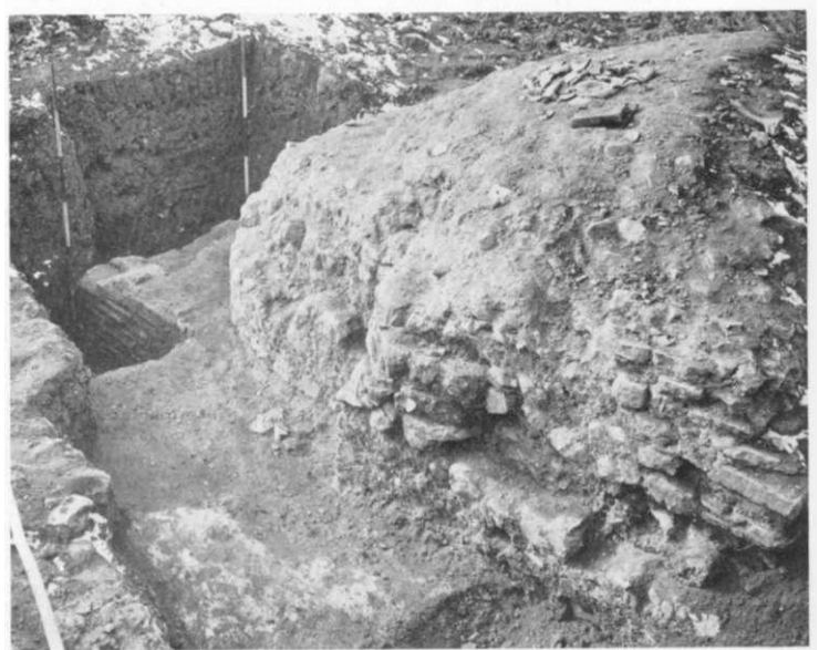
C. Entrance to Norman forebuilding, showing part of Roman brick pedestal beneath (in background). [148], p. 176.
