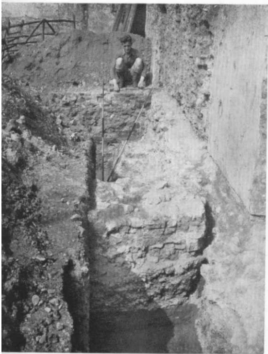
C. Excavation of foundations of Bastion 4. [147], p. 50.
