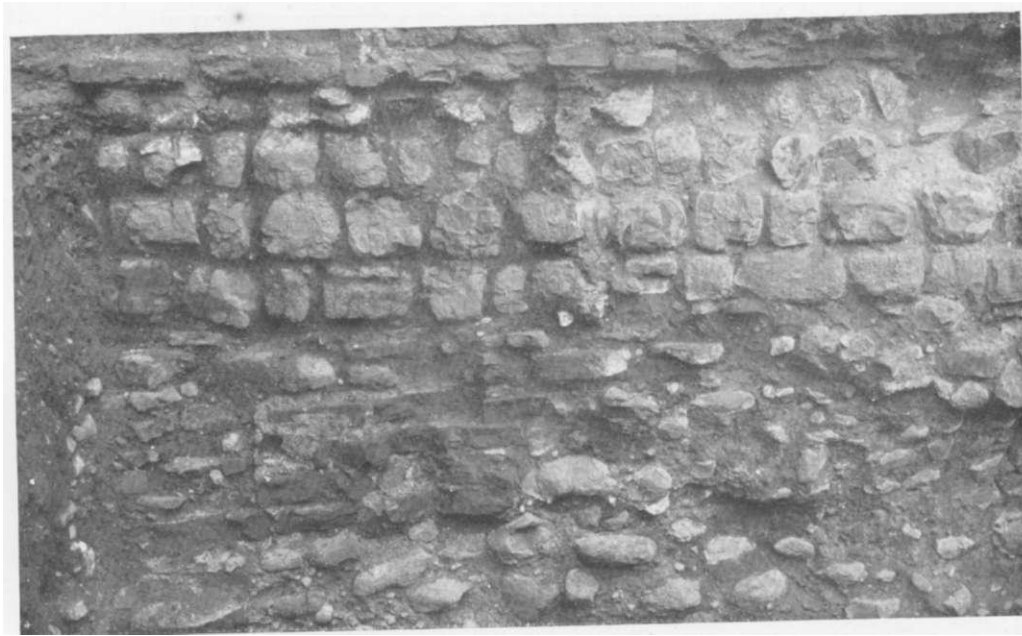
A. West face of cross-wall in Keep, showing tiling in the Roman work beneath. [34], p. 167.
