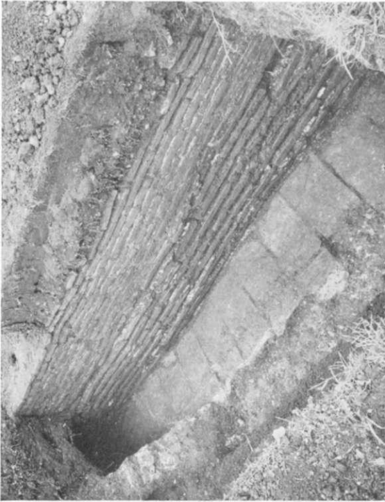
A. Drain, near NE. Gate, showing construction. [39], pp. 88, 89.
