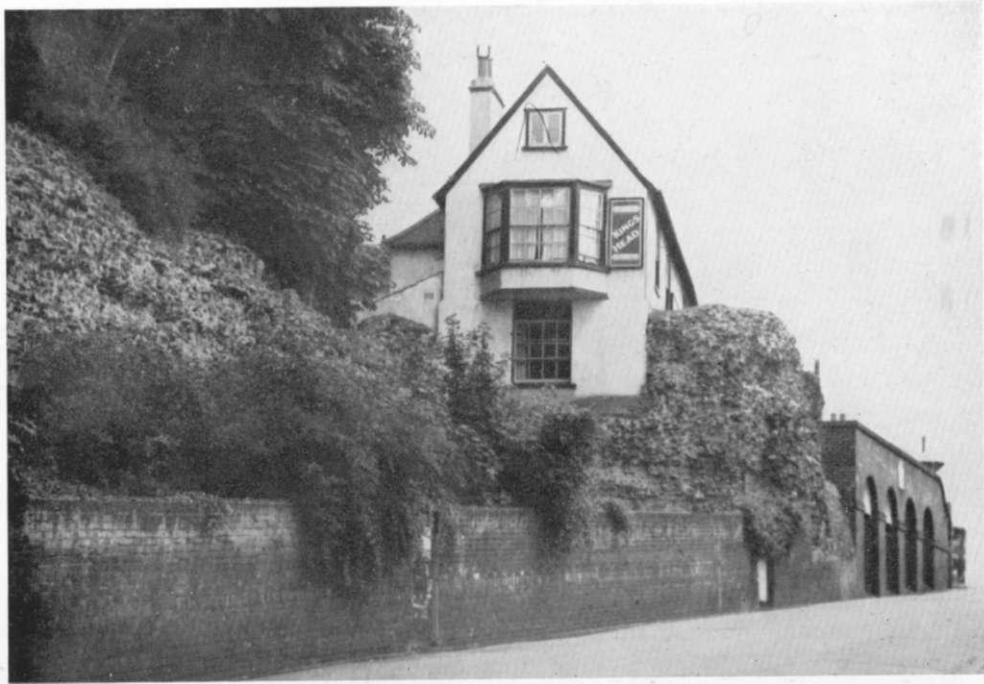
A. Roman town wall and north tower of Balcerne Gate.
