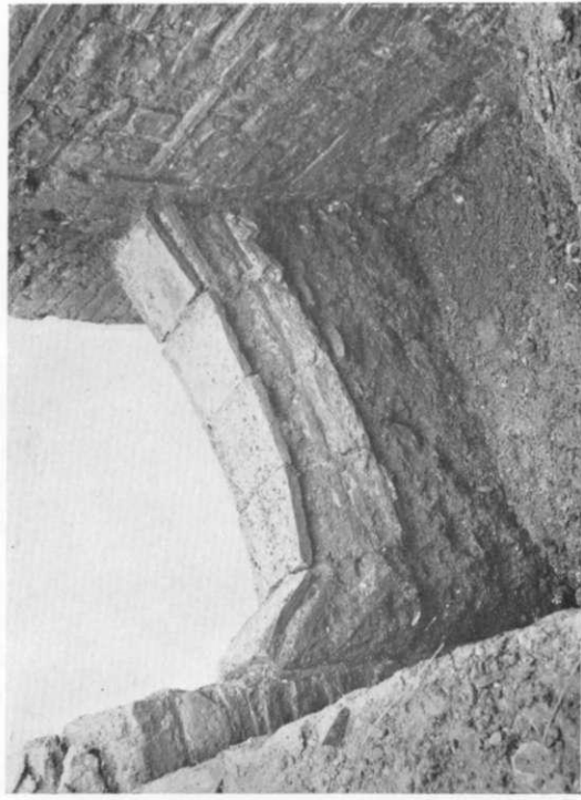
C. Entrance to underground room of 'Mithraeum', showing blocking masonry. [39], p. 108.
