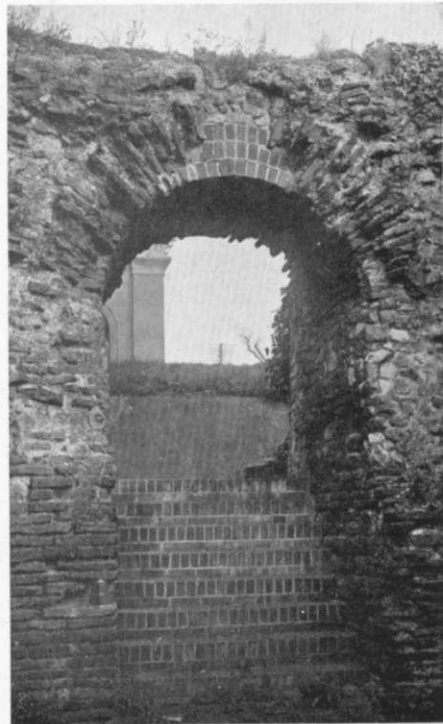
C. Balcerne Gate, doorway of south guardroom, looking east.
