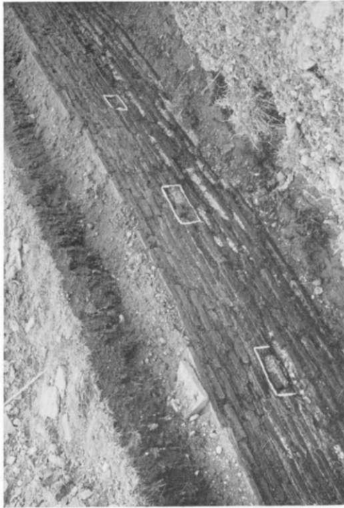
B. Drain, showing difference between upper and lower parts, and line of holes filled with mortar. [39], p. 88.
