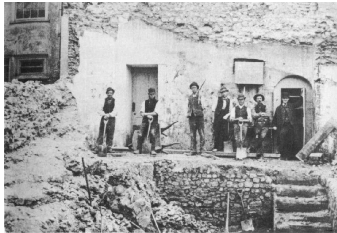
Above: Demolition of the Norman stone house near Jacklin's cafe in 1886. Photograph by J.C. Shenstone. (Courtesy of the Colchester and Essex Museum.)
