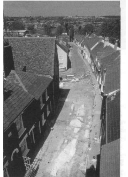
The foundations exposed in Maidenburgh Street in 1984 are parts of the outer wall of the theatre.
