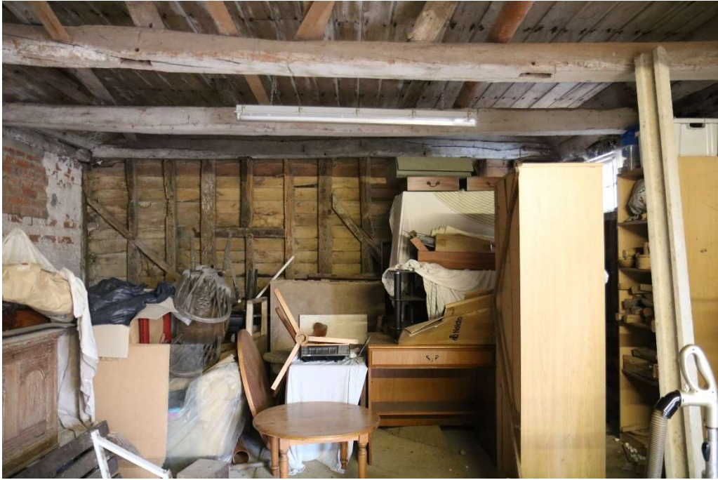
Photograph 11 Detail of wall-framing of south-eastern wall. Photograph taken facing east south-east.
