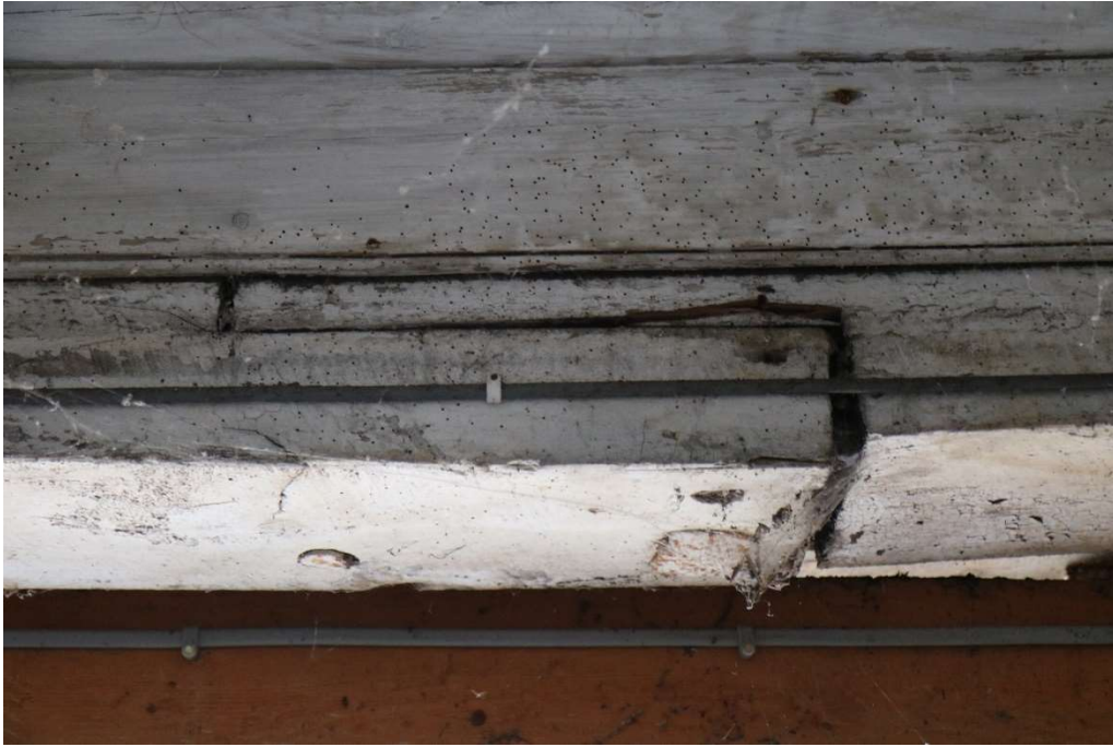
Photograph 13 Detail of south-western wall-plate scarf-joint. Photograph taken facing south south-west.
