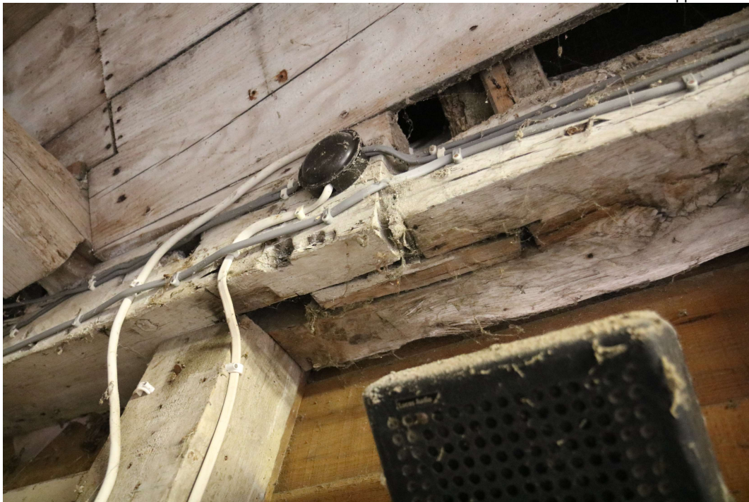
EEX60095_PhotoGraph_025 Detail of south-western wall-plate scarf-joint. Photograph taken facing south.
