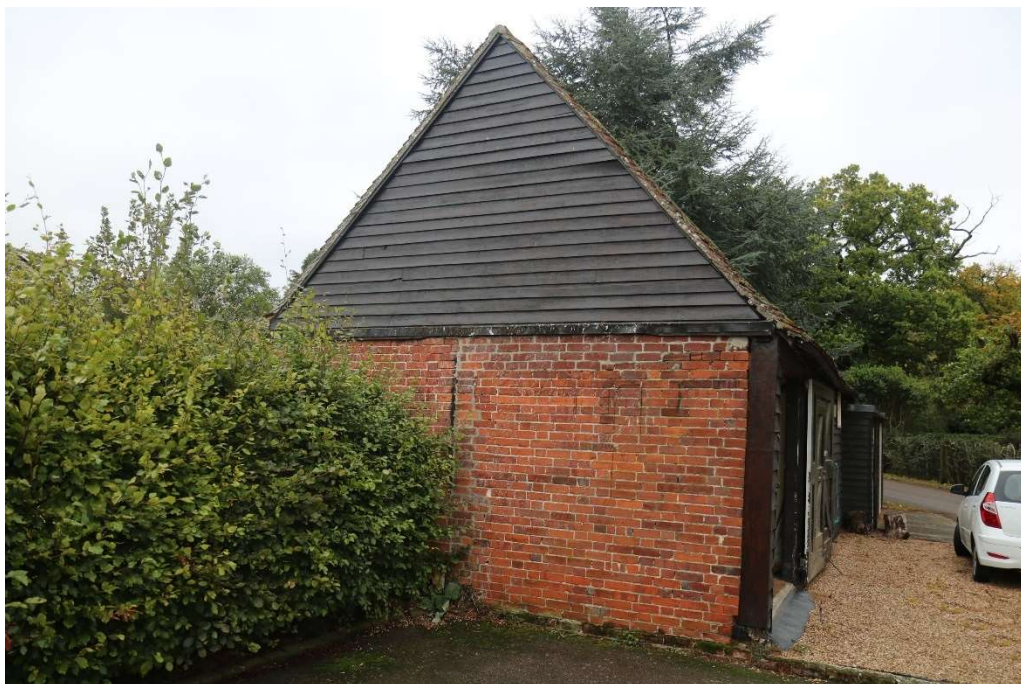
Photograph 3 North-western elevation. Photograph taken facing east.
