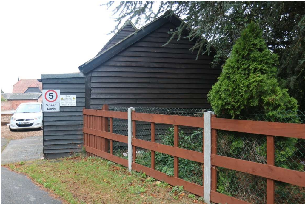
Photograph 5 South-eastern elevation. Photograph taken facing north-west.
