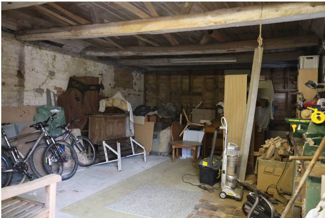
EEX60095_PhotoGraph_011 Interior of coach house. Photograph taken facing north-east.
