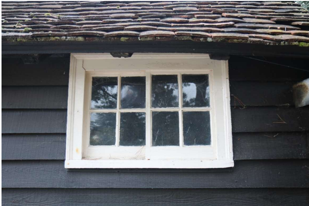
Photograph 2 Detail of Yorkshire sash-window on south-western elevation. Photograph taken facing north-east.
