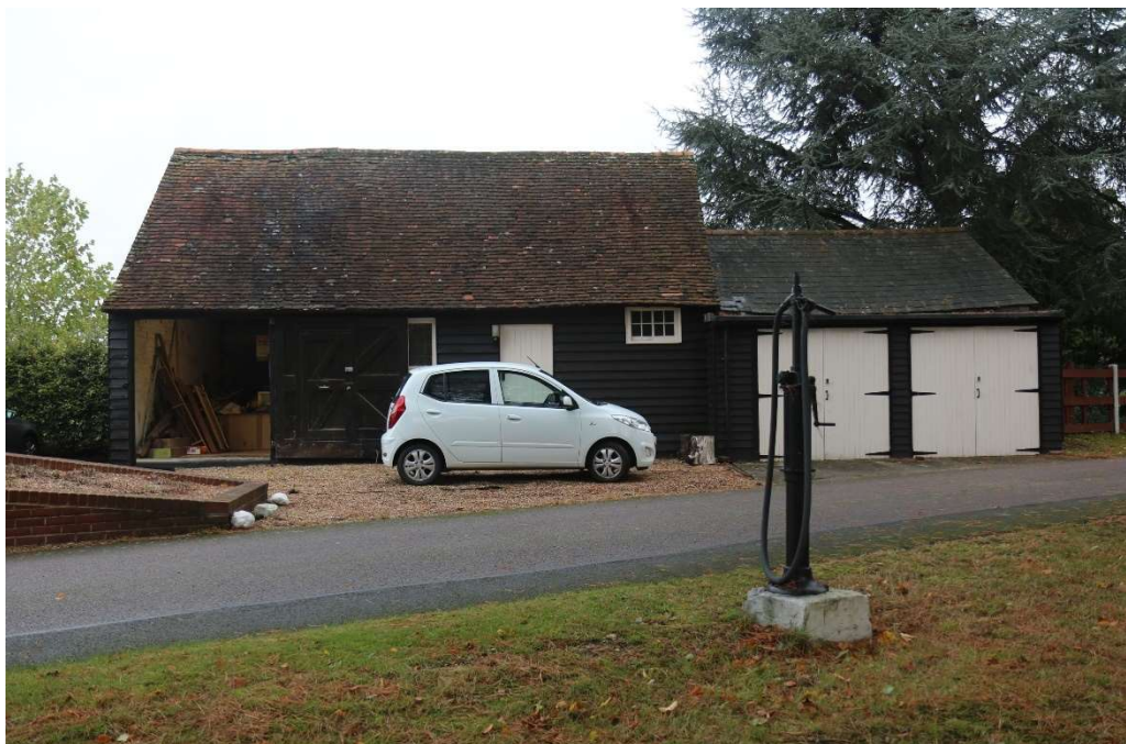
Photograph 1 South-western elevation. Photograph taken facing north north-east.
