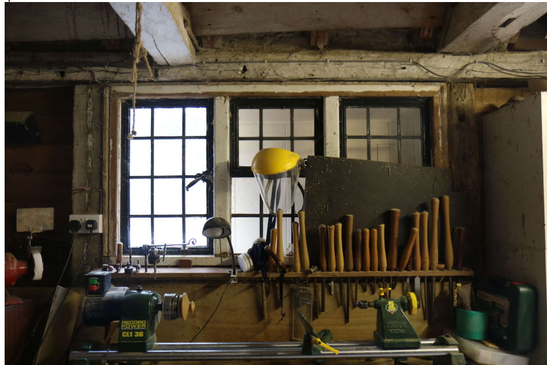
EEX60095_PhotoGraph_026 Detail of window in south-western wall of coach house. Photograph taken facing south south-west.
