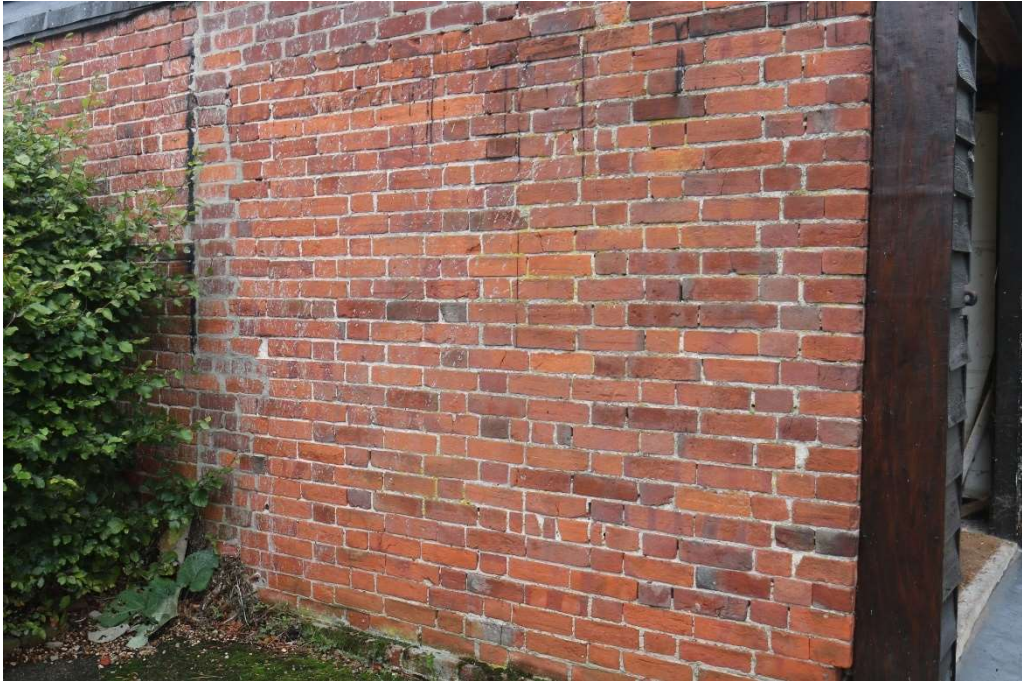
Photograph 4 Detail of brickwork on north-western elevation. Photograph taken facing east.
