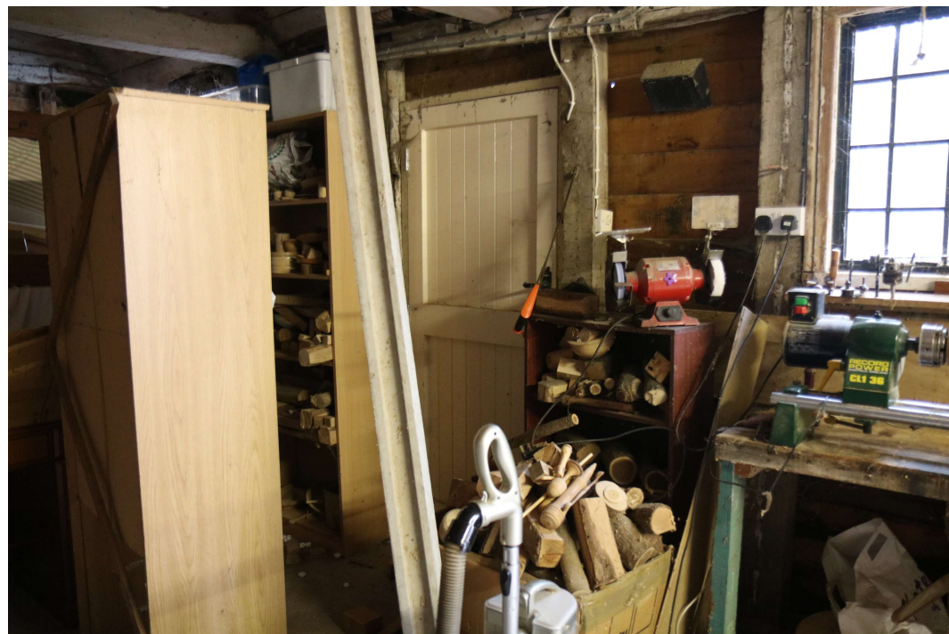
EEX60095_PhotoGraph_028 Detail of door in south-western wall of coach house. Photograph taken facing south-east.
