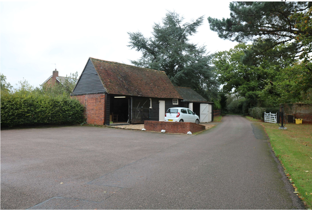
EEX60095_PhotoGraph_041 Location shot of building. Photograph taken facing north-east.
