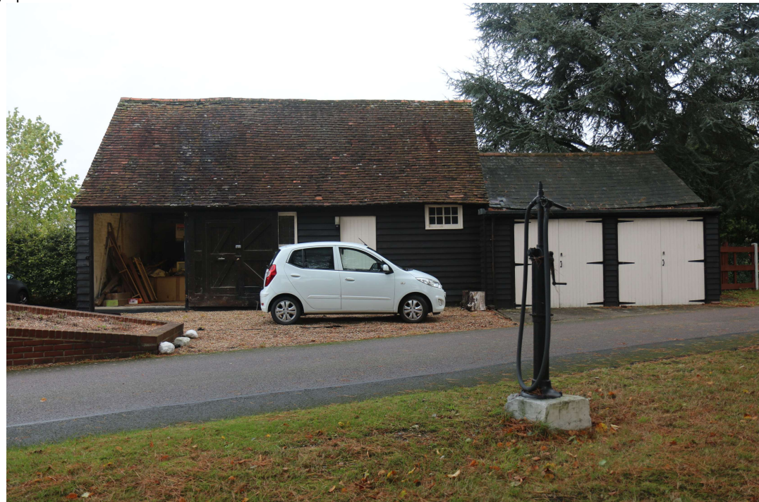
EEX60095_PhotoGraph_002 South-western elevation. Photograph taken facing north north-east.
