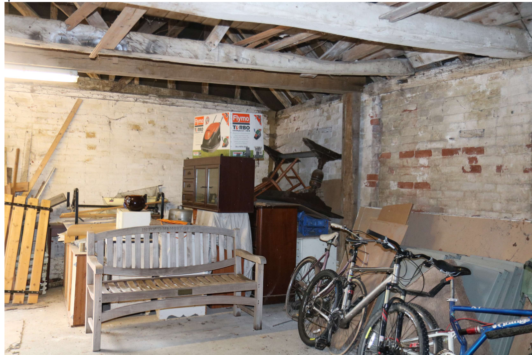
EEX60095_PhotoGraph_014 Interior of coach house. Photograph taken facing north-west.
