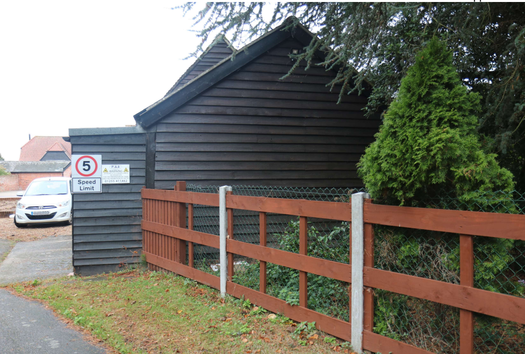
EEX60095_PhotoGraph_001 South-eastern elevation. Photograph taken facing west north-west.
