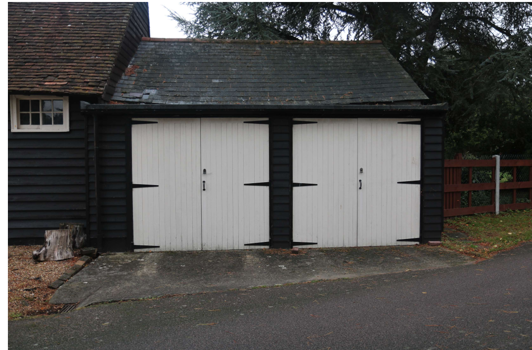
EEX60095_PhotoGraph_004 South-western elevation of garage. Photograph taken facing north north-west.
