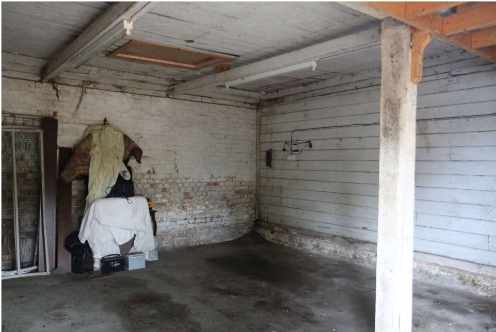
Photograph 12 Interior of garage. Photograph taken facing north-east.
