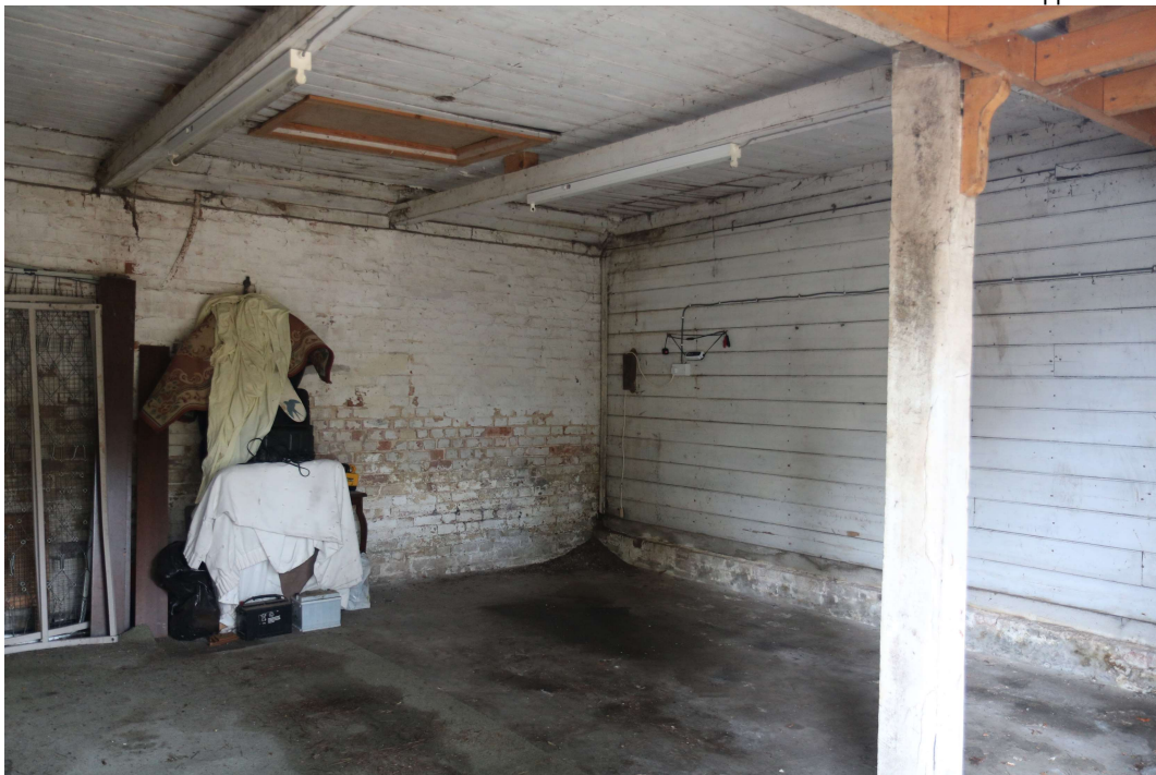
EEX60095_PhotoGraph_033 Interior of garage. Photograph taken facing north-east.
