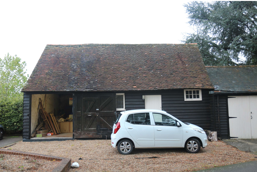
EEX60095_PhotoGraph_003 South-western elevation of coach house. Photograph taken facing north north-east.
