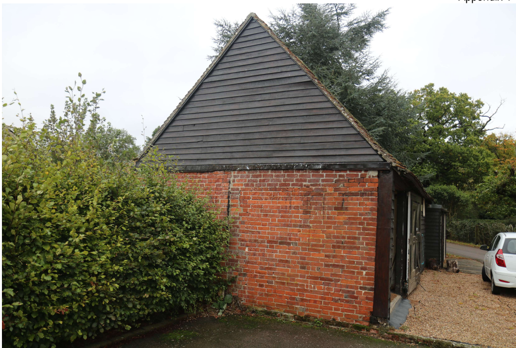
EEX60095_PhotoGraph_009 North-western elevation. Photograph taken facing east.
