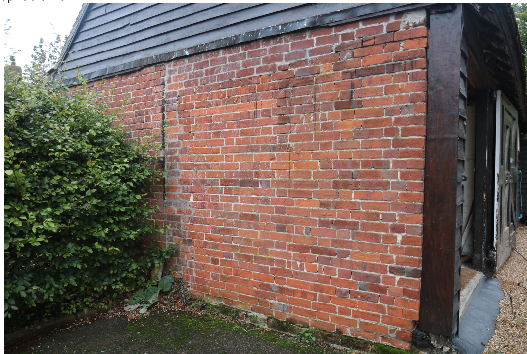
EEX60095_PhotoGraph_010 Detail of bricks of north-western elevation. Photograph taken facing east.
