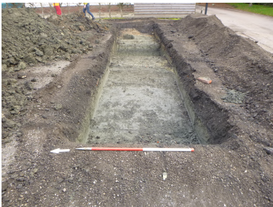
Photograph 6 Trench 12, looking east.
