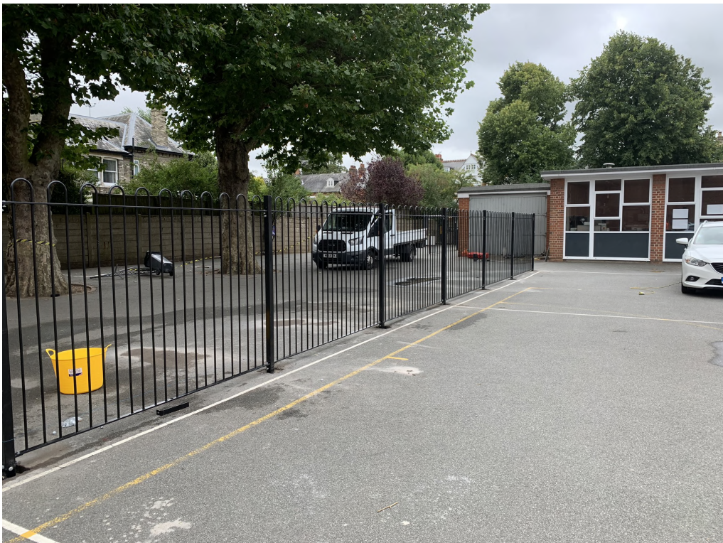
Photograph 6 Section 2 completed, looking south-east.
