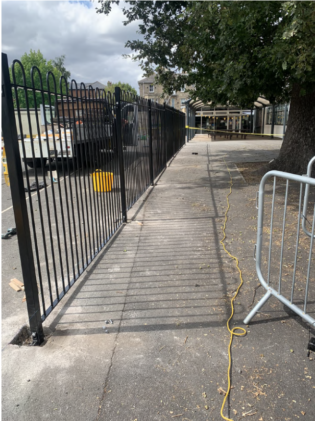
Photograph 3 Section 1 complete, looking north-west.
