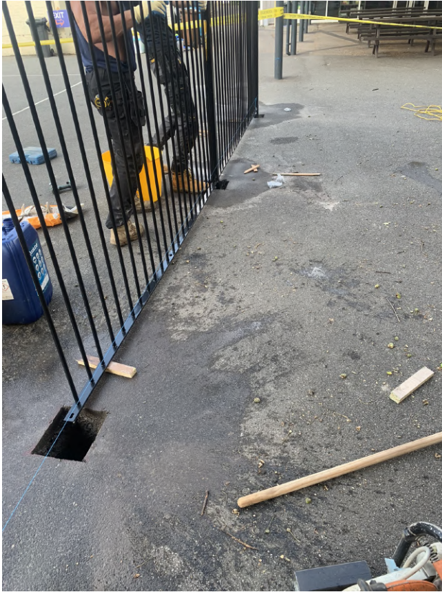
Photograph 1 Section 1 fencing, looking west.
