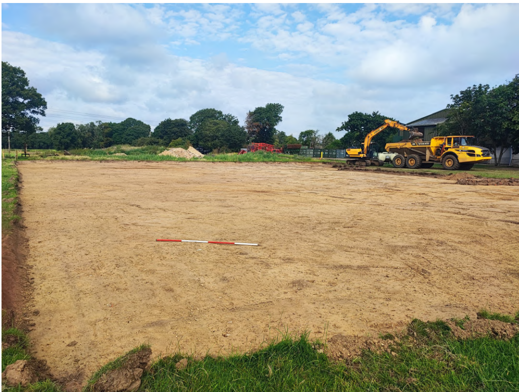
Photograph 1 General site shot, looking north-west.
