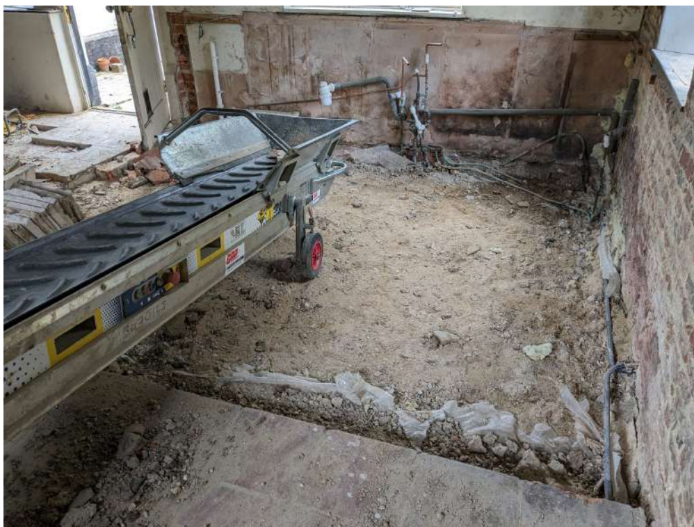
Photograph 5 Concrete removal in the kitchen, view east.
