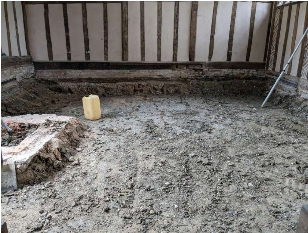
Photograph 1 Completed excavation the Great Hall, view east.
