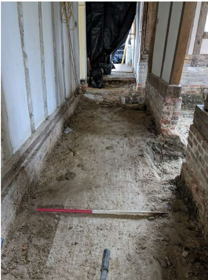
Photograph 4 Completed excavation in the passageway, view north.
