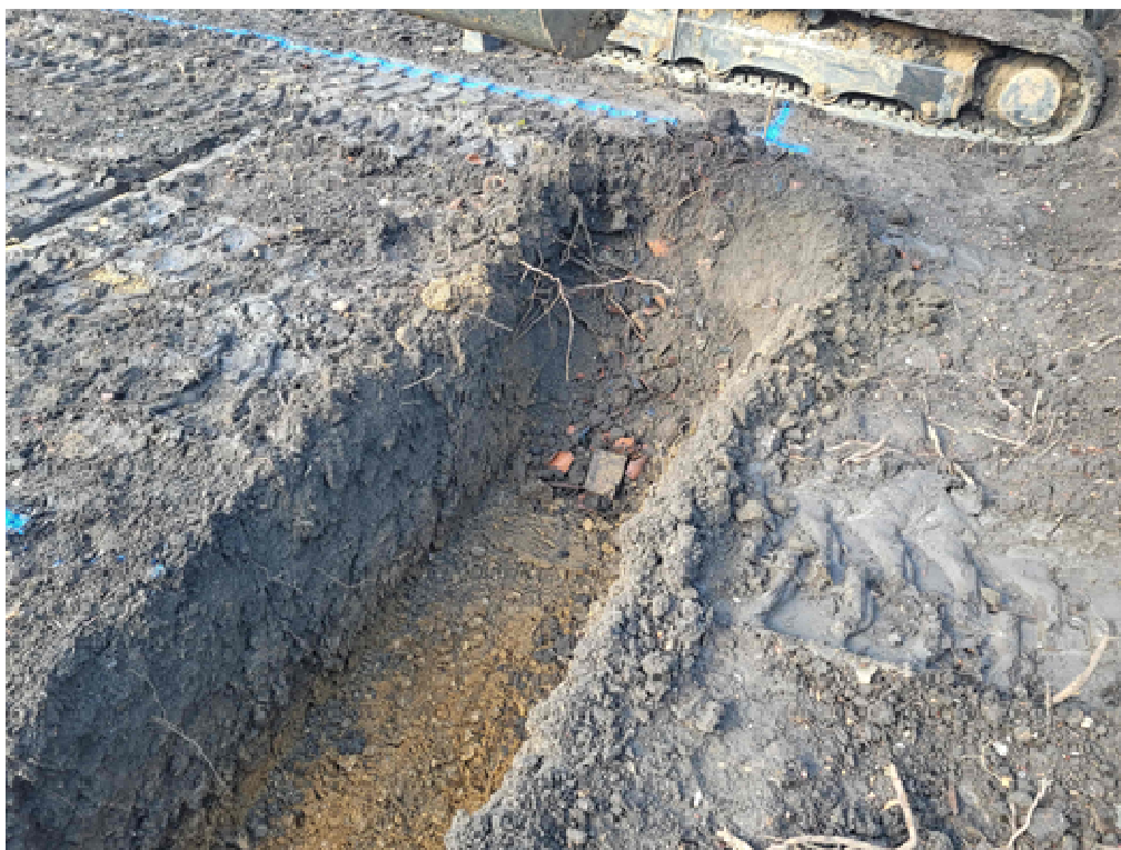
Photograph 1 Foundation trenches with F1, looking south-west
