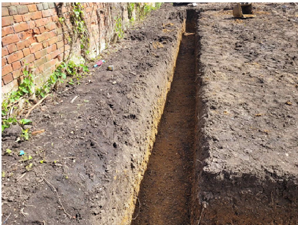
Photograph 2 Foundation trenches, looking south-east
