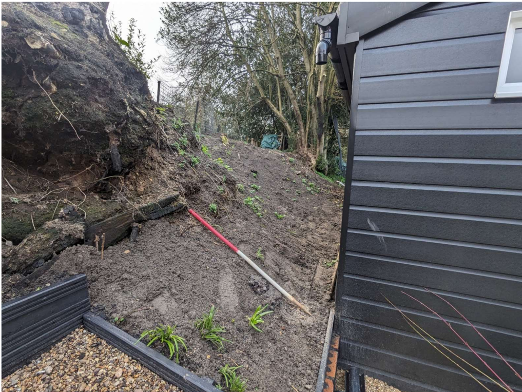
Photograph 7 Dyke after reconstruction, view south-east.
