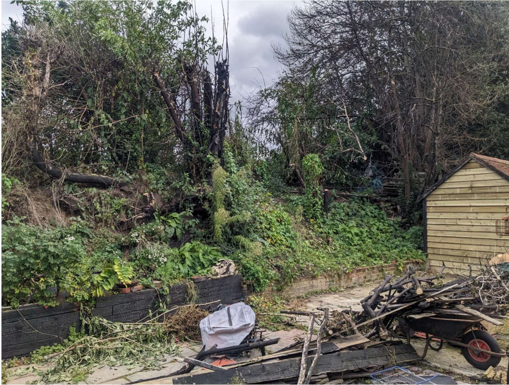
Photograph 4 Dyke after tree removal, view south-east.
