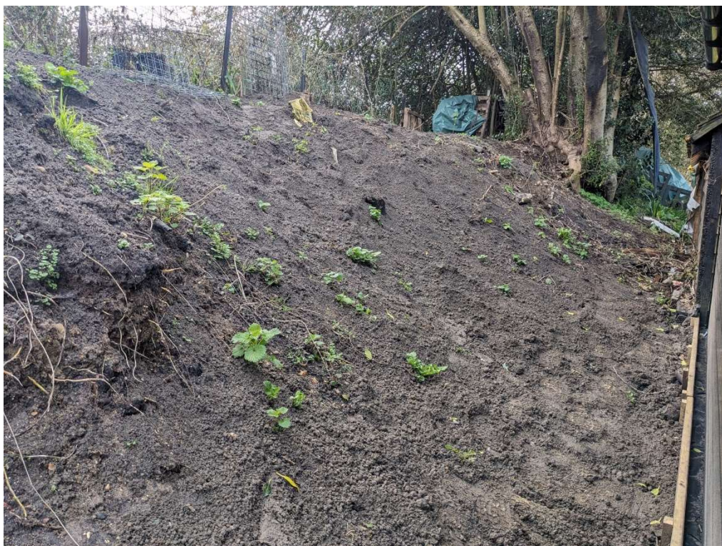
Photograph 8 Dyke after reconstruction, view south-east.
