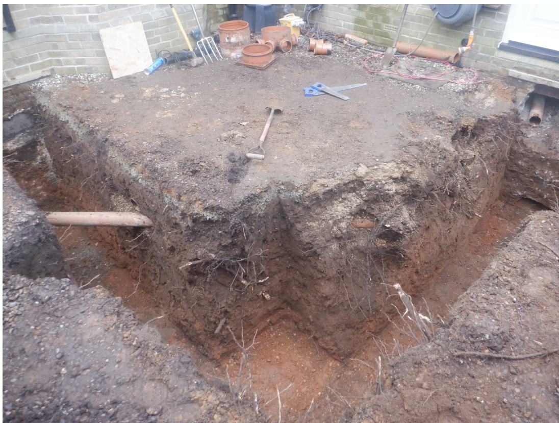
Photograph 2 Excavated foundation, view south east.
