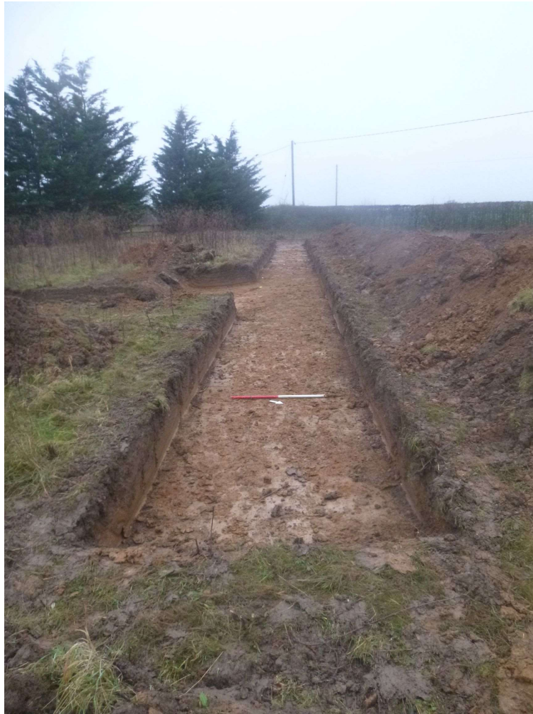
Photograph 1 T3 trench shot – looking west
