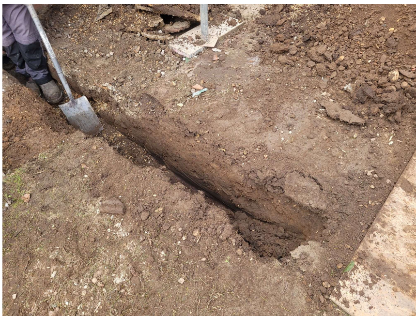
Photograph 3 Service trench – looking north
