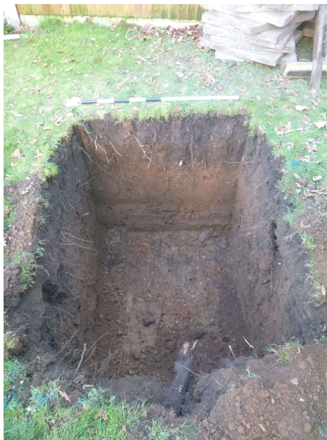
Photograph 4 Soakaway – looking south-east.
