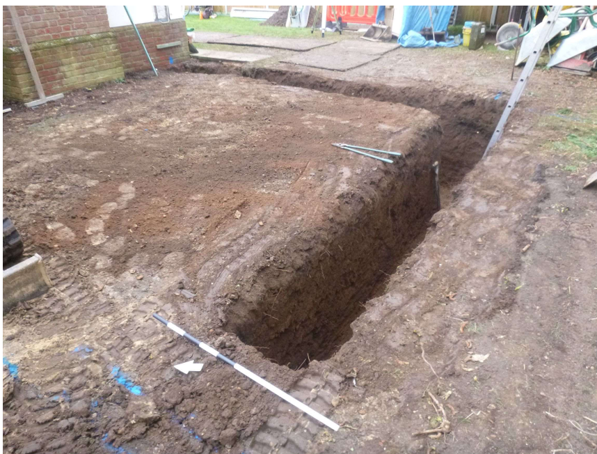
Photograph 2 Foundation trenching – looking north-east
