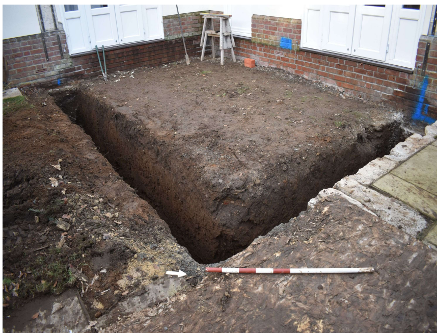
Photograph 1 Foundation trenching – looking west
