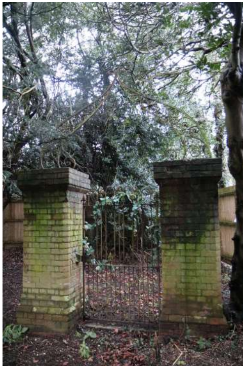
ECCP24 photograph_009Detail of gate. Photograph taken facing north-west.
