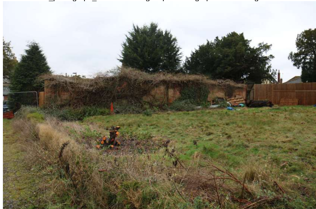
ECCP24_photograph_032Detail of wall. Photograph taken facing south south-west.
