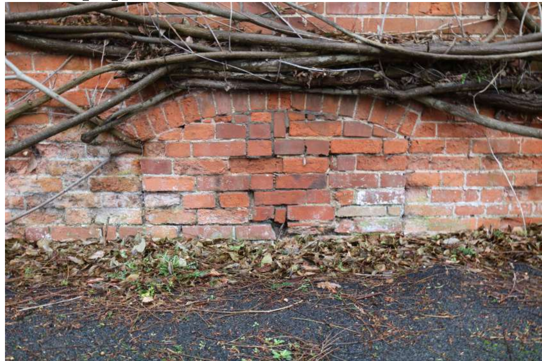
ECCP24_photograph_038Detail of bricked up arch in wall. Photograph taken facing north-w...
