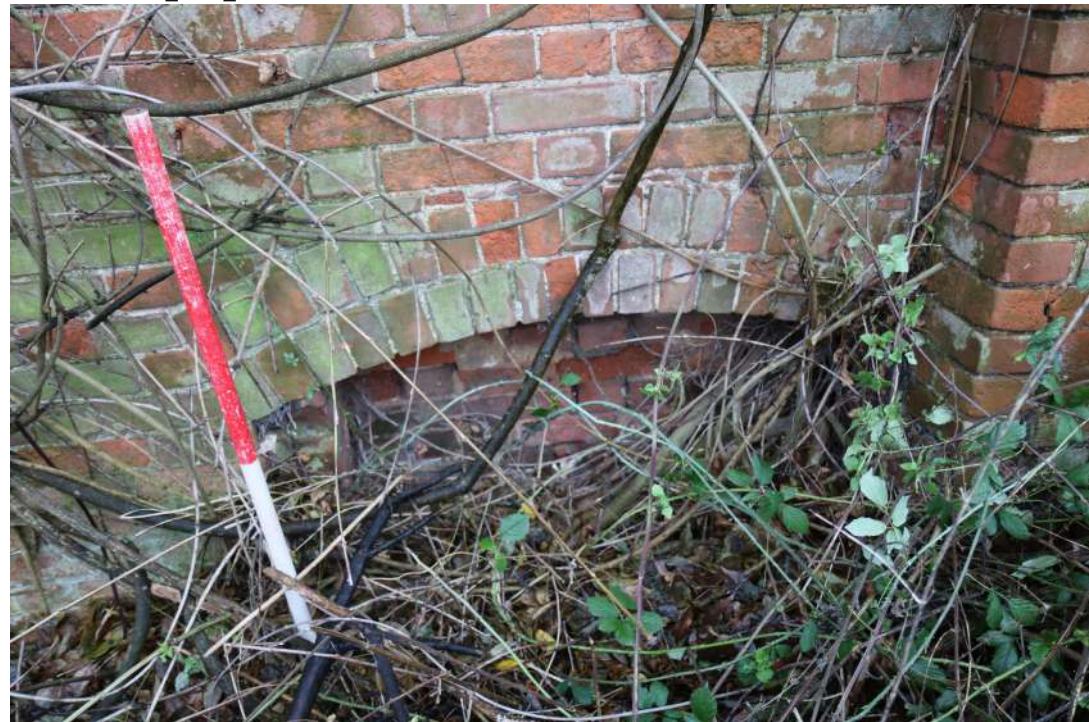
ECCP24_photograph_034Detail of arch in wall. Photograph taken facing south.
