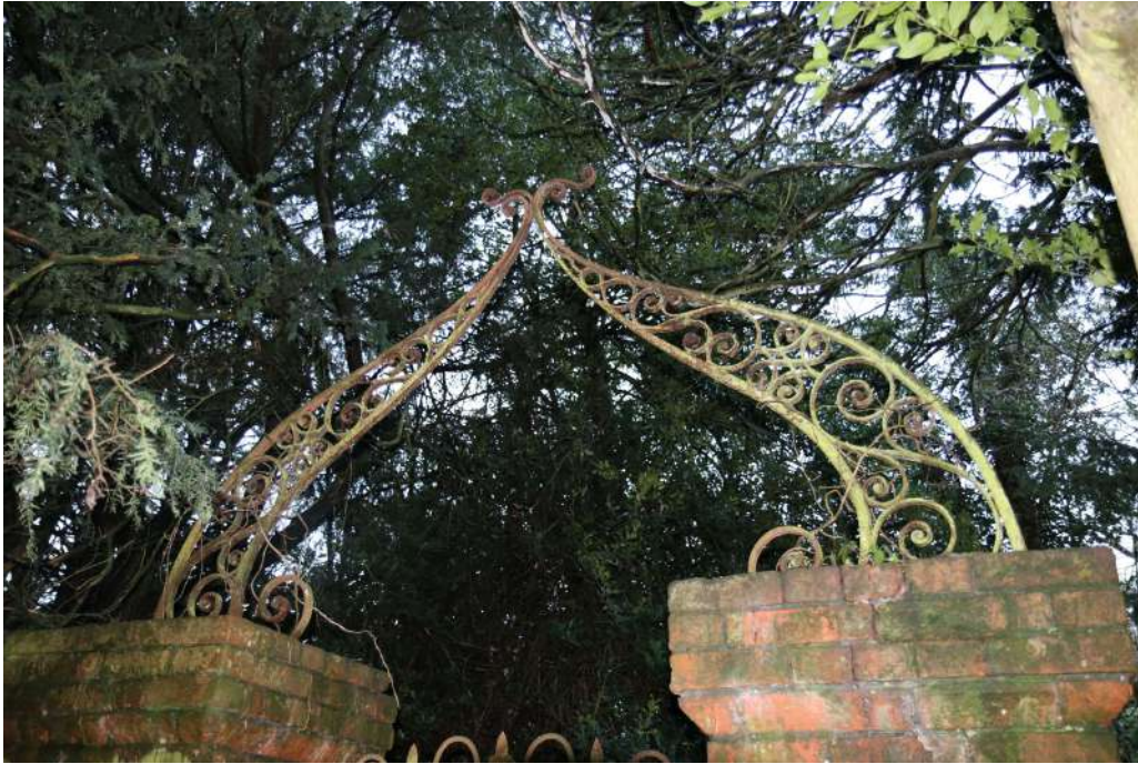
Photograph 7 Detail of iron arch above gate. Photograph taken facing north-west.
