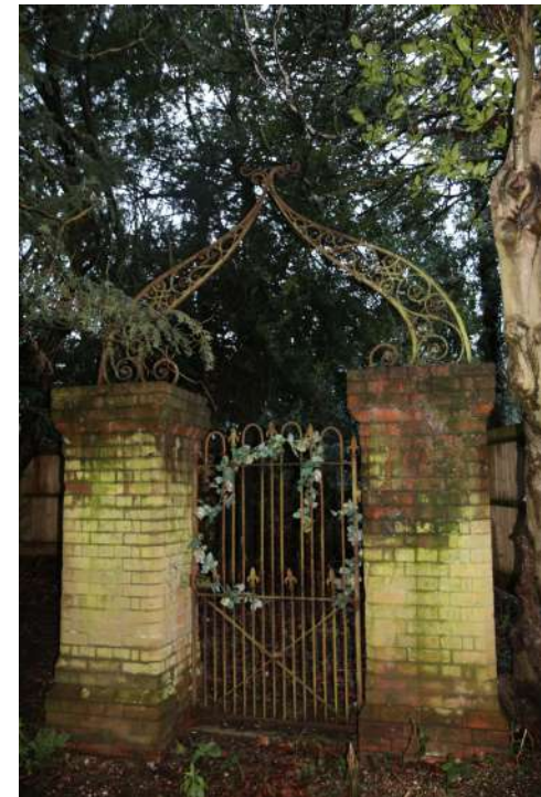
ECCP24 photograph_010Detail of gate. Photograph taken facing north-west.
