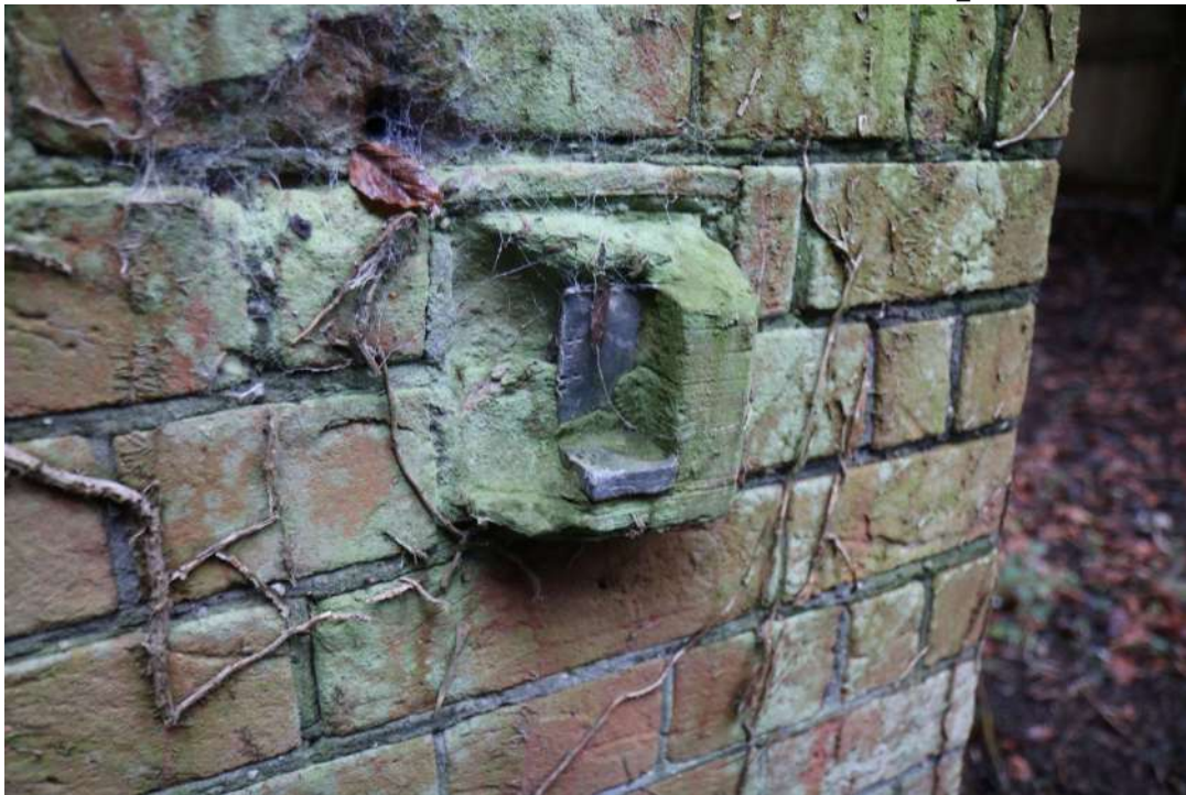
ECCP24_photograph_017Detail of gate lock. Photograph taken facing south-west.
