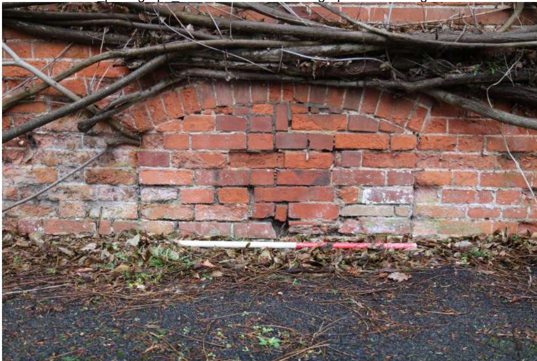
ECCP24_photograph_039Detail of bricked up arch in wall. Photograph taken facing north-w...
