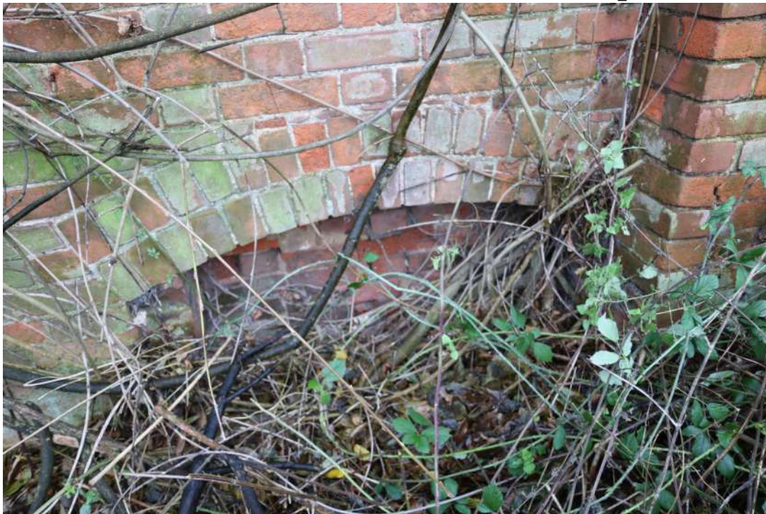
ECCP24_photograph_033Detail of arch in wall. Photograph taken facing south.
