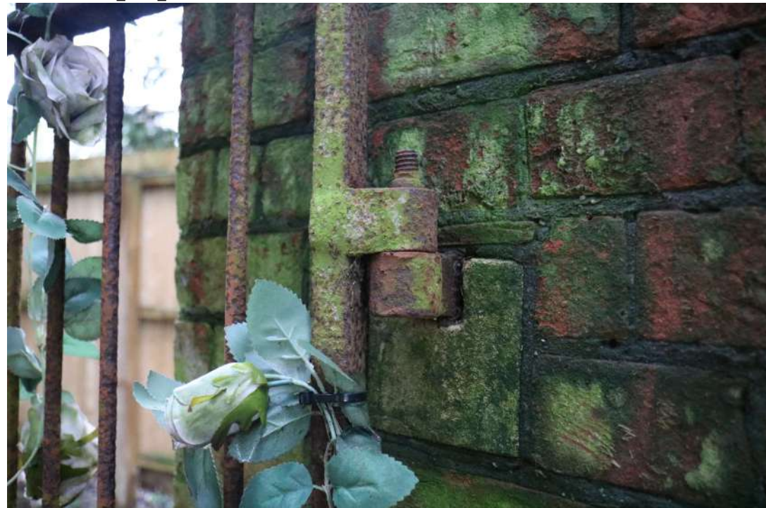
ECCP24_photograph_018Detail of gate hinge. Photograph taken facing north-east.
