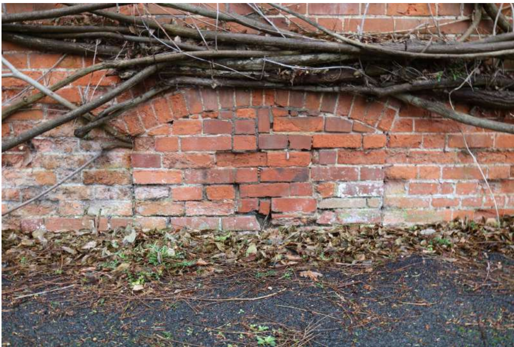
Photograph 10 Detail of bricked up arch in wall. Photograph taken facing north-west.
