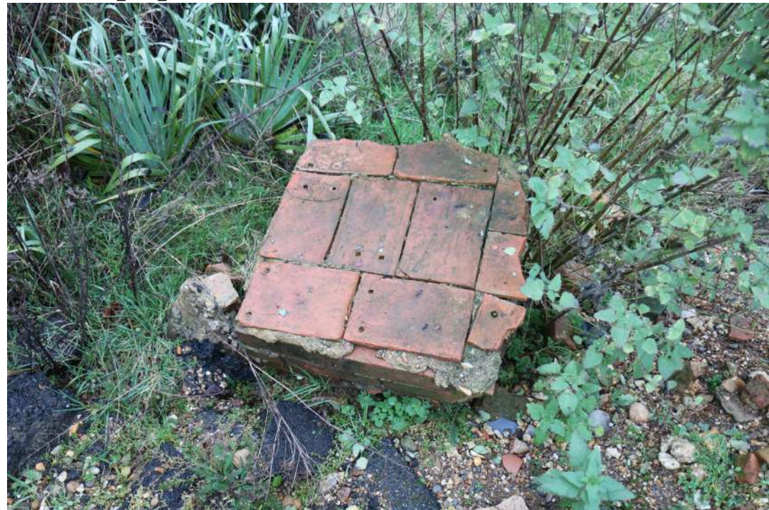
ECCP24_photograph_026Detail of demolished brickwork covered with geotextile.
