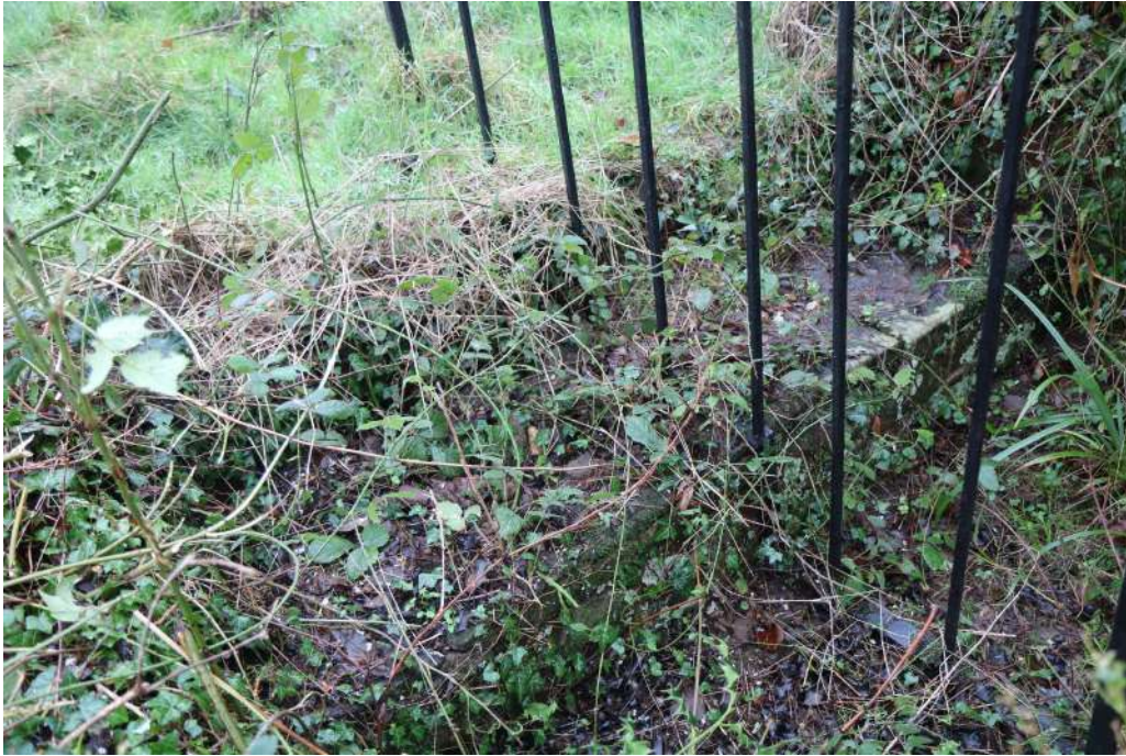
Photograph 5 Detail of small steps. Photograph taken facing south-west.
