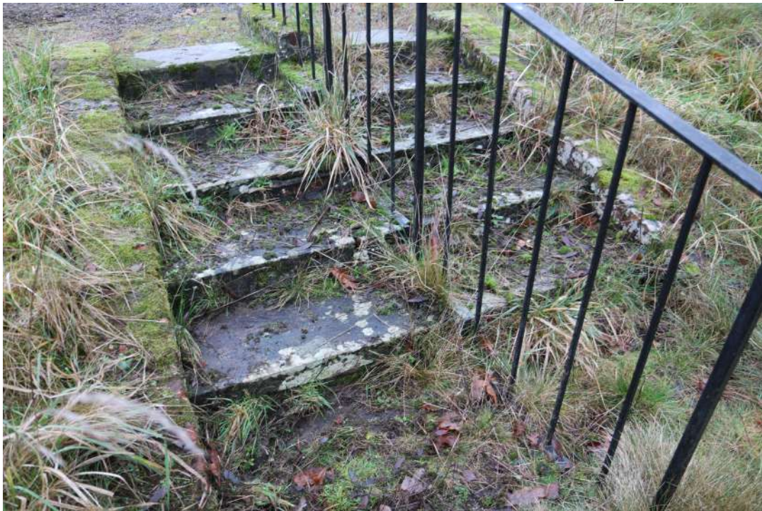
ECCP24_photograph_029Detail of big steps. Photograph taken facing west.
