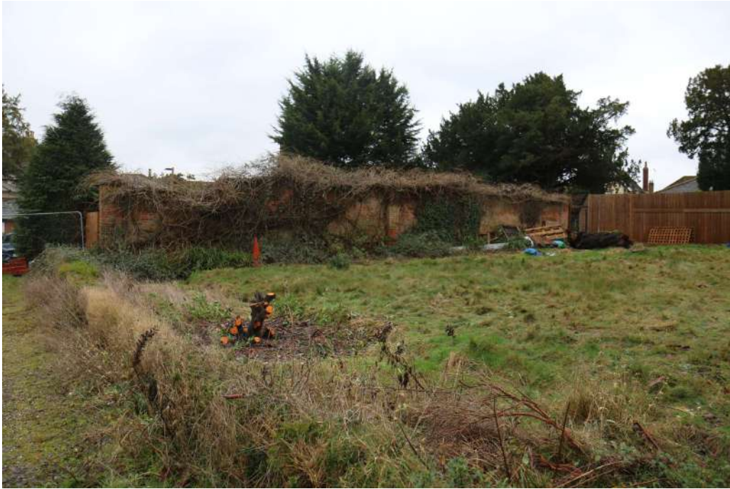
Photograph 9 Detail of wall. Photograph taken facing south south-west.
