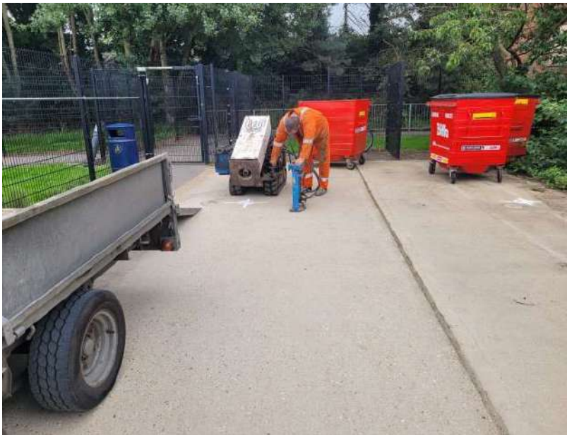
Photograph 1 Working shot of excavation of boreholes, view east.
