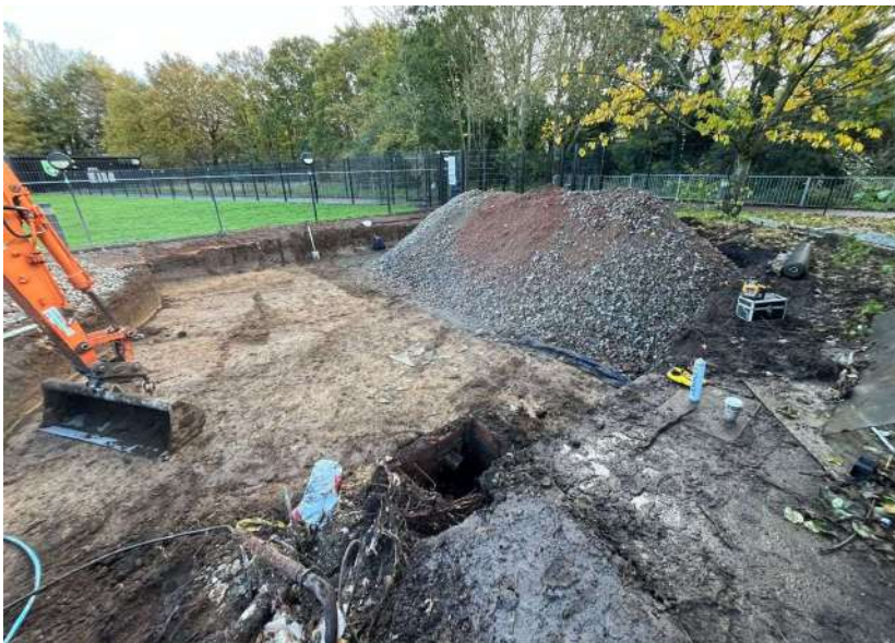
Photograph 3 Working shot of building footprint, view north-east.
