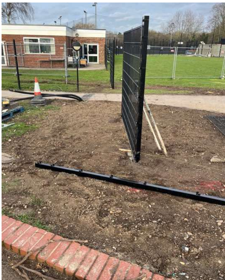
Photograph 18 Completed section of fencing, view north.
