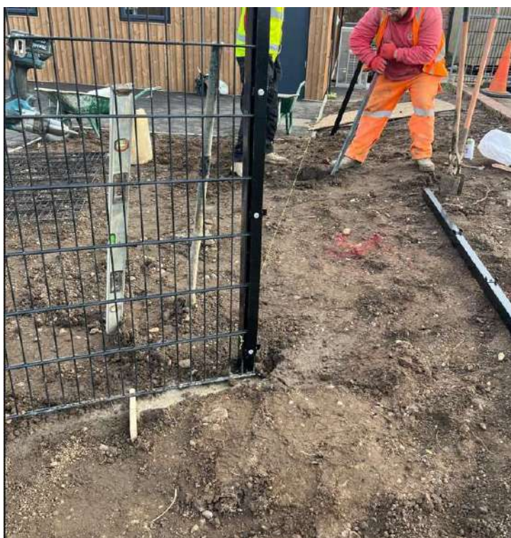
Photograph 19 Working shot of fence posts, view east.
