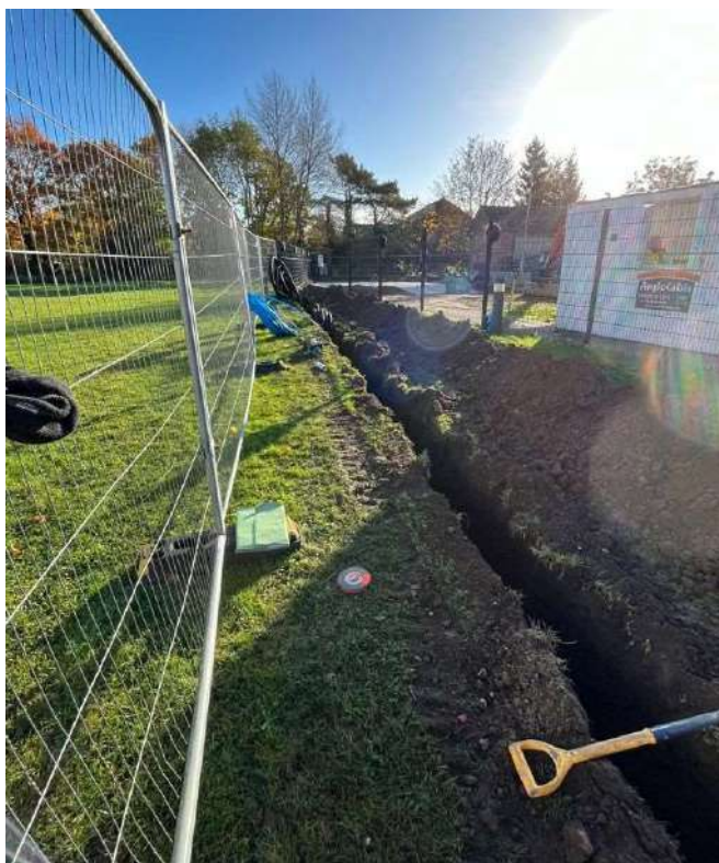
Photograph 8 Working shot of service trench looking towards footprint, view south-east.
