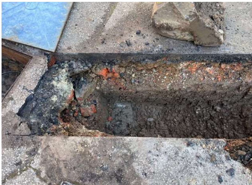
Photograph 11 General shot of L4 and L5, view north-east.
