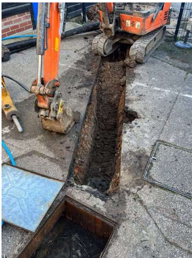
Photograph 10 Working shot of service trench at the west end, view south-east.
