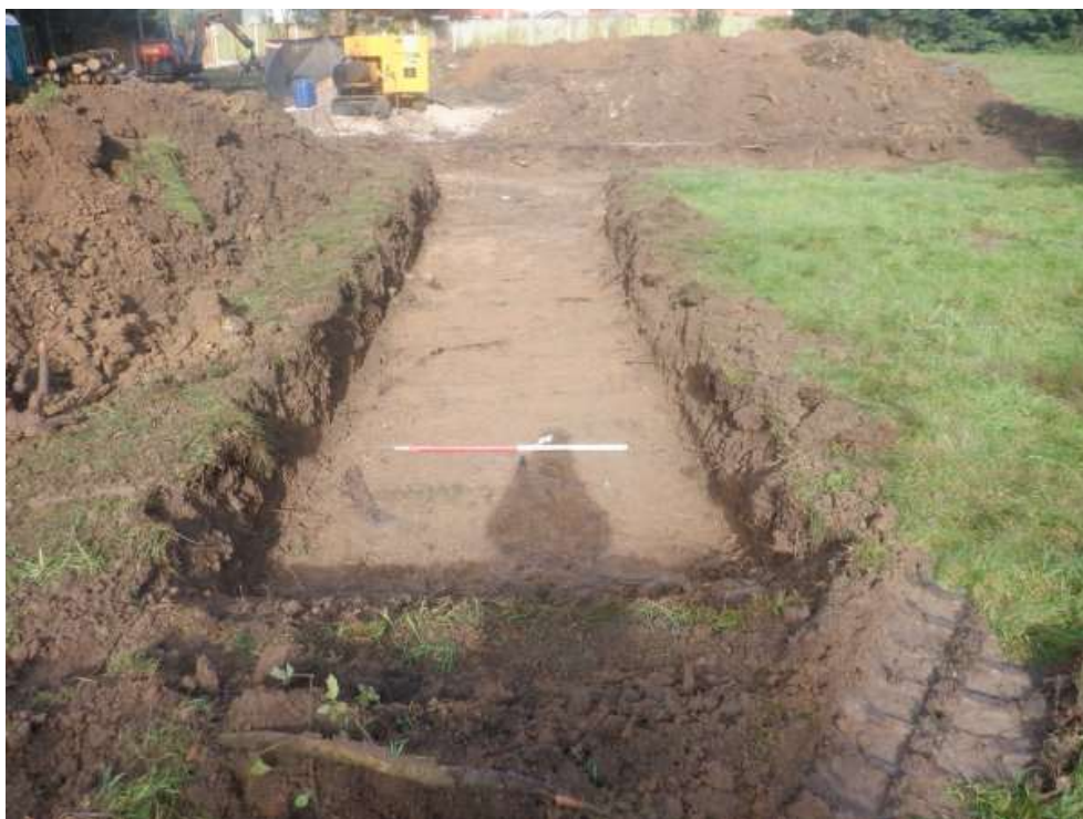
Photograph 9 T6, view north-west.
