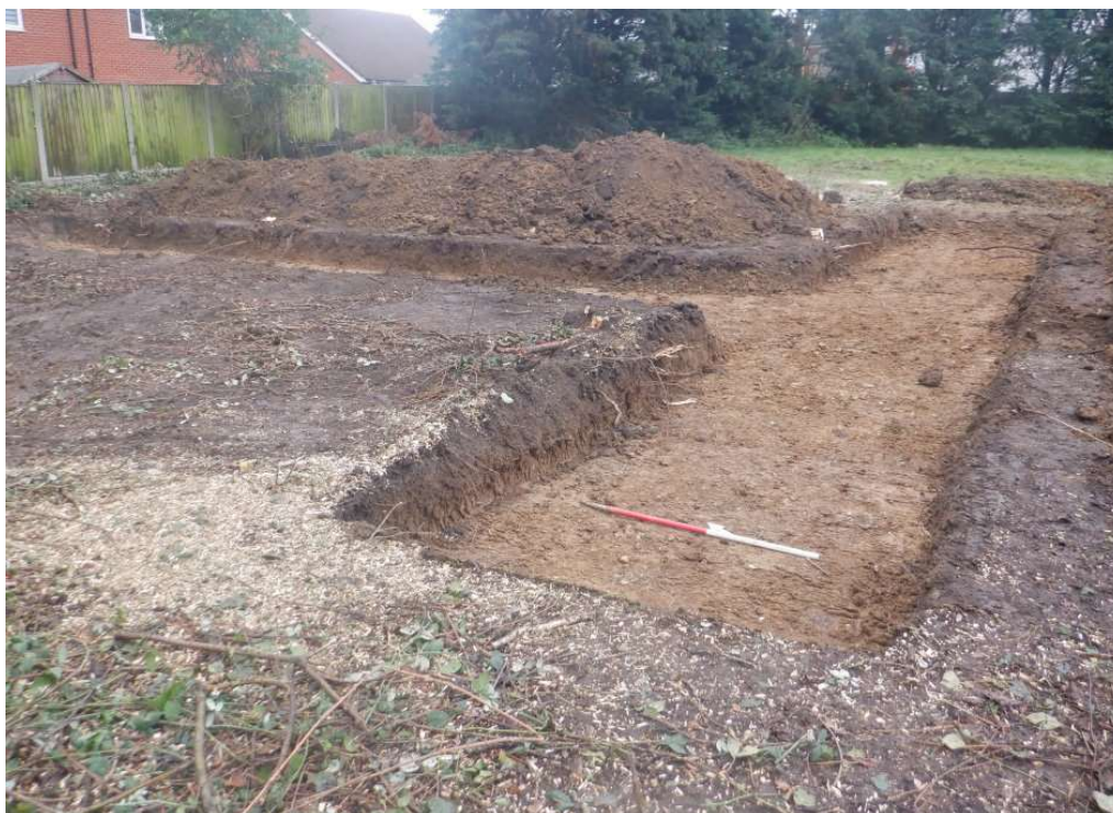
Photograph 2 T2, view north-east.
