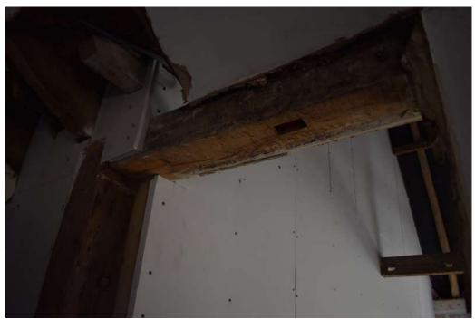
**Photograph 49** Detail of empty mortice in wall-plate in room 21. Photograph taken facing south-west.
