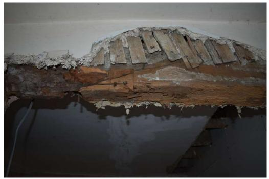
**Photograph 35** Detail of splayed scarf-joint in girding-beam in room 13. Photograph taken facing north-west.
