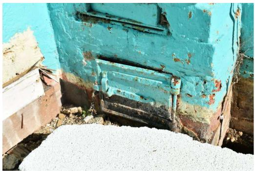
**Photograph 15** Detail of clean out door in south-west elevation. Photograph taken facing north.
