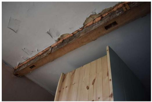
**Photograph 32** Detail of empty mortices in girding-beam above window in room 11. Photograph taken facing south-west.
