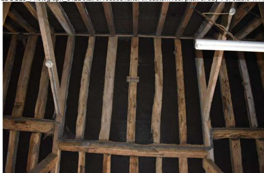
LBGG23\_Photograph\_043Detail of roof structure, showing reused timbers, of eastern roof p... LBGG23\_Photograph\_044Detail of roof structure, showing reused timbers, of eastern roof p... Page 11/18
