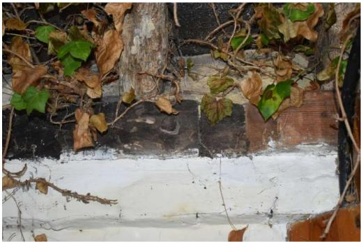
**Photograph 15** Detail of scarf-joint in eastern wall-plate in bay 3 of stable 1. Photograph taken facing east.
