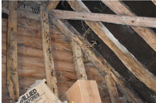
LBGG23\_Photograph\_037Detail of timber-frame showing reused wall-plate in northern wall ... LBGG23\_Photograph\_038Detail of reused principal rafter in northern wall of bay 1 of stable ...
