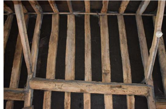
LBGG23\_Photograph\_049Detail of knee-brace between bays 3 and 4 of stable 1. Photograp...LBGG23\_Photograph\_050Detail of roof structure, showing reused timbers, of western roof p...
