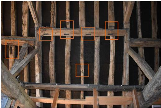
Photograph 17 Detail of roof structure of western roof pitch of bay 5 of stable 1. Evidence of reuse highlighted in orange. Photograph taken facing west.
