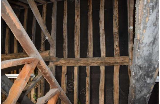
LBGG23\_Photograph\_051Detail of reused rafters in western roof pitch of bay 3 of stable 1. ... LBGG23\_Photograph\_052Detail of roof structure, showing reused timbers, of eastern roof p... Page 13/18
