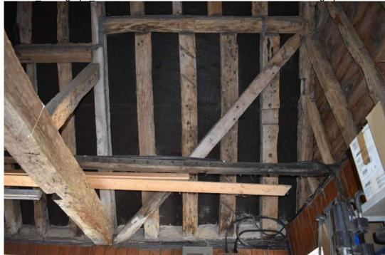
LBGG23\_Photograph\_035Detail of reused tie-beam in bay 1 of stable 1. Photograph taken f... LBGG23\_Photograph\_036Detail of roof structure showing reused rafters in western roof pitc...
