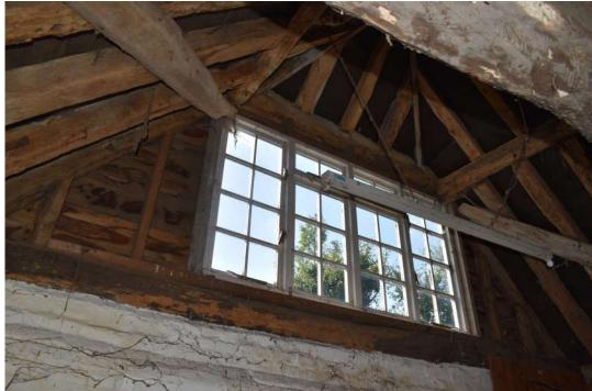
LBGG23\_Photograph\_061Detail of roof structure, showing reused timbers, of western roof p...LBGG23\_Photograph\_062Detail of window in south wall of bay 6 of stable 1. Photograph tak...
