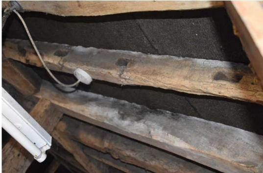
LBGG23\_Photograph\_045Detail of reused tie-beam with iron strap, between bays 2 and 3 o... LBGG23\_Photograph\_046Detail of reused rafter in western roof pitch of bay 2 of stable 1. P...
