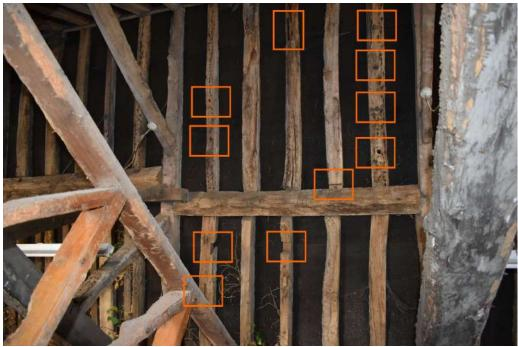
**Photograph 16** Detail of roof structure of eastern roof pitch of bay 4 of stable 1. Evidence of reused highlighted in orange. Photograph taken facing north-east.
