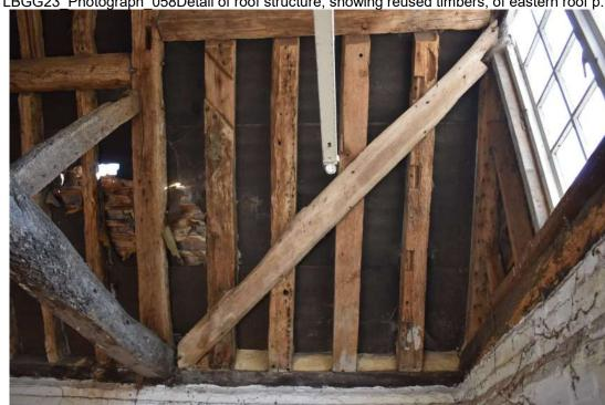
LBGG23\_Photograph\_059Detail of roof structure, showing reused timbers, of western roof p...LBGG23\_Photograph\_060Detail of roof structure, showing reused timbers, of eastern roof p...Page 15/18
