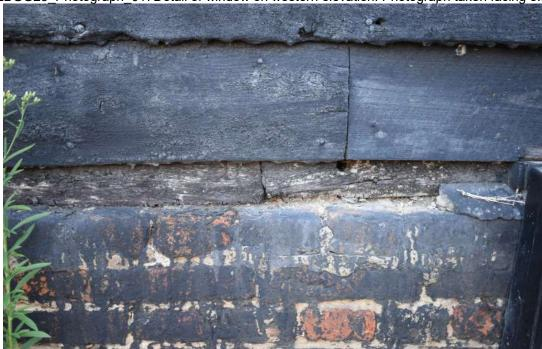
LBGG23 Photograph 019Detail of ?scarf-joint in western sill-beam. Photograph taken facin...
