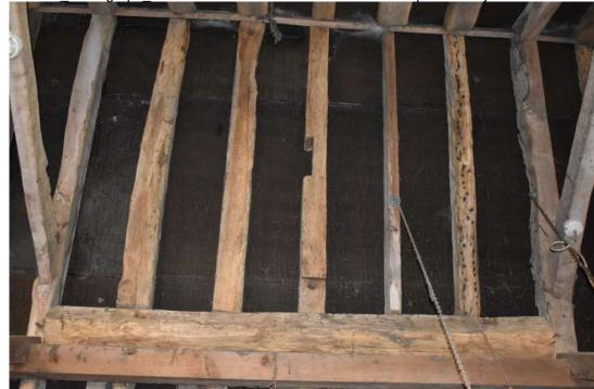
LBGG23\_Photograph\_047Detail of scarf-joint in eastern wall-plate in bay 3 of stable 1. Phot... LBGG23\_Photograph\_048Detail of roof structure, showing reused timbers, of eastern roof p...
