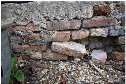
**Photograph 2** Detail of brick plinth on northern elevation. Photograph taken facing south.
