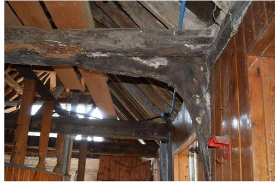
LBGG23\_Photograph\_053Detail of roof structure, showing reused timbers, of western roof p...LBGG23\_Photograph\_054Detail of knee-brace between bays 4 and 5 of stable 1. Photograp...
