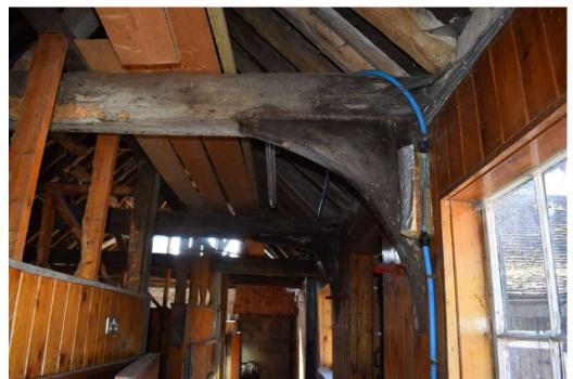
**Photograph 13** Detail of knee-brace between bays 3 and 4 of stable 1. Photograph taken facing south.
