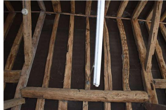
LBGG23\_Photograph\_057Detail of reused tie-beam between bays 4 and 5 of stable 1. Phot... LBGG23\_Photograph\_058Detail of roof structure, showing reused timbers, of eastern roof p...
