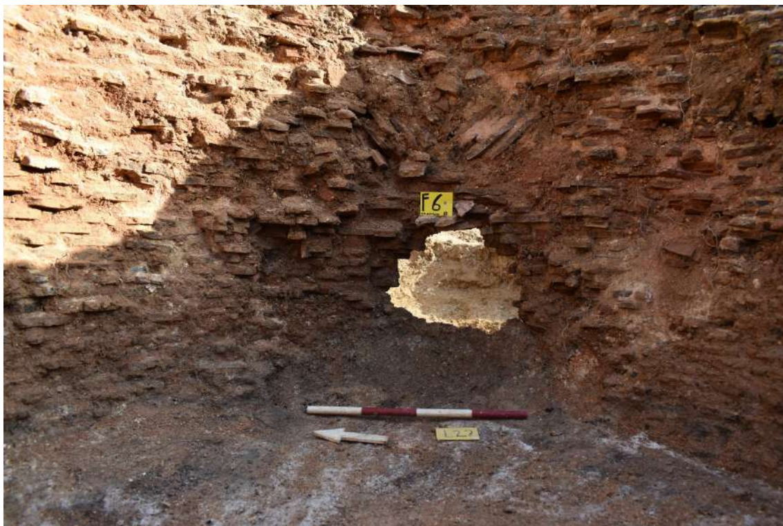
Photograph 10 Draw-hole between Chambers A and B of lime kiln F6, looking east from Chamber B into A.
