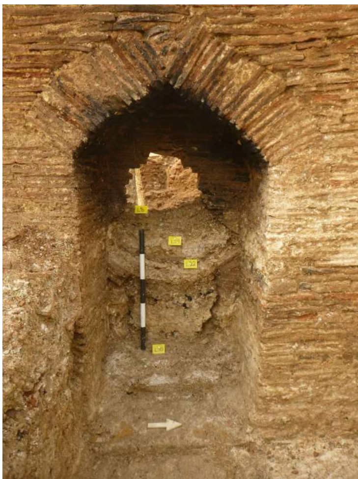
Photograph 9 Draw-hole between Chambers A and B of lime kiln F6, looking west from Chamber A into B.
