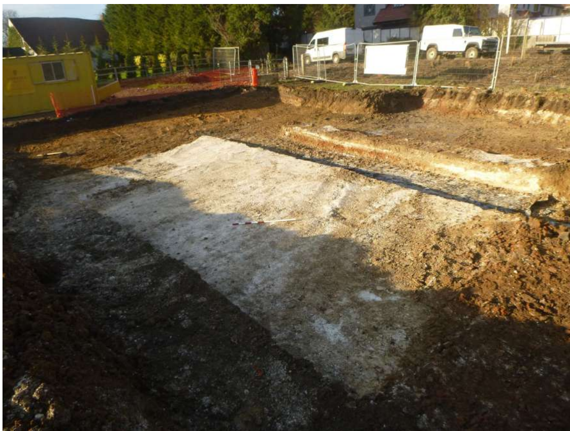
Photograph 14 Lime layer L7, looking north-west.
