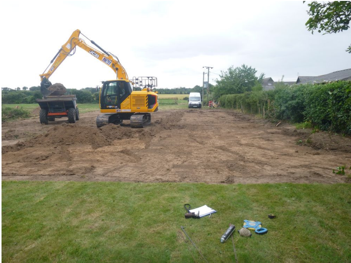
Photograph 1 Area strip/level reduction, view south.
