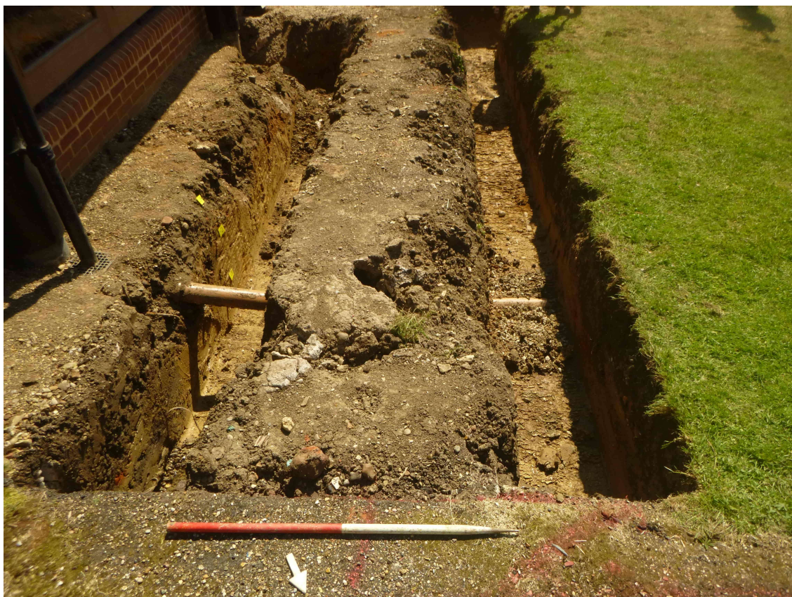
Photograph 2 Foundation trench, looking south-west.
