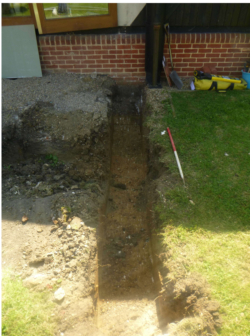
Photograph 1 Foundation trench, looking south-east.
