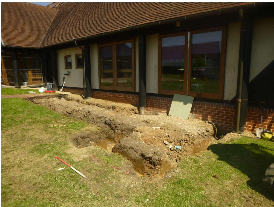
Photograph 3 General shot of completed works, looking east-south-east.
