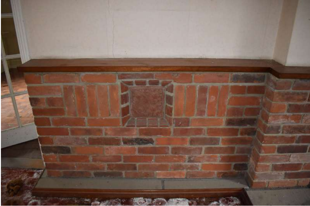
Photograph 13 Detail of decorative tile in lounge. Photograph taken facing south-east.
