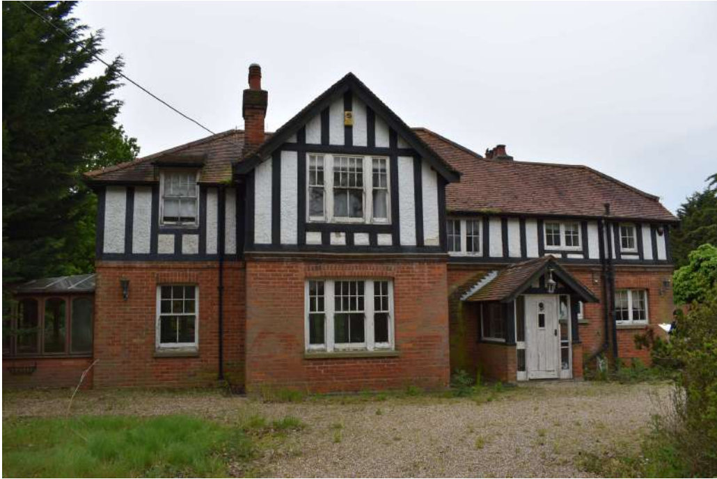
Photograph 2 Northern elevation. Photograph taken facing south-west.
