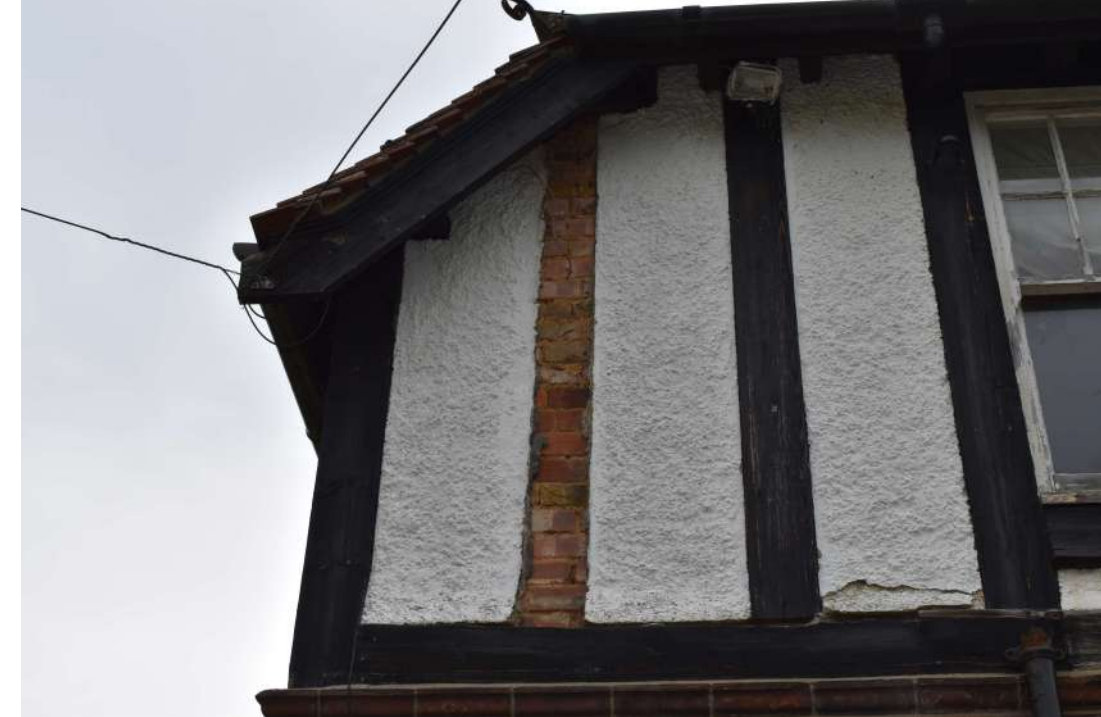
SAWO23a_PhotoGraph_023Detail of missing timber and brickwork beneath on western elevation. Ph...
