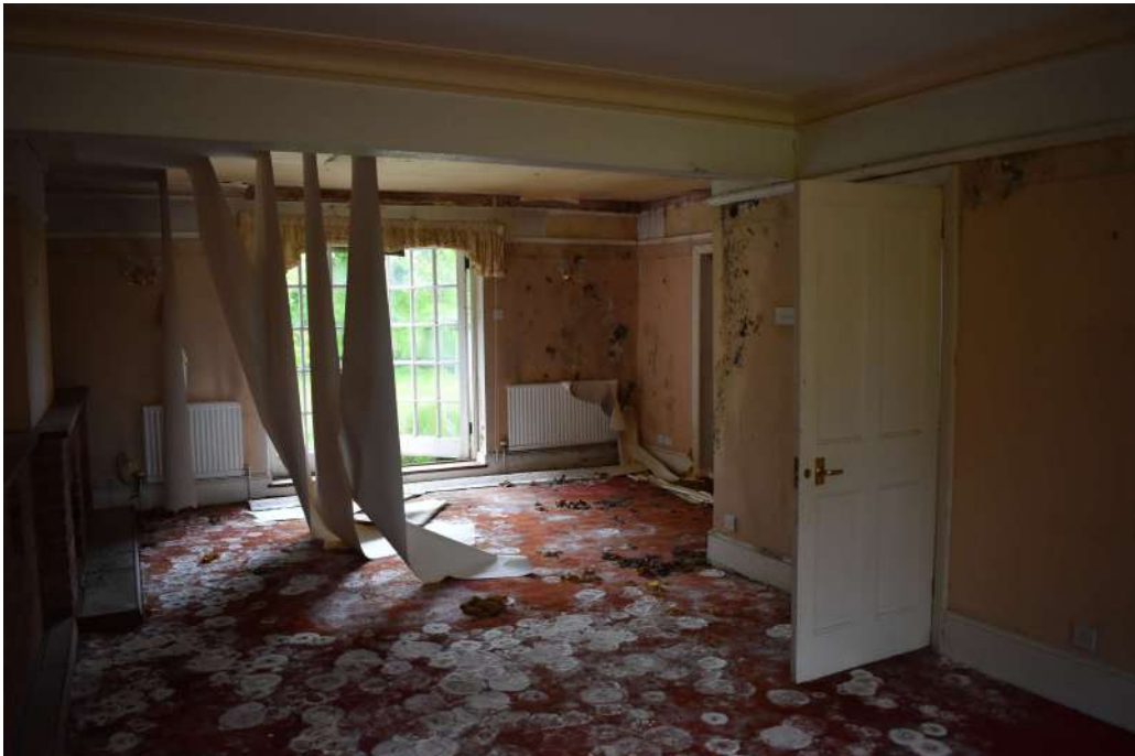
Photograph 11 Interior of lounge. Photograph taken facing south-west.
