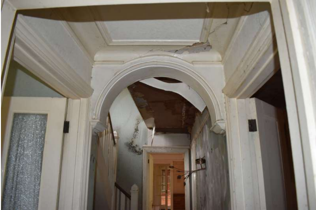
Photograph 15 Detail of timber arch in hall. Photograph taken facing east south-east.
