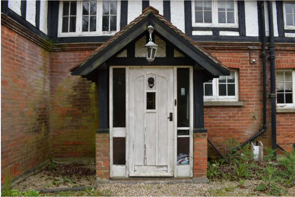
Photograph 4 Detail of porch of northern elevation. Photograph taken facing south south-west.
