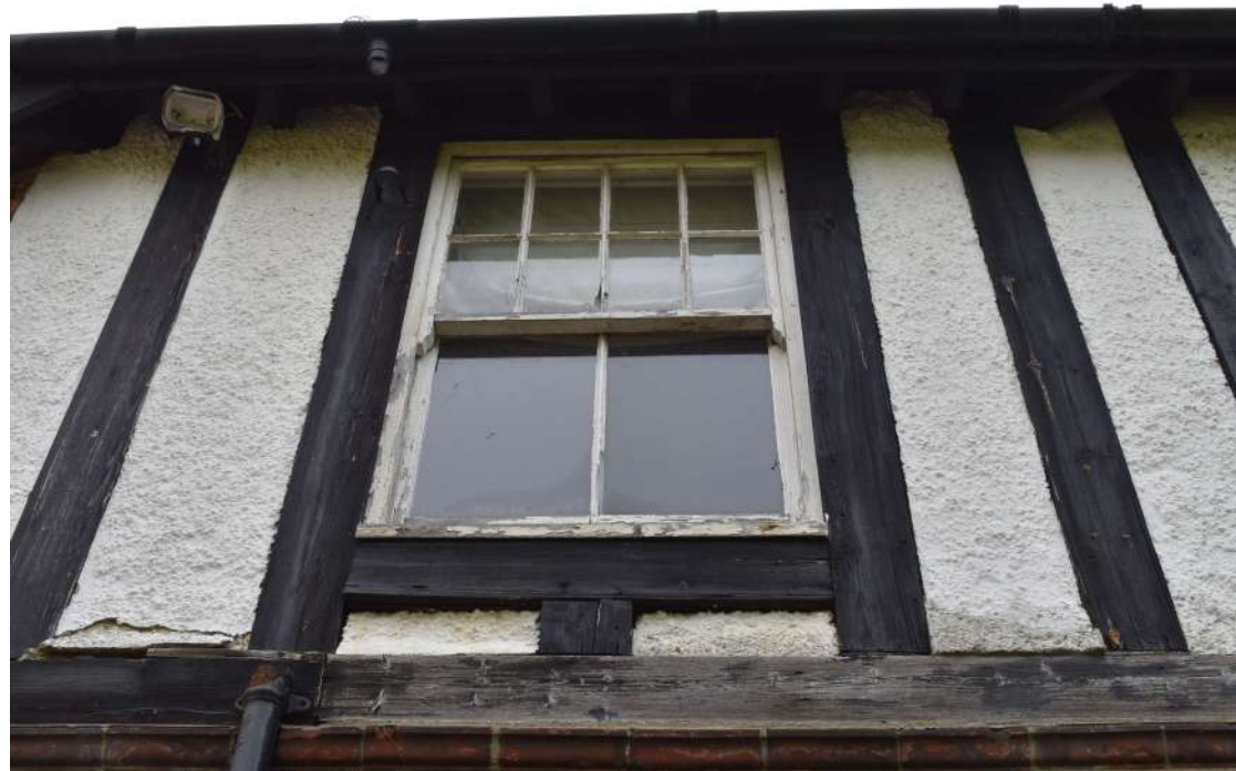
SAWO23a_PhotoGraph_023Detail of missing timber and brickwork beneath on western elevation. Ph...
