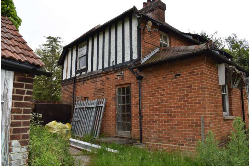
Photograph 10 Western elevation. Photograph taken facing north-east.
