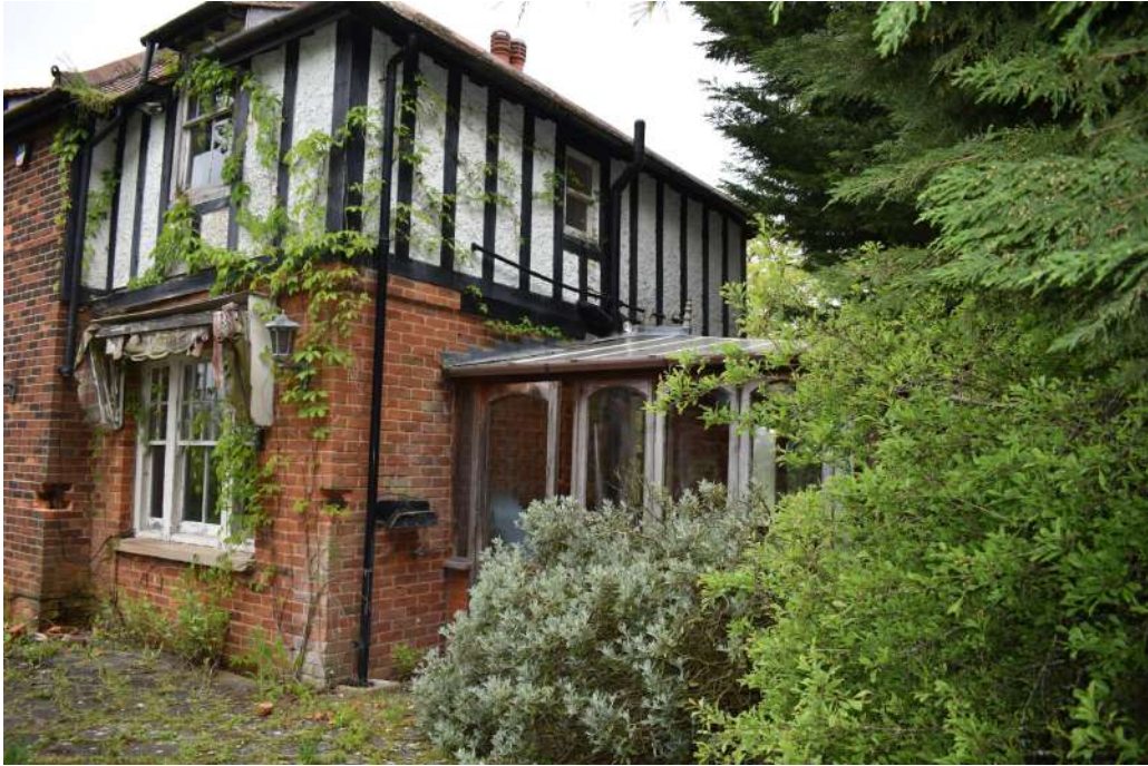
Photograph 7 Eastern elevation. Photograph taken facing north.
