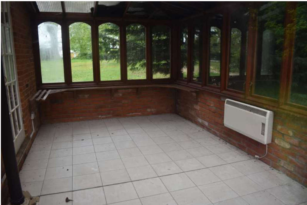
Photograph 18 Interior of conservatory. Photograph taken facing north north-east.
