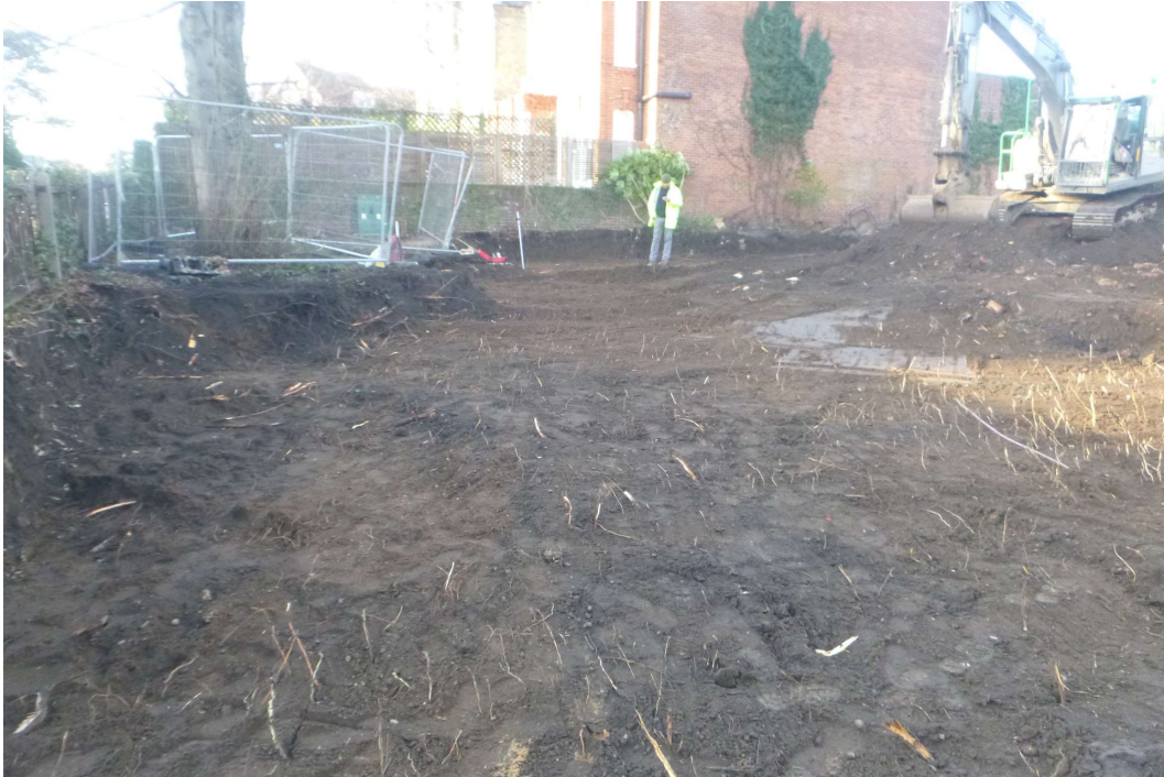
Photograph 5 Ground reduction of the driveway into L2, looking west.
