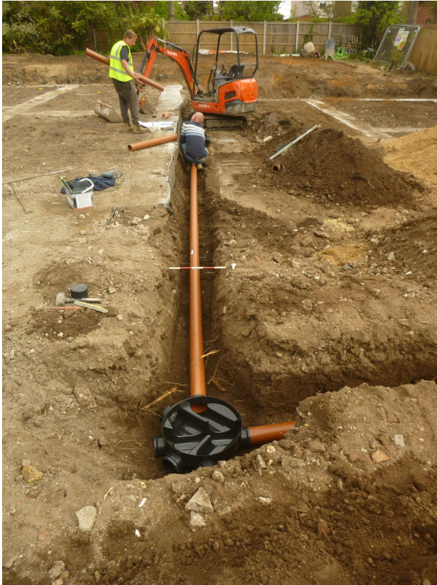
Photograph 7 Service trenches, looking north.
