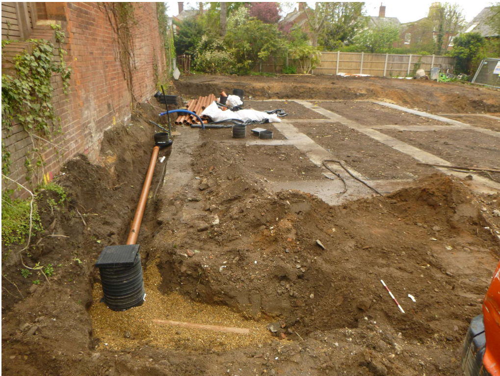
Photograph 8 Service trenches, looking north.
