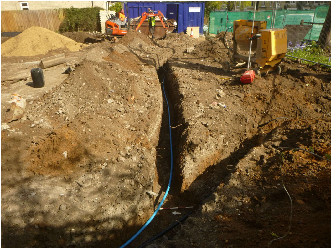
Photograph 6 Service trenches, looking east.
