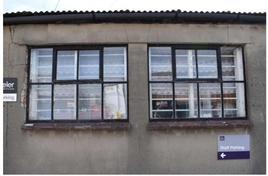
Photograph 4 Detail of Crittall windows on south-west elevation of outbuilding 2. Photograph taken facing north-east.
