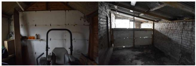
GEAGE23\_Photograph\_051.JPG Detail of interior wall cladding in sectional timber hut. Photograph taken facing north-west.
