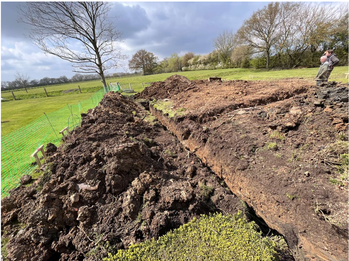
Photograph 2 Foundation trench, looking north-west.
