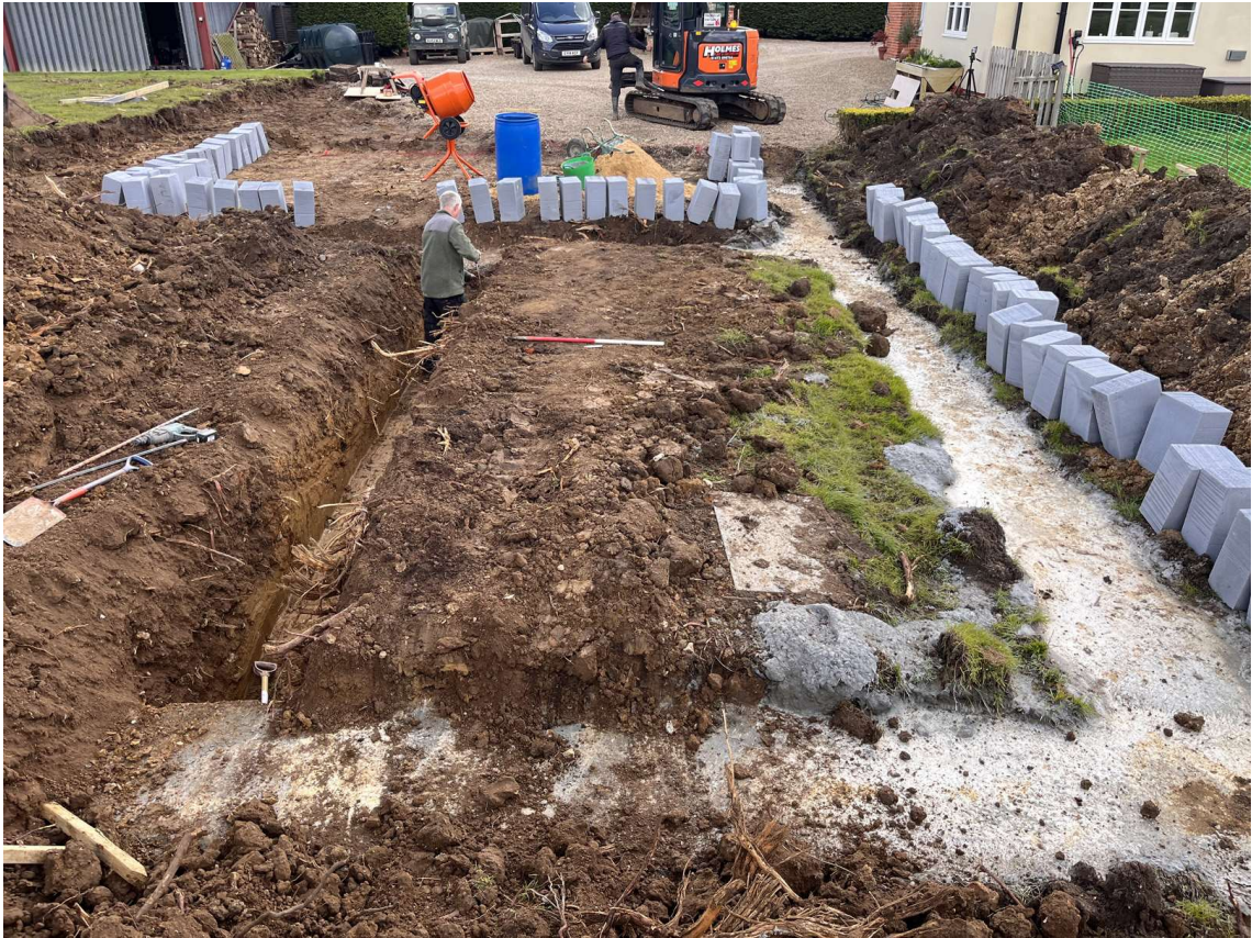
Photograph 3 Foundation trench, some concreted, looking east.
