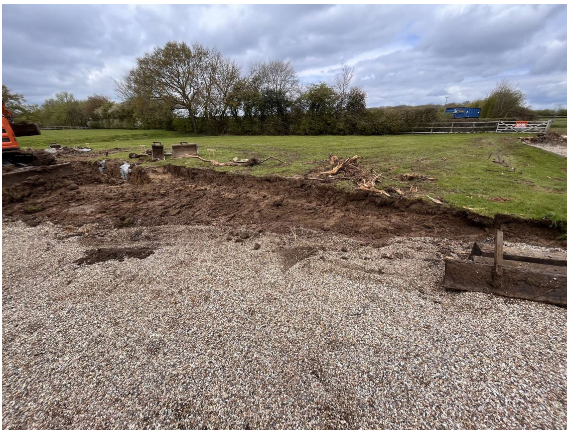
Photograph 5 Soil reduction area, looking north-west.
