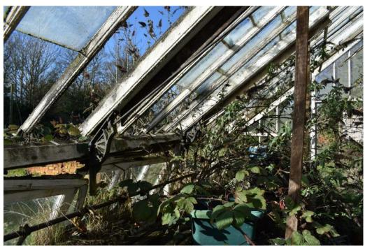
**Photograph 13** Detail of cast iron eave spandrels in glasshouse. Photograph taken facing south-west.
