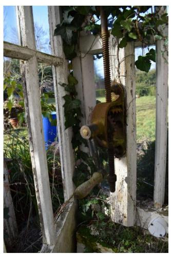
Photograph 16 Detail of cast and wrought iron upper window opening/closing mechanism in glasshouse. Photograph taken facing west.
