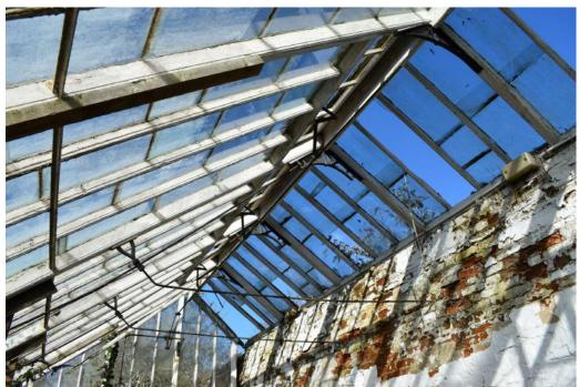
**Photograph 12** Detail of glasshouse roof showing cast iron ridge spandrels and wrought iron supports. Photograph taken north-west.
