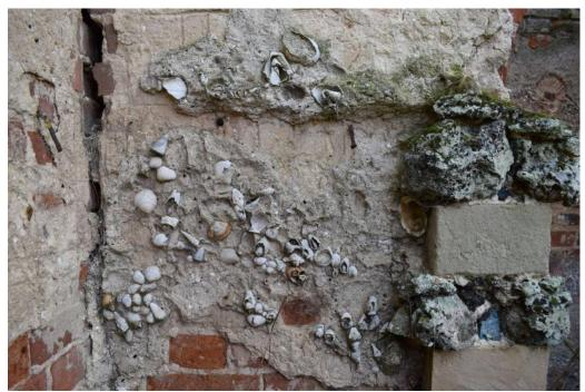
**Photograph 18** Detail of shells in plaster on southern wall. Photograph taken facing south-west.
