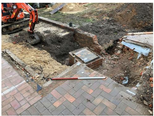
Photograph 2 Excavations around the drain, looking south-east.
