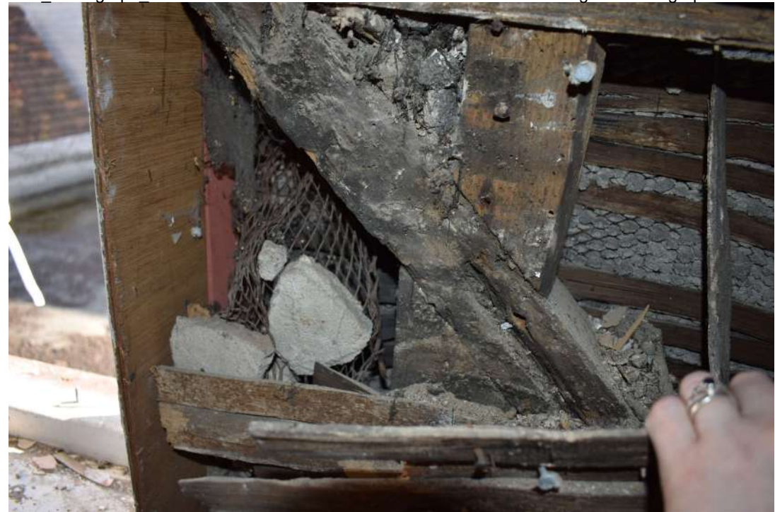
CF98_Photograph_140Detail of original plaster in north-east wall of north-west range. Photograph tak...
