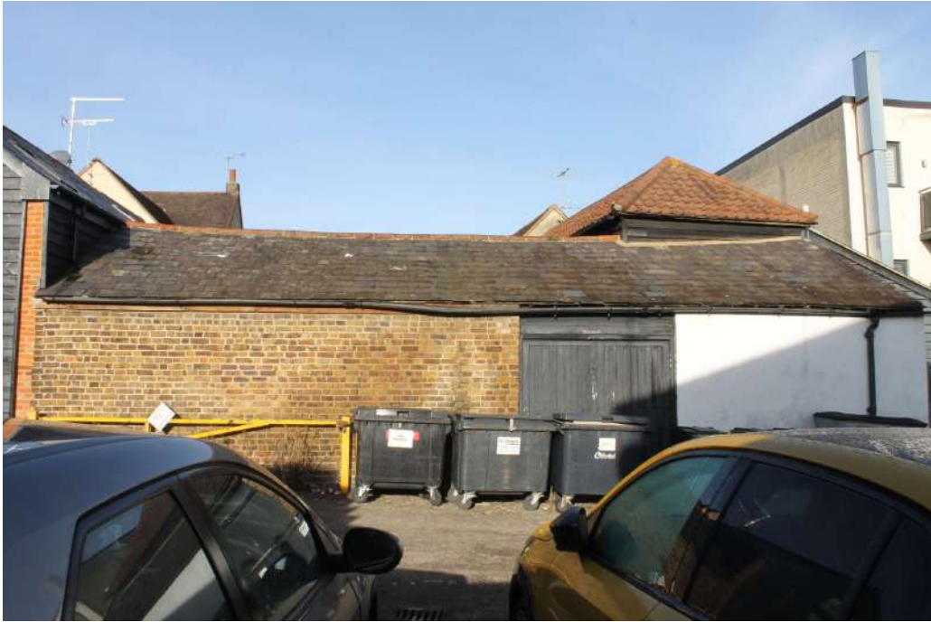
Photograph 6 South-east elevation. Photograph taken facing north-west.
