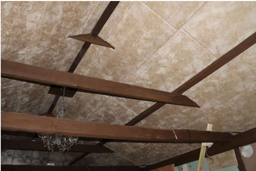
Photograph 17 Detail of roof structure in range 3. Photograph taken facing north-east.
