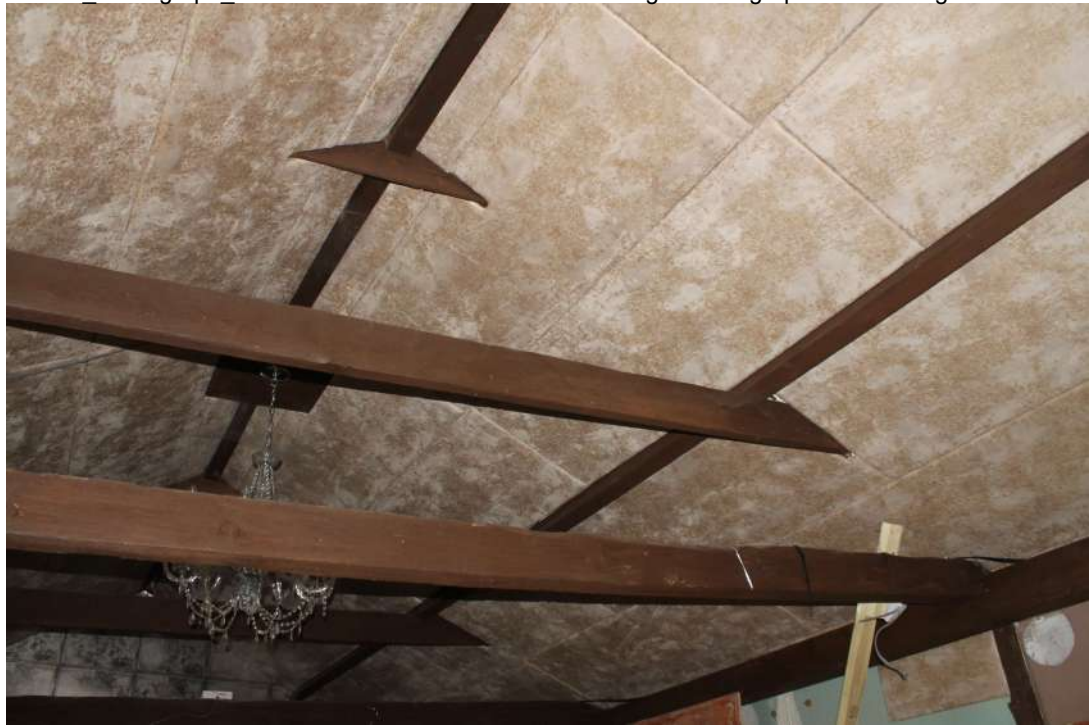
CF98_Photograph_044Detail of splayed scarf joint on western purlin in south range.
