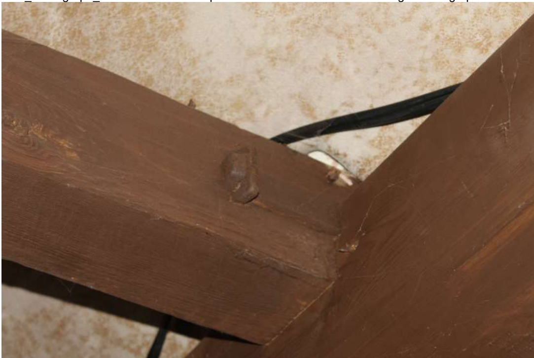
CF98_Photograph_043Detail of iron strap on southern tie-beam in south range. Photograph taken facing north-east.
