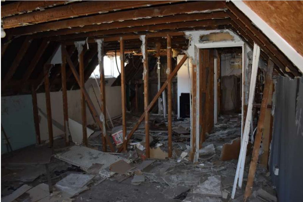
Photograph 30 Internal shot of range 10. Photograph taken facing north-east.
