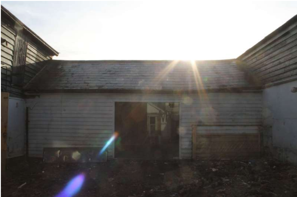
Photograph 11 North-west courtyard elevation. Photograph taken facing south-east.
