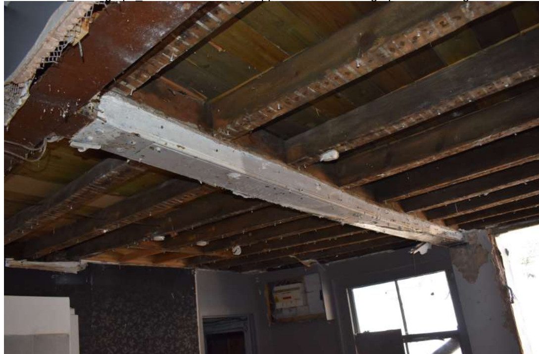
CF98_Photograph_120Detail of timber-framing, including laths, in south-eastern wall of north-west ra...
