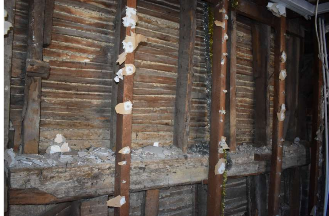
CF98_Photograph_131Detail of laths in north-eastern wall of middle range B. Photograph taken facin... CF98_Photograph_132Detail of laths in ceiling of middle range B. Photograph taken facing north-west.
