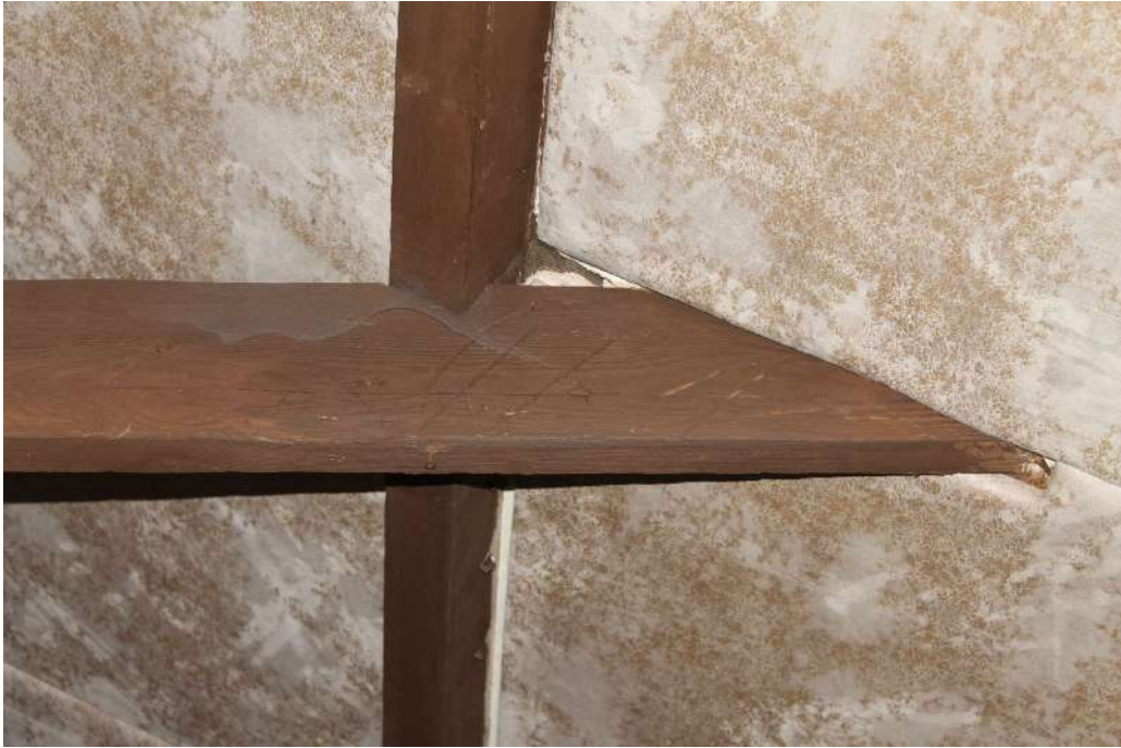
Photograph 18 Detail of Baltic timber mark on southern tie-beam in range 3. Photograph taken facing north-east.
