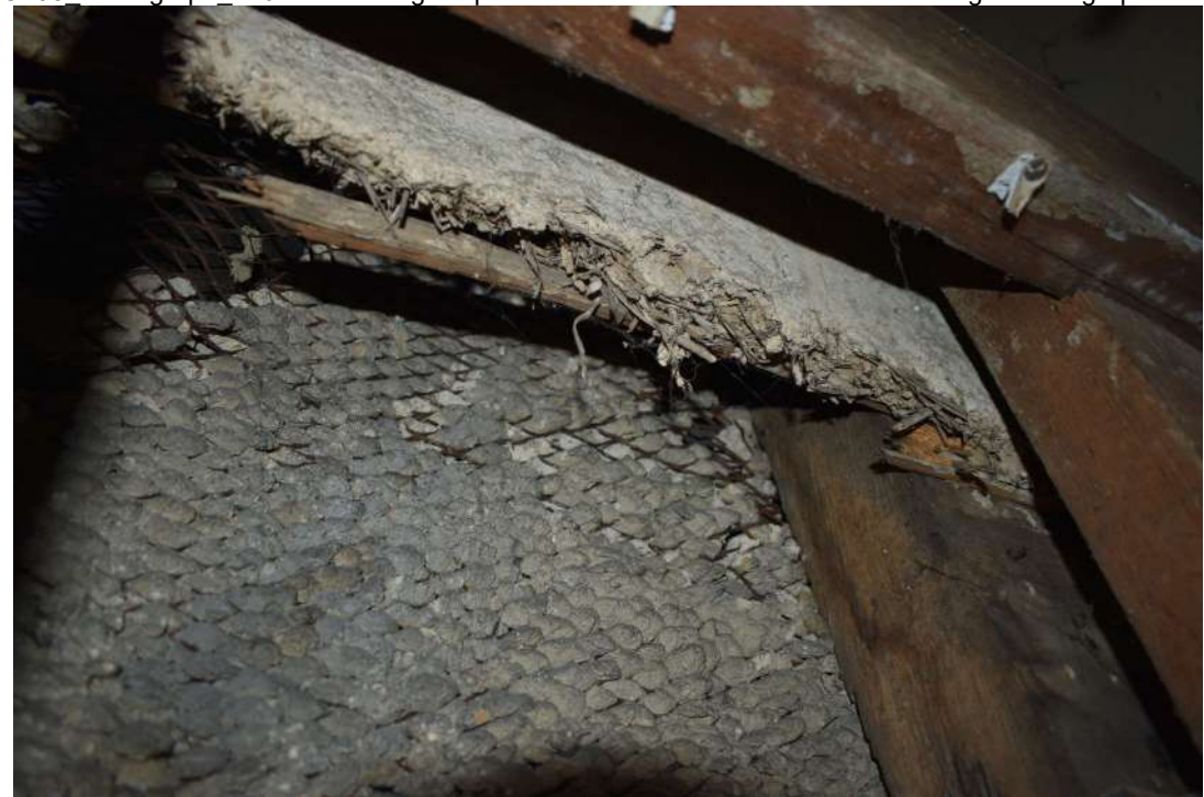
CF98_Photograph_140Detail of original plaster in north-east wall of north-west range. Photograph tak...
