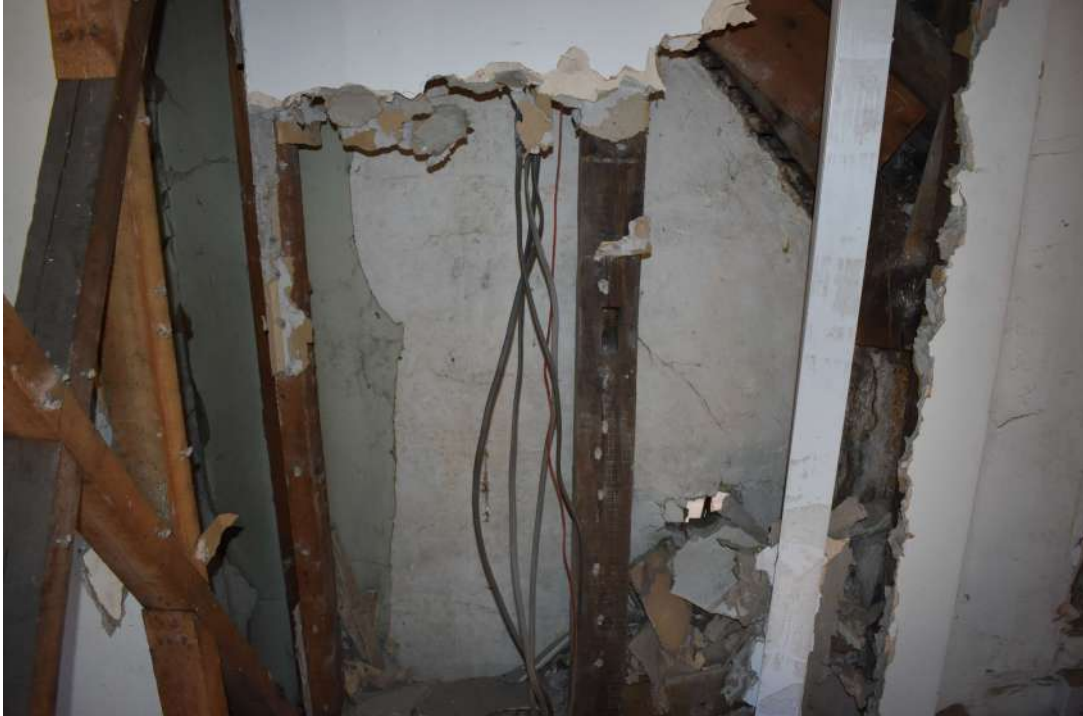
CF98 Photograph 123Detail of reused timber in north-east wall of north-west range. Photograph tak...
