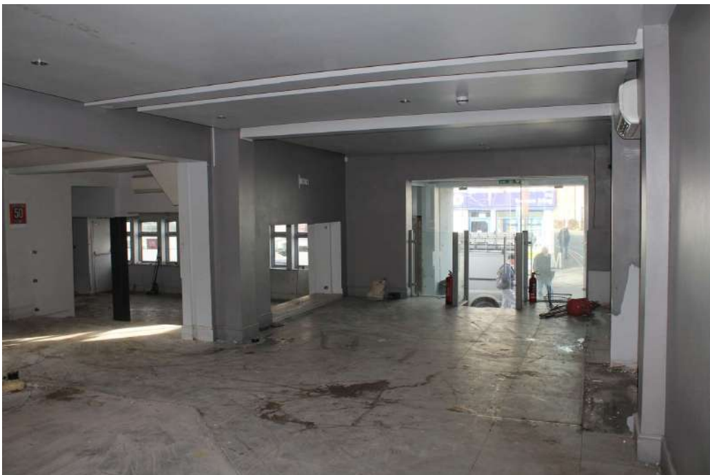
Photograph 23 Internal view of range 6 and range 5, showing modern interior. Photograph taken facing west.
