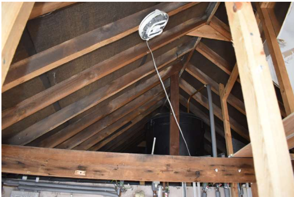
Photograph 12 Detail of roof construction of ranges 2 and 4. Photograph taken facing north.
