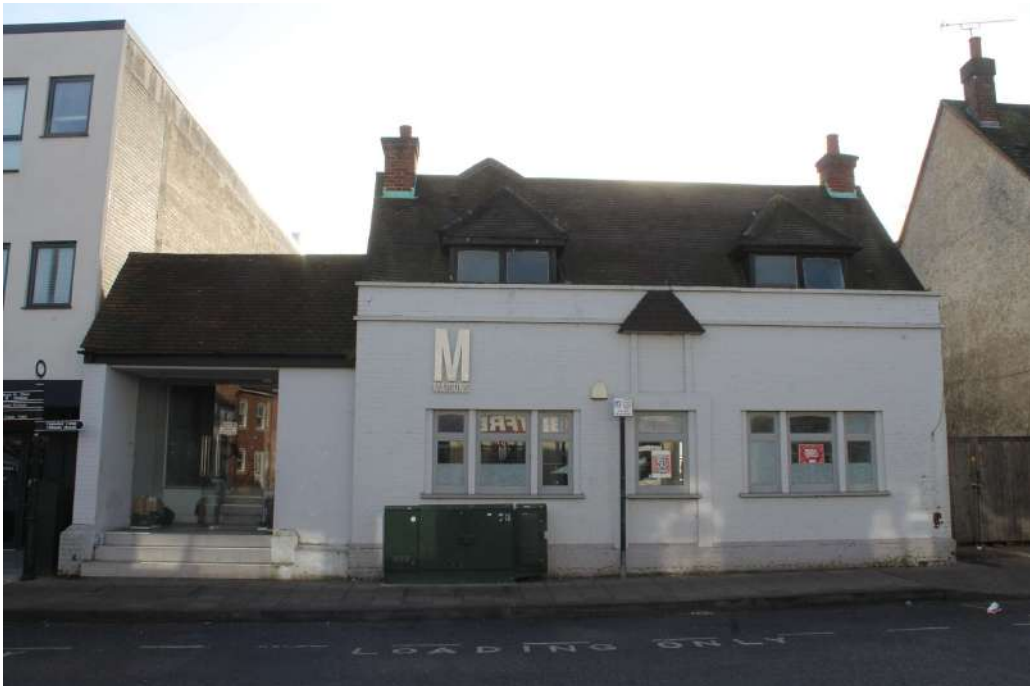
Photograph 2 North-west elevation. Photograph taken facing south-east.
