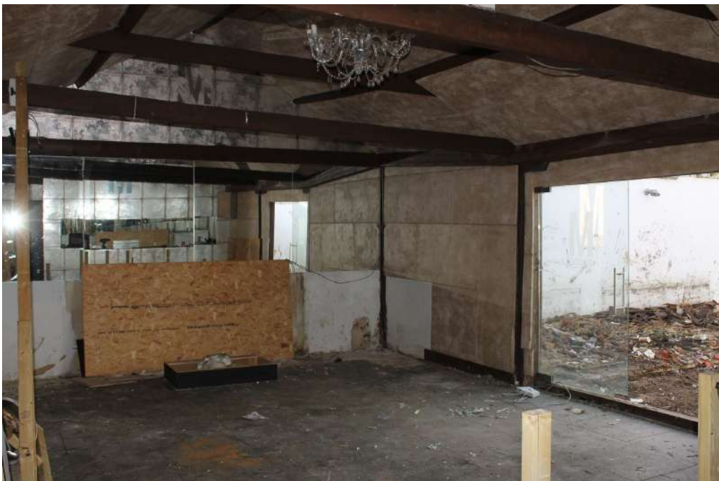
Photograph 29 Internal view of range 3. Photograph taken facing west.
