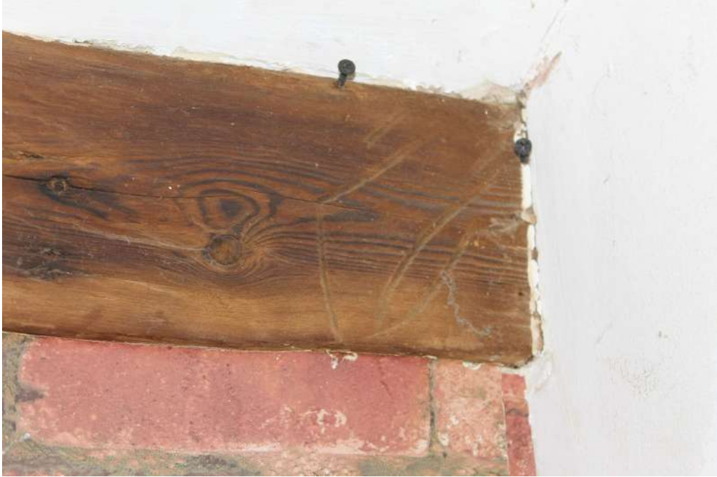
Photograph 14 Detail of Baltic timber mark on wall-plate of range 2. Photograph taken facing west south-west.
