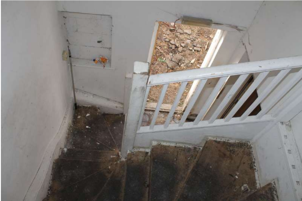
Photograph 26 Internal view of stairwell in range 6. Photograph taken facing south-west.
