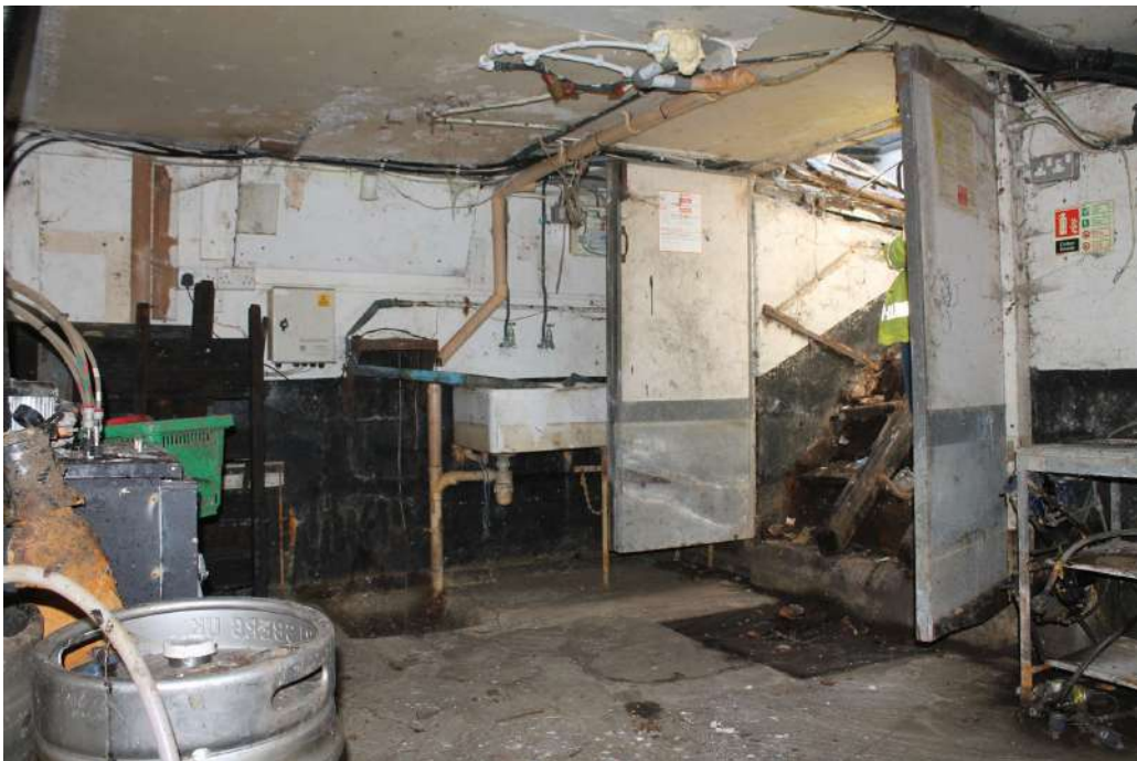
Photograph 19 Internal view of cellar. Photograph taken facing south.
