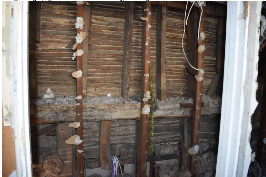
CF98_Photograph_120Detail of timber-framing, including laths, in south-eastern wall of north-west ra...
