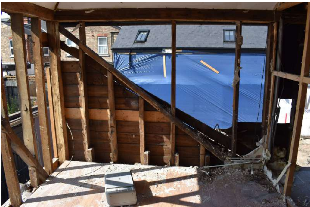
Photograph 36 Interior of bedroom 4, showing timber-frame. Photograph taken facing south-west.
