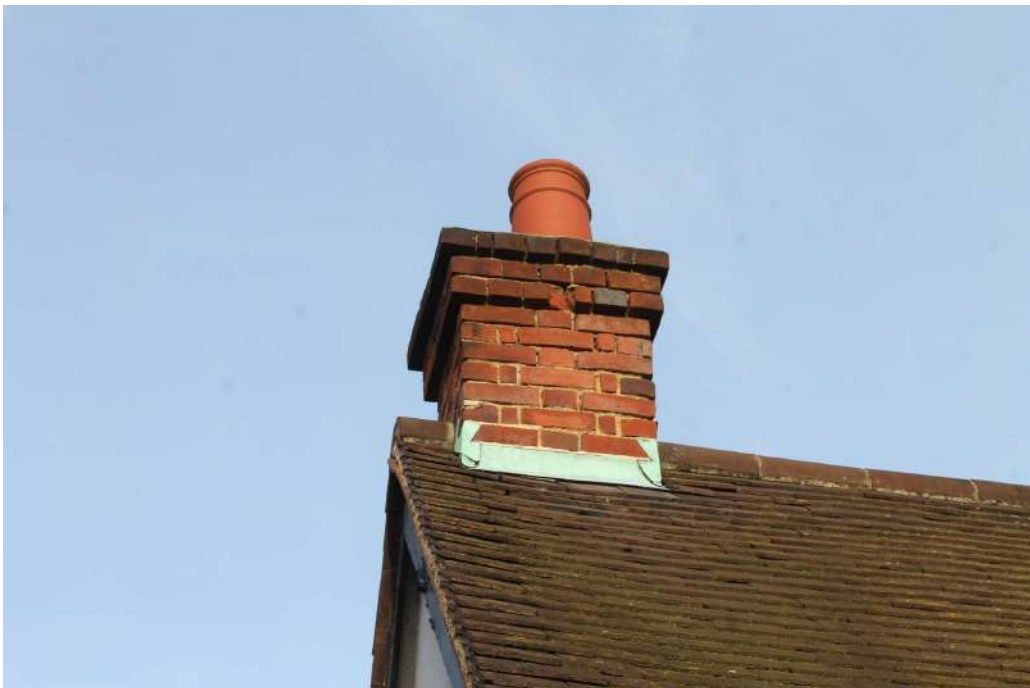
Photograph 4 Detail of southern chimney stack. Photograph taken facing north.
