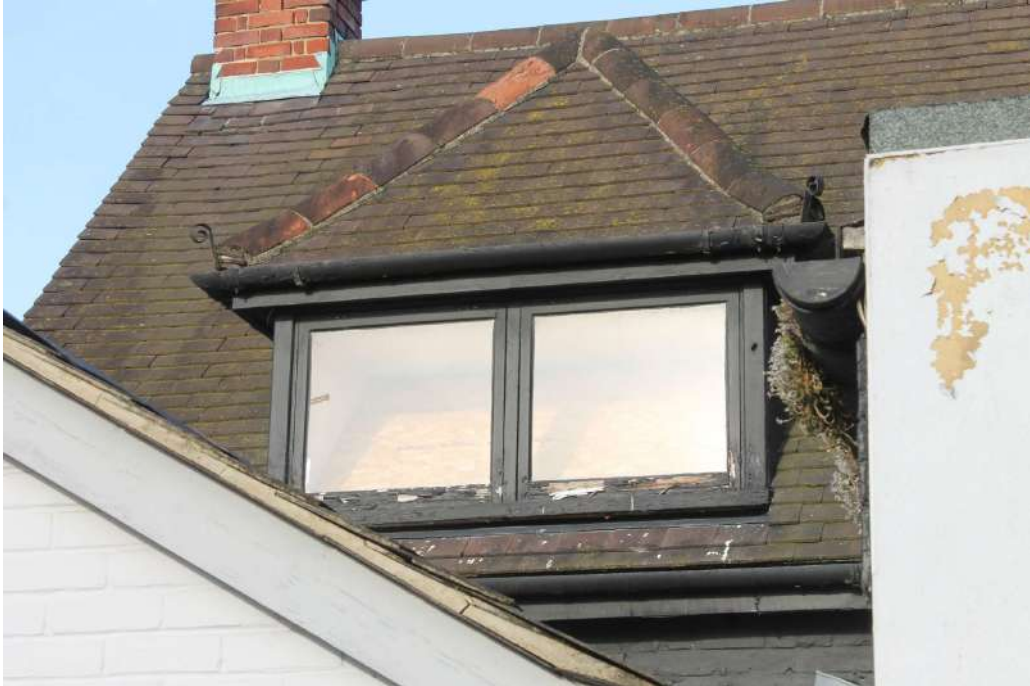
Photograph 3 Detail of window on south-east courtyard elevation. Photograph taken facing north-west.
