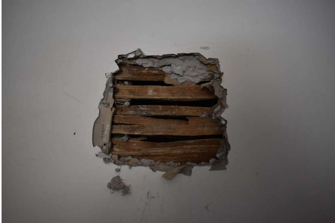
CF98_Photograph_143Detail of laths in north-east wall of middle range B. Photograph taken north-we...
