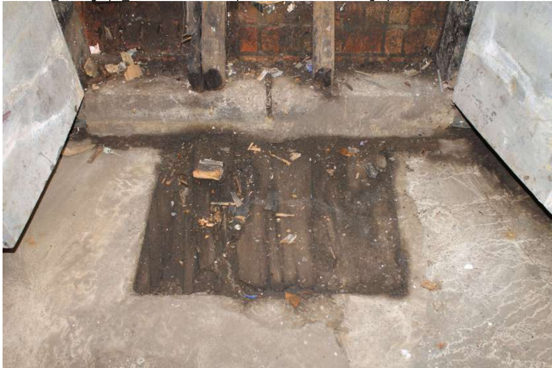
CF98_Photograph_035Detail of timber pad in cellar floor. Photograph taken facing south-west.
