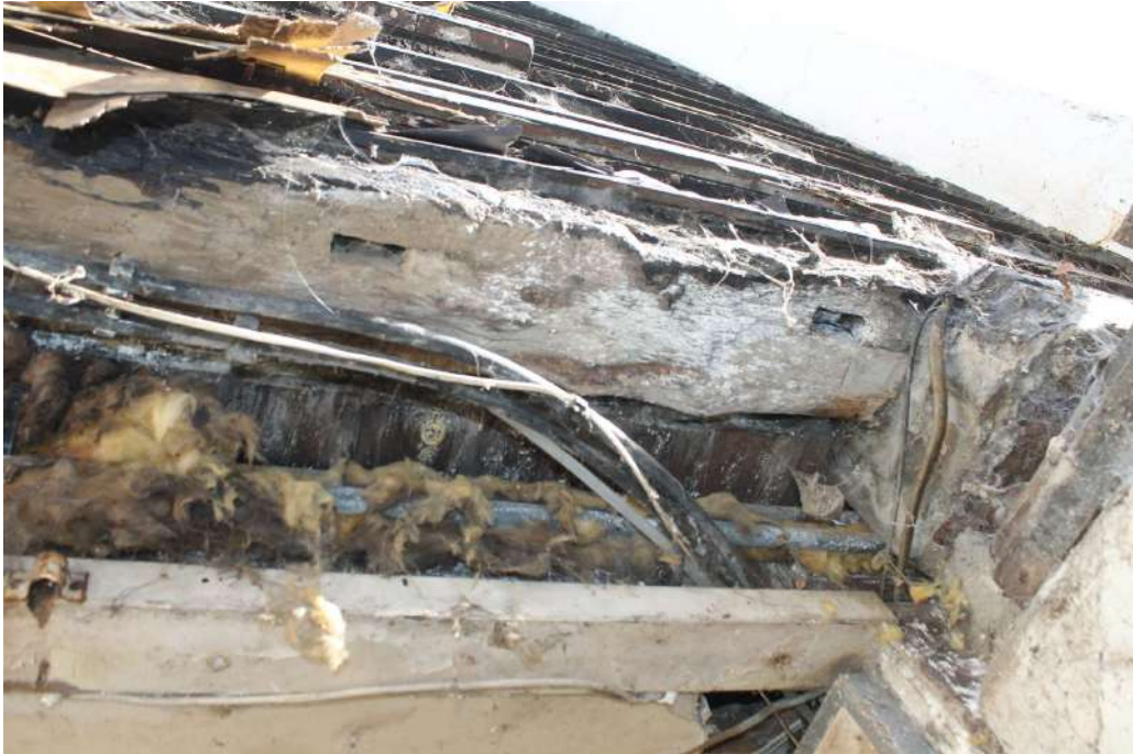
Photograph 20 Detail of mortices in reused beam in cellar entrance.
