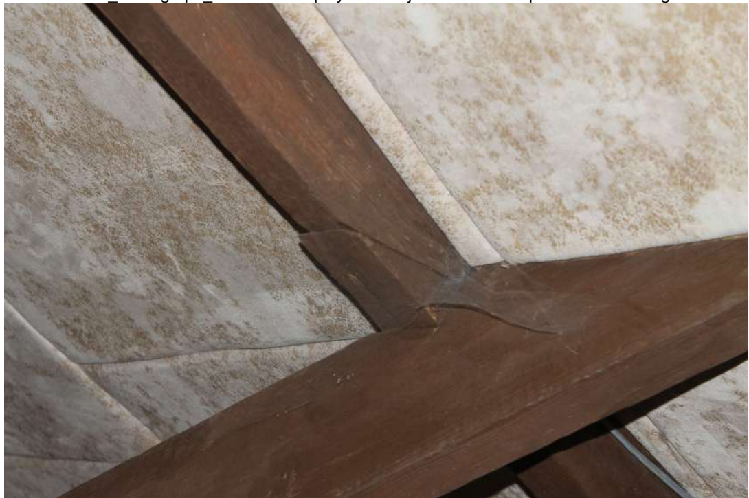
CF98_Photograph_044Detail of splayed scarf joint on western purlin in south range.
