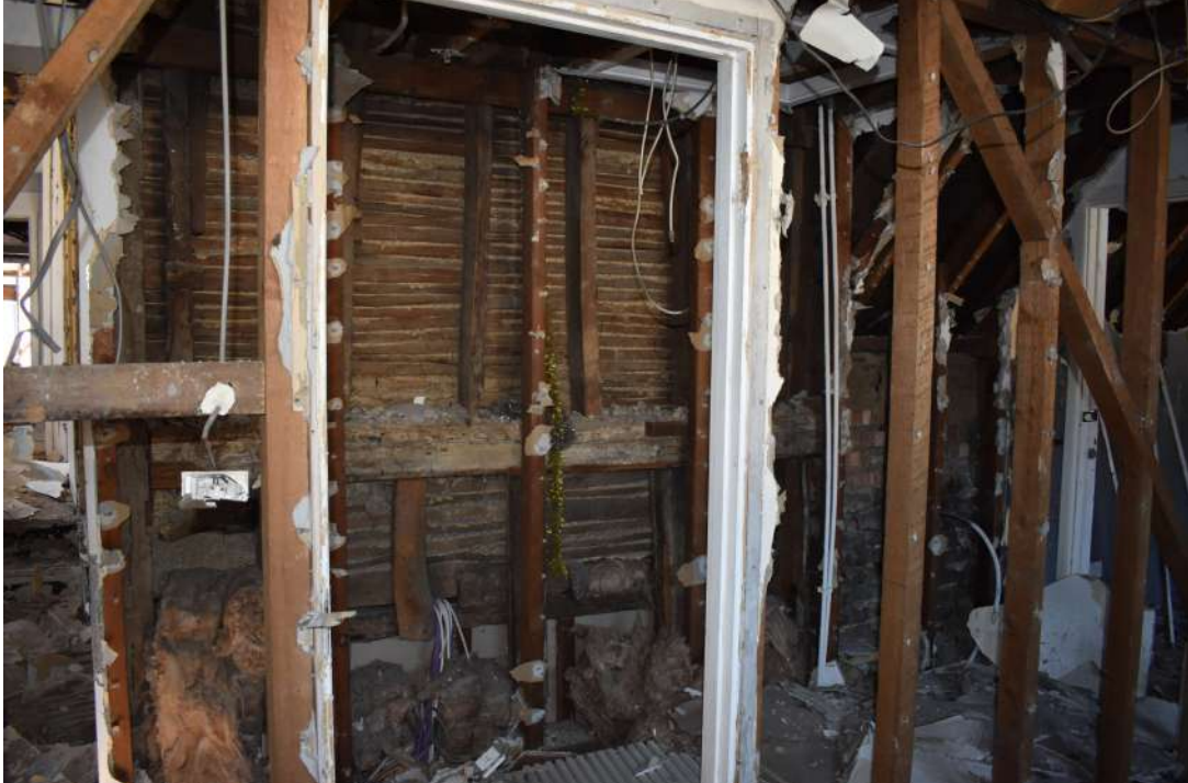
CF98 Photograph 123Detail of reused timber in north-east wall of north-west range. Photograph tak...
