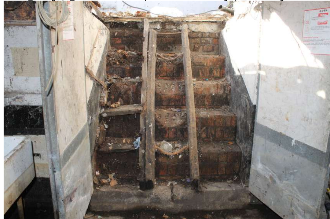
CF98_Photograph_036Detail of mortices in reused beam in cellar entrance.
