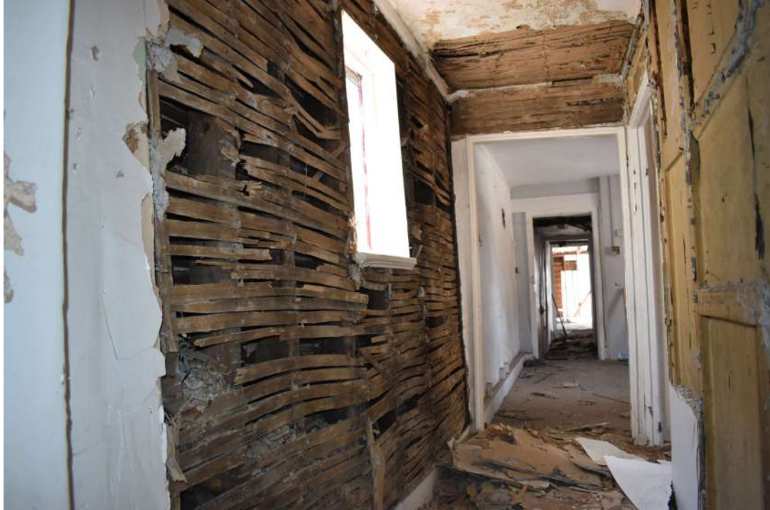
CF98_Photograph_131Detail of laths in north-eastern wall of middle range B. Photograph taken facin... CF98_Photograph_132Detail of laths in ceiling of middle range B. Photograph taken facing north-west.
