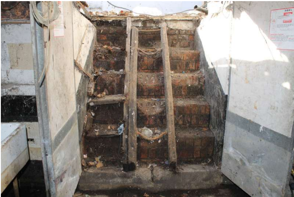
Photograph 21 Detail of cellar steps with barrel-run. Photograph taken facing south-west.
