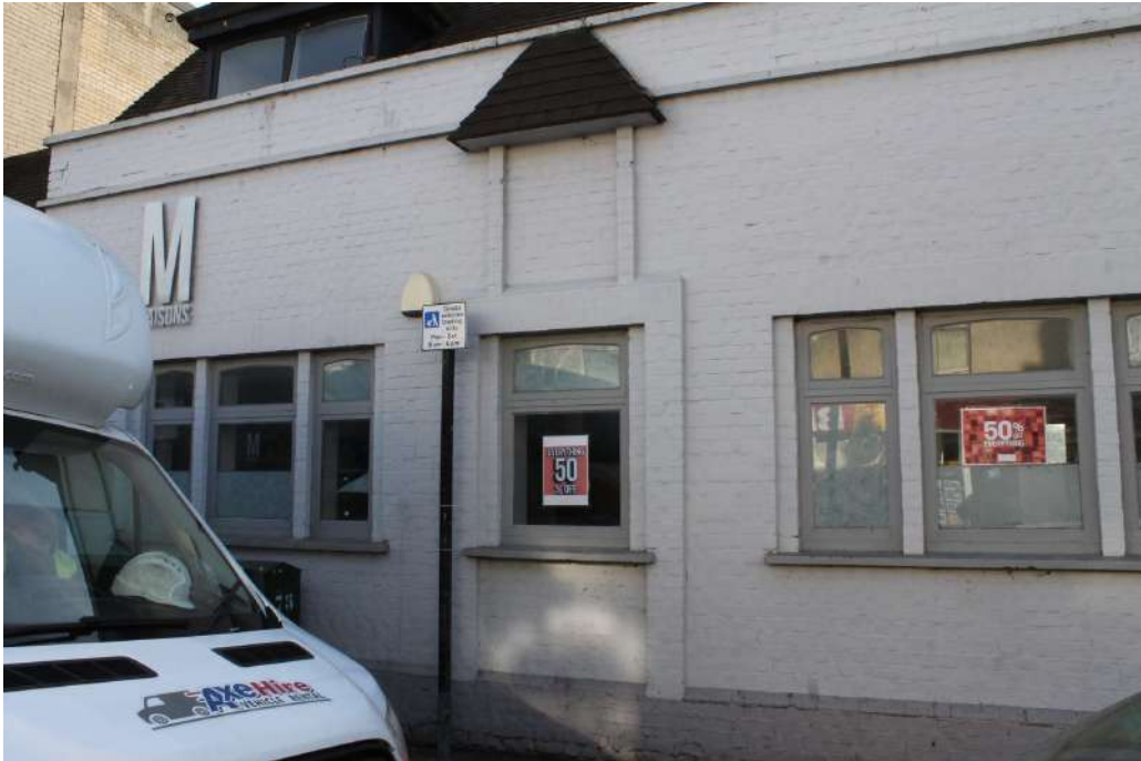
Photograph 5 North-west elevation of range 10. Photograph taken facing south-east.
