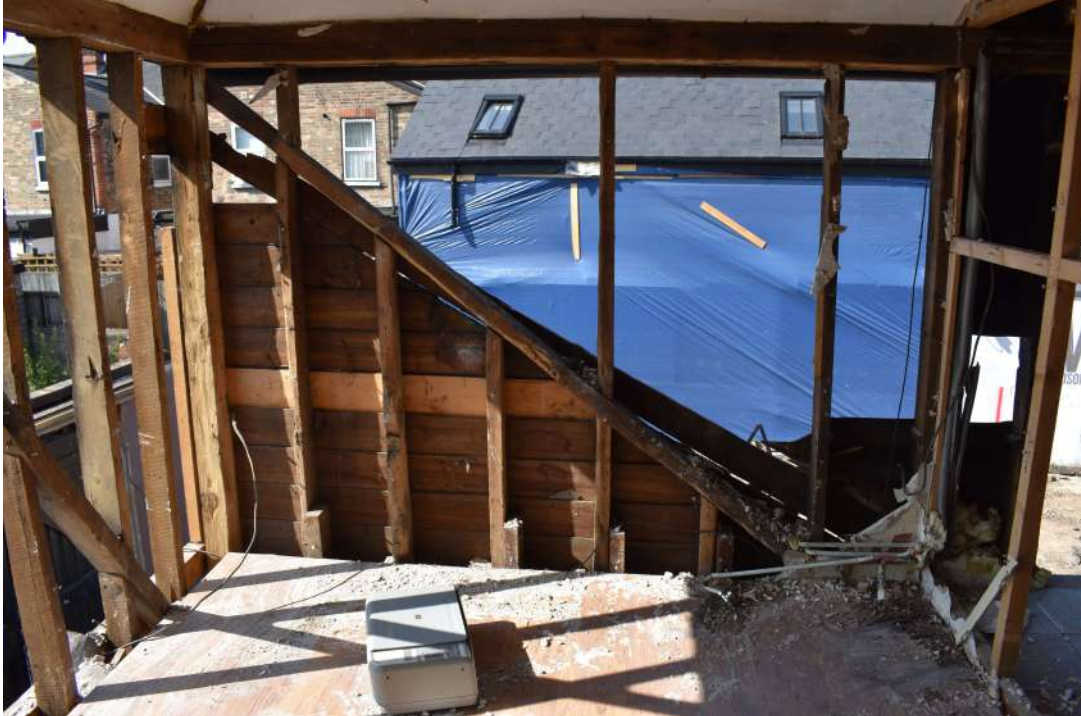
CF98_Photograph_147Interior of middle range A (first floor), showing timber-frame. Photograph taken... CF98_Photograph_148Detail of roof construction of middle range A. Photograph taken facing north-w...
