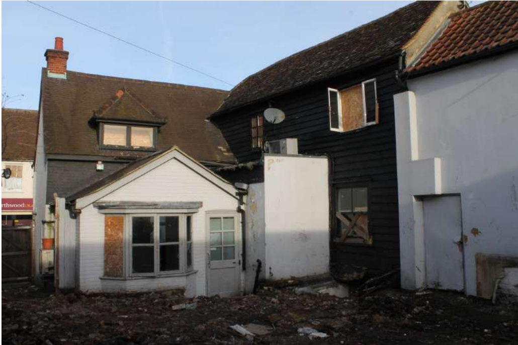
Photograph 10 South-west and south-east courtyard elevation. Photograph taken facing north.
