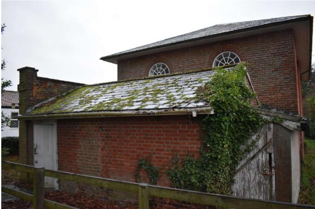
Photograph 6 South elevation. Photograph taken facing north-west.
