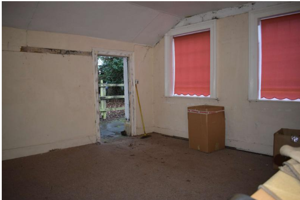
Photograph 20 Internal view of vestry. Photograph taken facing south-west.
