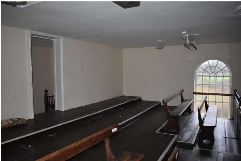
Photograph 19 Internal view of gallery. photograph taken facing north-east.
