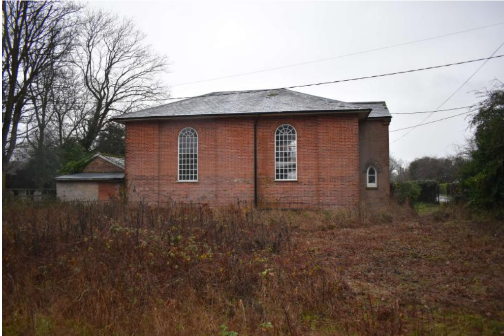
Photograph 4 East elevation. Photograph taken facing west.
