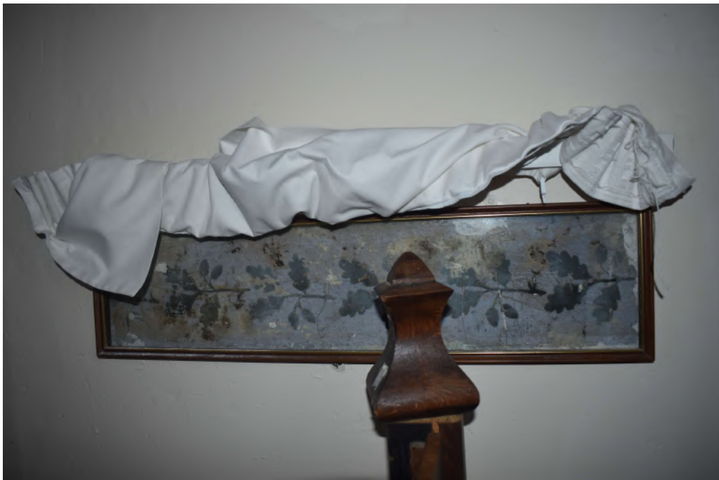
Photograph 13 Detail of preserved painting in main hall. Photograph taken facing south.
