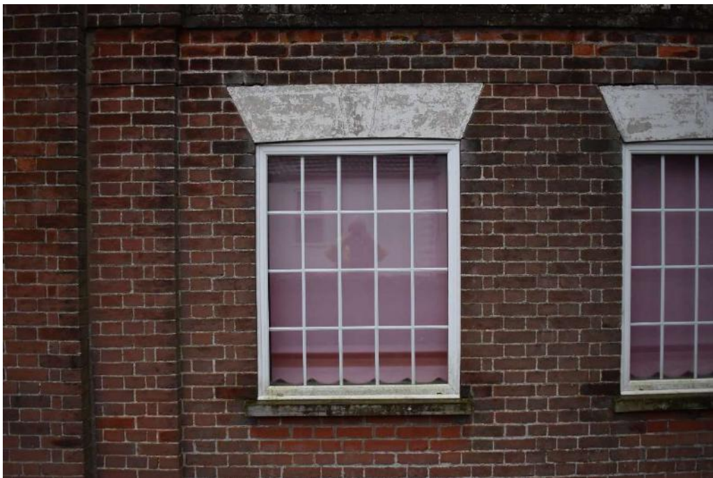
Photograph 9 Detail of PVC window on west elevation. Photograph taken facing east.
