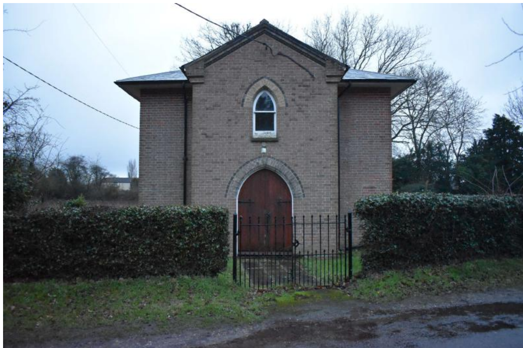
Photograph 1 North elevation. Photograph taken facing south.
