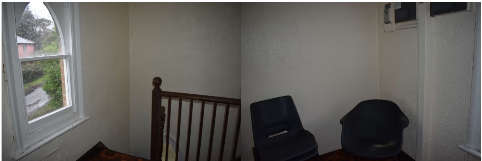
ECC4764_PhotoGraph_081Internal view of landing. Photograph taken ... ECC4764_PhotoGraph_082Detail of internal door between landing and...
