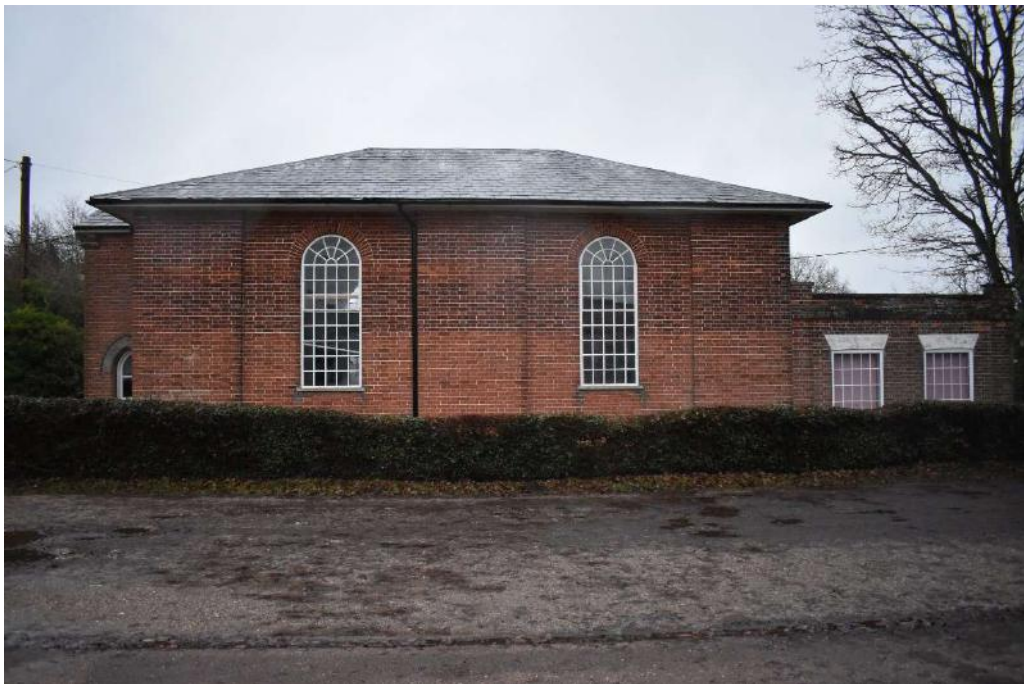
Photograph 7 West elevation. Photograph taken facing east.
