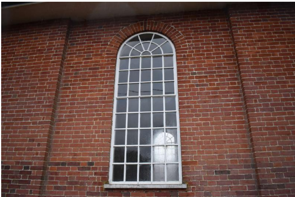
Photograph 5 Detail of window on east elevation. Photograph taken facing west.
