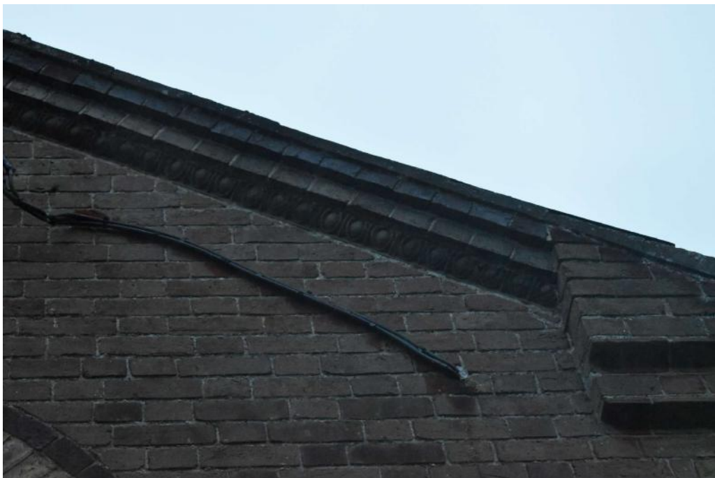
Photograph 3 Detail of decorative brickwork on north elevation. Photograph taken facing south.
