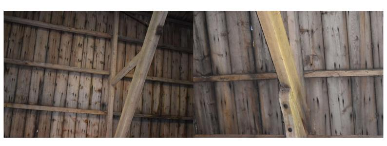
$CFTF22\_Photograph\_099Detail\ of\ upper\ scarf-joint\ in\ purlin\ in\ eastern...\ CFTF22\_Photograph\_100Detail\ of\ scarf-joints\ in\ purlin\ in\ eastern\ roof\ ...$
