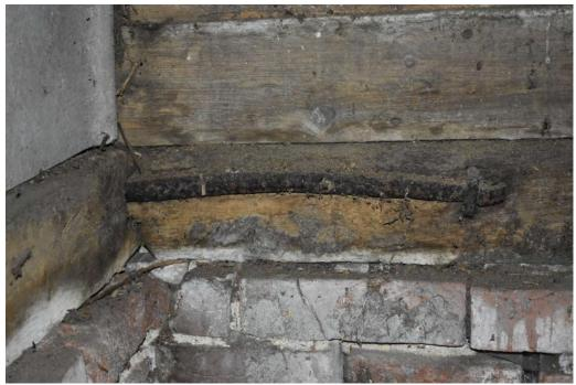
Photograph 18 Detail of iron strap on sill-beam of northern wall of bay 5 of barn. Photograph taken facing north.
