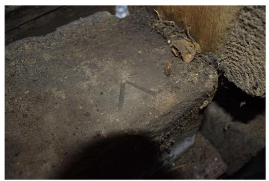
**Photograph 14** Detail of carpenters' mark 'V' on sill-beam on western wall of bay 2 in barn. Photograph taken facing north.
