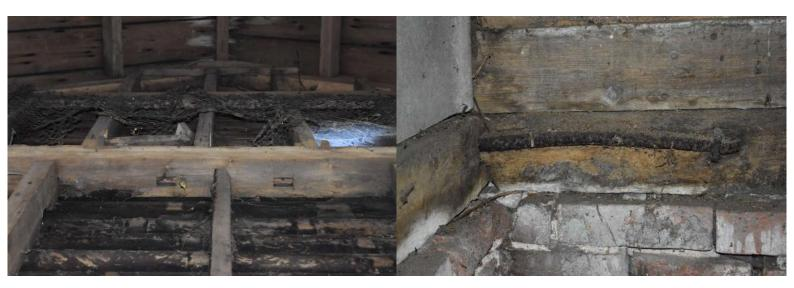
CFTF22\_Photograph\_125Detail of iron strap on sill-beam of northern ... CFTF22\_Photograph\_126Detail of scarf joint on sill-beam in eastern w...
