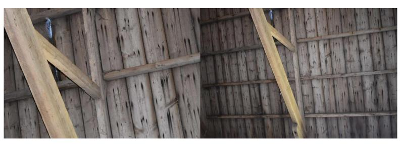
CFTF22\_Photograph\_101Detail of scarf-joint in wall-plate of western w... CFTF22\_Photograph\_102Detail of scarf-joint in wall-plate of eastern w...
