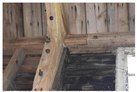
**Photograph 15** Detail of scarf-joint in wall-plate of western wall of bay 3 of barn. Photograph taken facing south-west.
