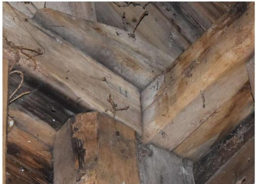
**Photograph 13** Detail of carpenters' mark 'll' on gable-tie and wall-plate in north-west corner of bay 1 in barn. Photograph taken facing north.
