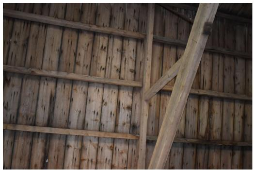
**Photograph 10** Detail of scarf-joints in purlin in eastern roof pitch between bays 2 and 3 of the barn. Photograph taken facing south-east.
