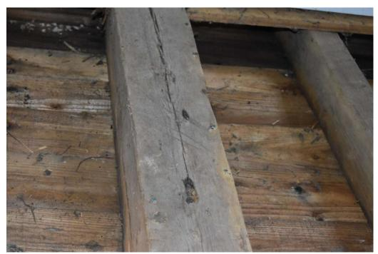
**Photograph 19** Detail of Baltic timber mark on post of eastern wall between bays 4 and 5. Photograph taken facing south-east.
