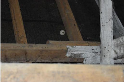
**Photograph 21** Detail of scarf-joint in purlin on the northern pitch of the roof of the store 5. Photograph taken facing north.
