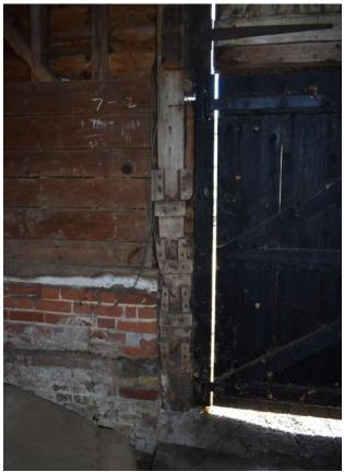
Photograph 16 Detail of wooden blocks adjacent to barn door on eastern wall.
