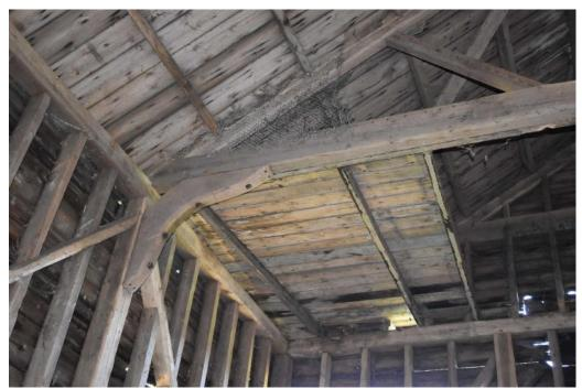
**Photograph 17** Detail of inserted loft level in bay 5 of barn. Photograph taken facing north.
