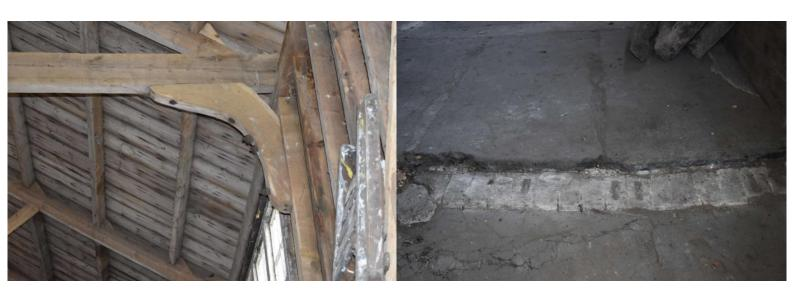
CFTF22\_Photograph\_129Detail of scarf joint in sill-beam on eastern w... CFTF22\_Photograph\_130Detail of Baltic timber mark on post of easter...
