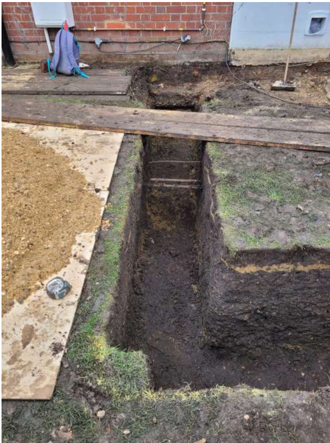
Photograph 4 Working shot of trench, south-south-east
