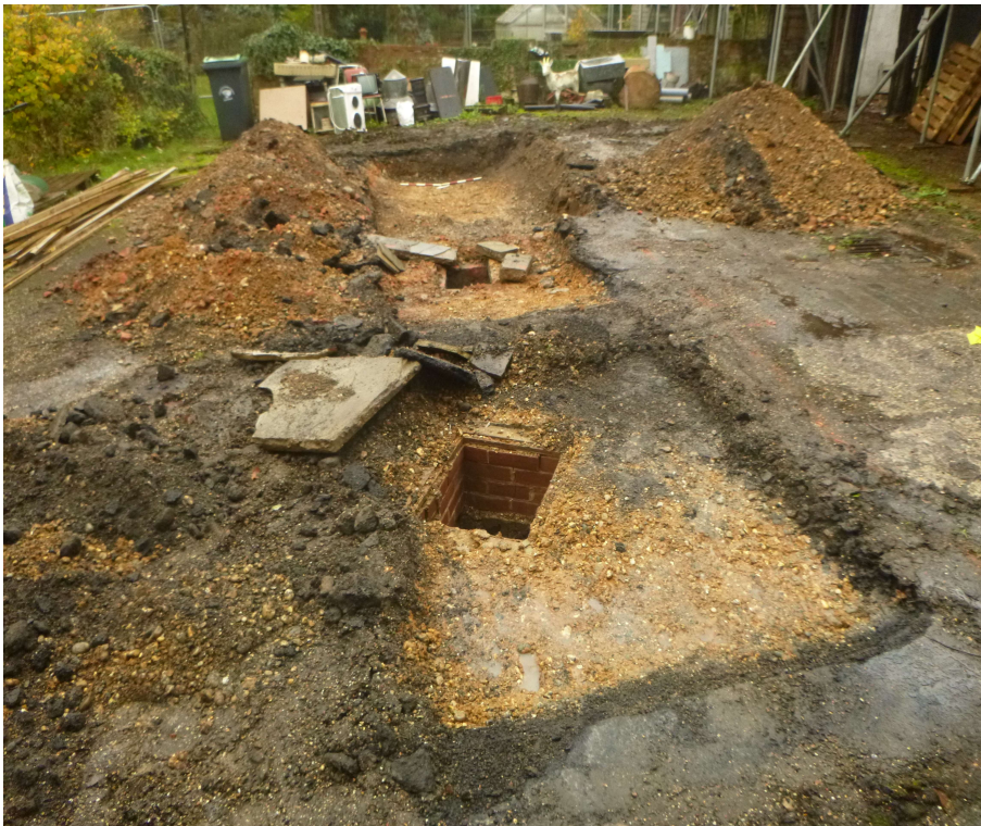
Photograph 1 Trench 3 showing well, looking south-east
