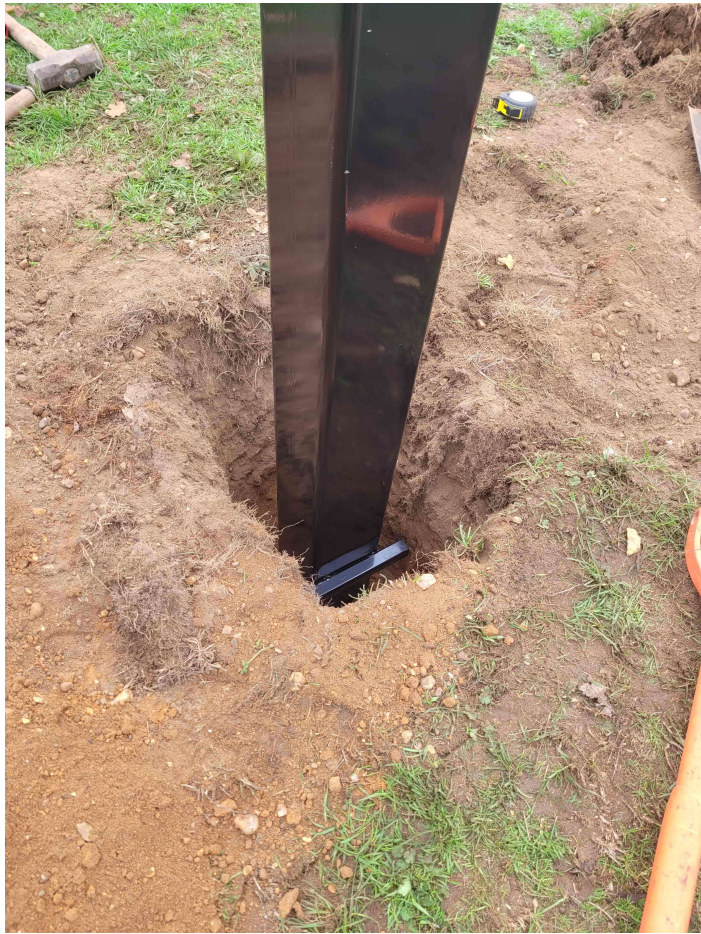
Photograph 3 Installation of panel 1
