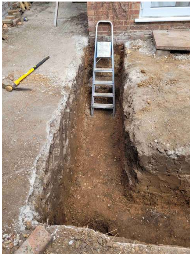
Photograph 3 Western foundation, looking north-north-east
