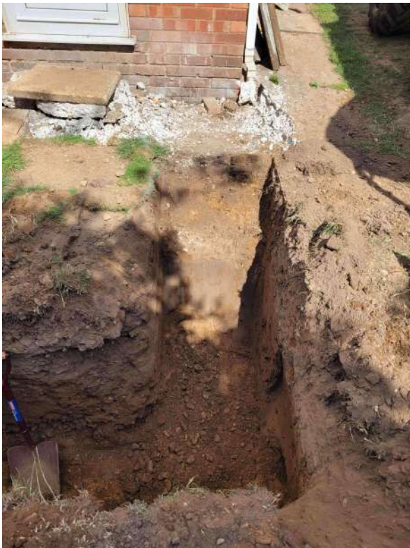
Photograph 5 Eastern foundation, looking north-north-east
