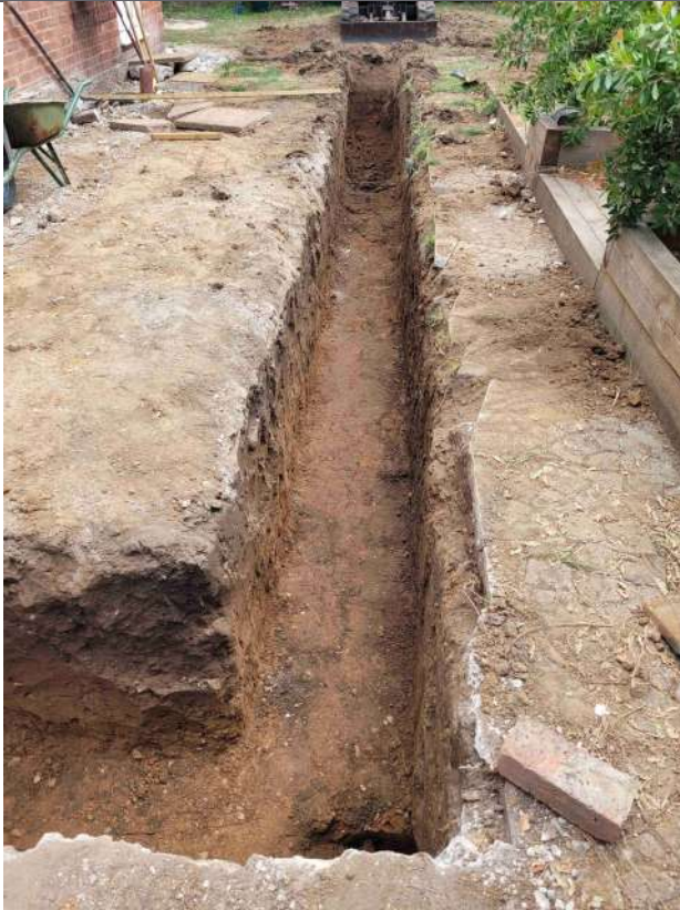
Photograph 4 South foundation, looking east-south-east
