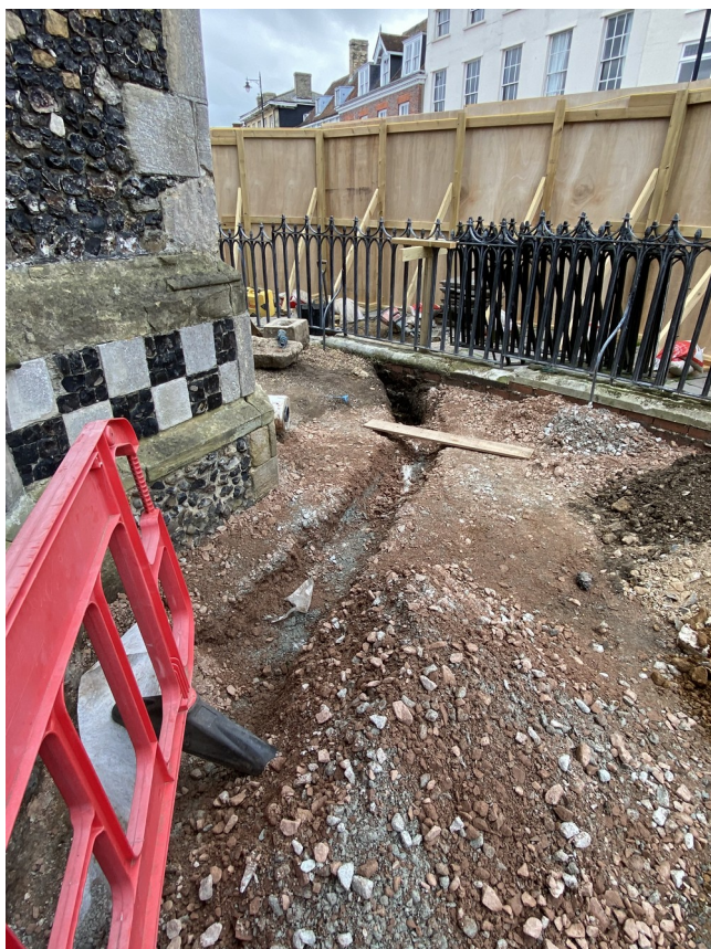
Photograph 6 Trench at north end of site, looking roughly west.
