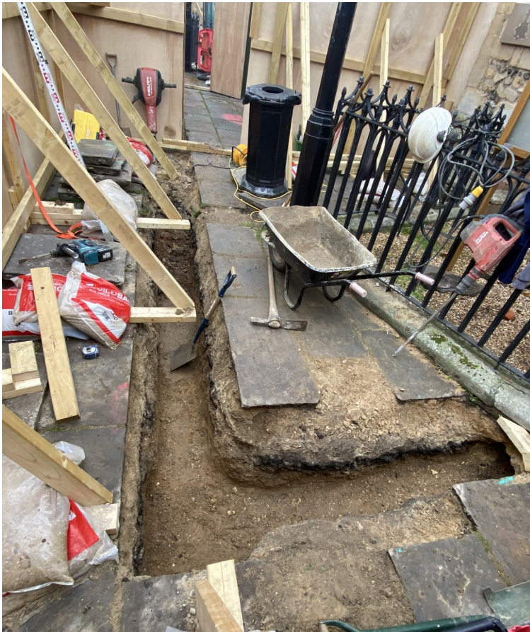
Photograph 1 Trenching at south end of site, looking north
