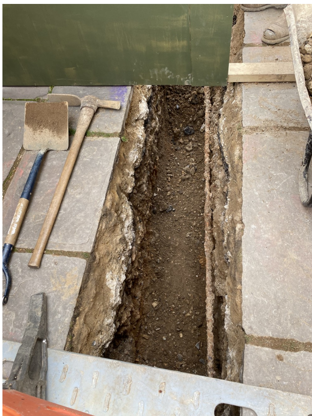
Photograph 5 North end of middle trenching, looking north
