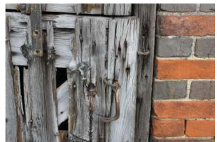
PLSB22_Photograph_13 Door furniture on stable door
