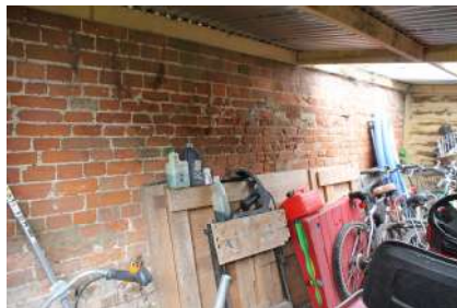
PLSB22_Photograph_24Interior of timber lean to show ing east w all
