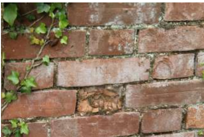
PLSB22_Photograph_27Graffiti on east wall
