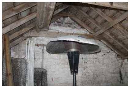
PLSB22_Photograph_30Interior stable show ing roof to apex
