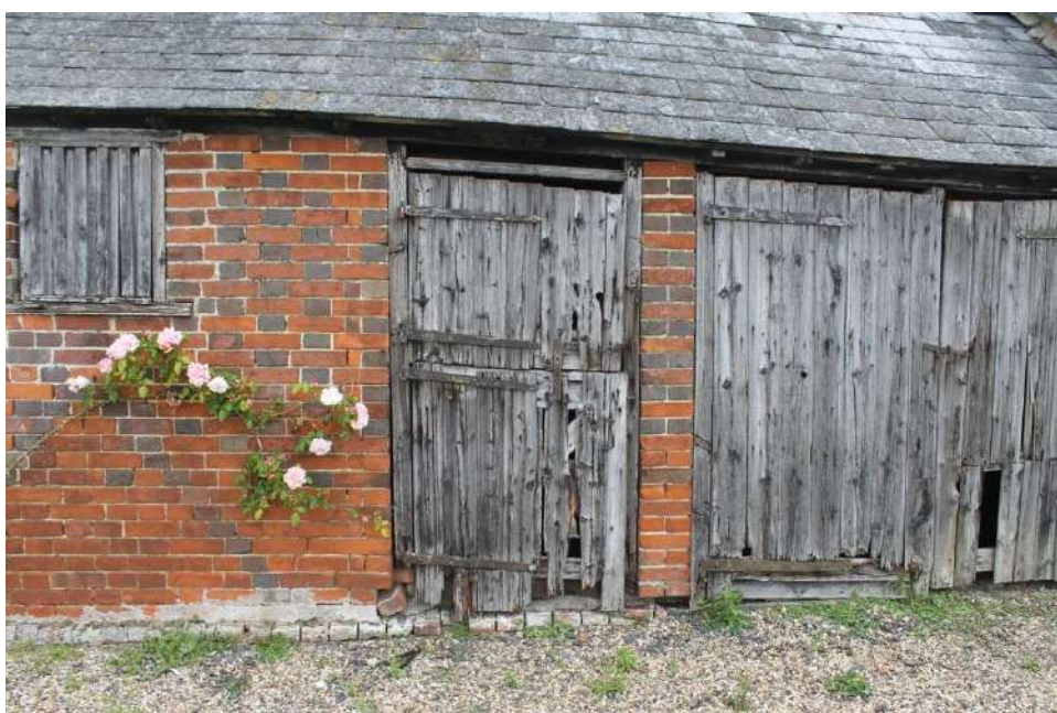
Photo 3: The vertical-slatted doors and window in the western façade of the stable and cart lodge.
