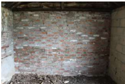
PLSB22_Photograph_49Internal south wall of cattle barn
