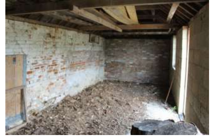
PLSB22_Photograph_45Interior of cattle barn (facing south)
