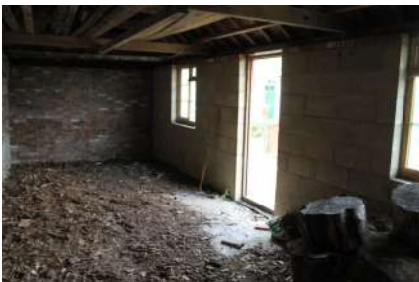
PLSB22_Photograph_44Interior of cattle barn (facing south)
