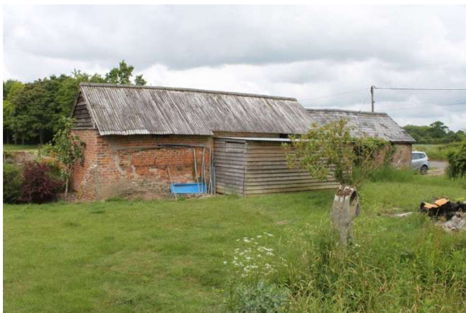
Photo 10: The eastern wall of the building.
