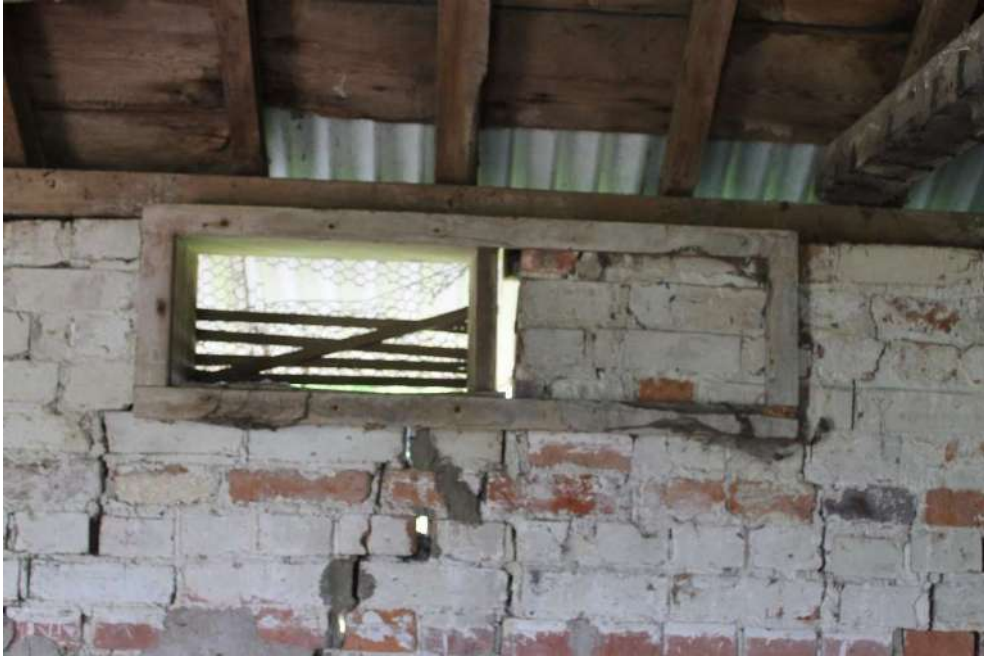
Photo 19: Window showing slatting and shutter array to the right.
