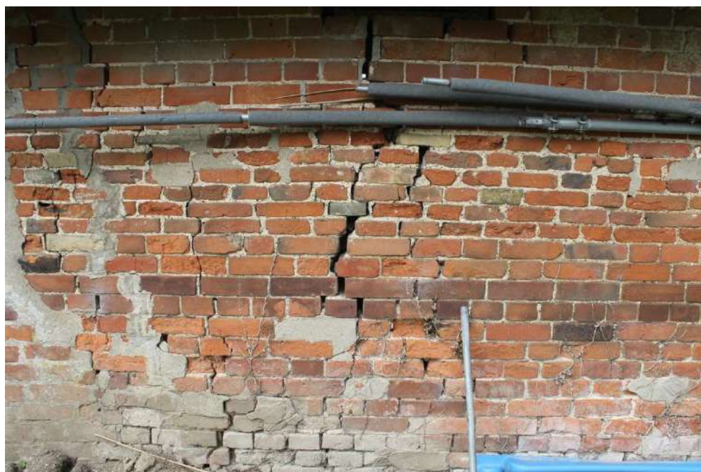
Photo 9: Detail of cattle shed wall showing irregular brickwork.
