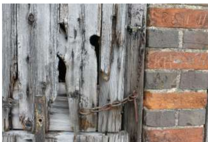
PLSB22_Photograph_12 Door furniture on stable door
