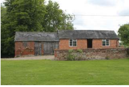
PLSB22_Photograph_01Exterior of building (west elevation)
