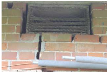
PLSB22_Photograph_22Small slatted ventilation window in east wall
