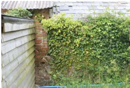
PLSB22_Photograph_25Join of the two parts of the building
