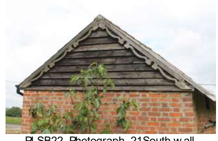
PLSB22_Photograph_21South wall, weatherboarding and decorative bargeboards
