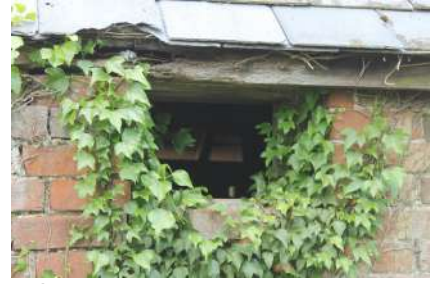
PLSB22_PhotoGraph_28Ventilation w indow in east w all
