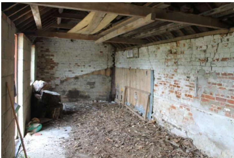
Photo 16: The interior of the cattle shed (facing north).
