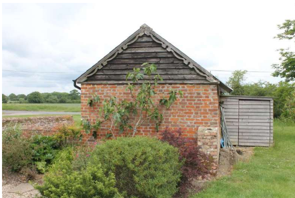
Photo 8: The northern wall of the building
