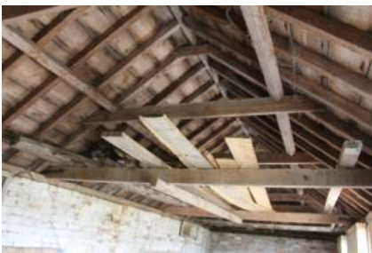
PLSB22_Photograph_46 Cattle barn roof
