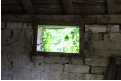
PLSB22_Photograph_31Internal ventilation window
