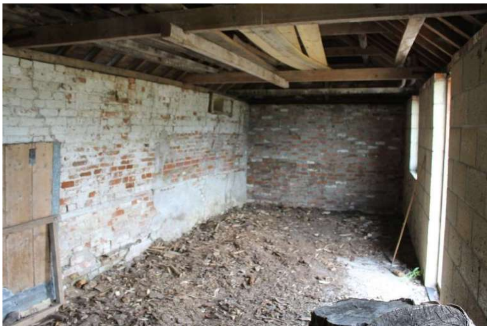
Photo 17: The interior of the cattle shed (facing south).
