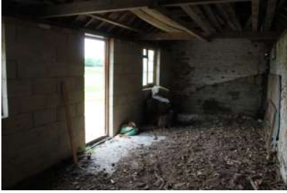
PLSB22_Photograph_43Interior of cattle barn (facing north)
