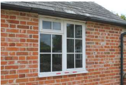
PLSB22_Photograph_20New window in cattle barn
