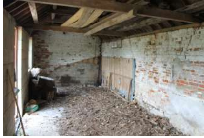
PLSB22_Photograph_42Interior of cattle barn (facing north)
