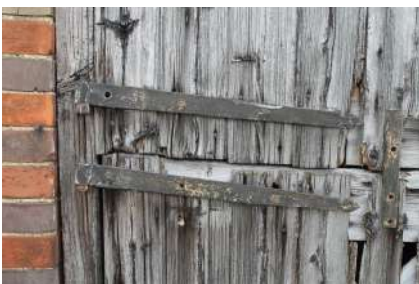
PLSB22_Photograph_11 Door furniture on stable door
