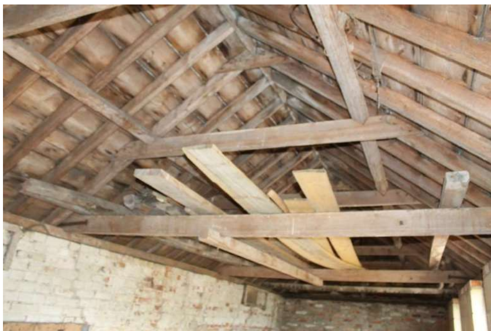
Photo 18: The roof of the cattle shed.
