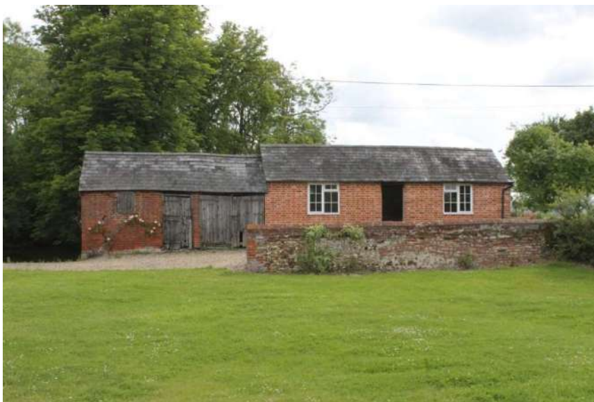
Photo 1: Exterior of building
