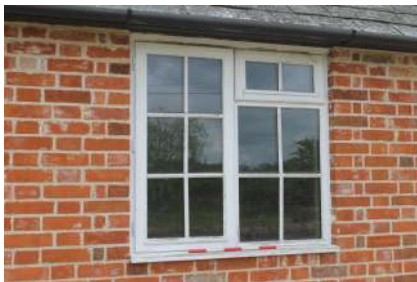
PLSB22_Photograph_19New window in cattle barn
