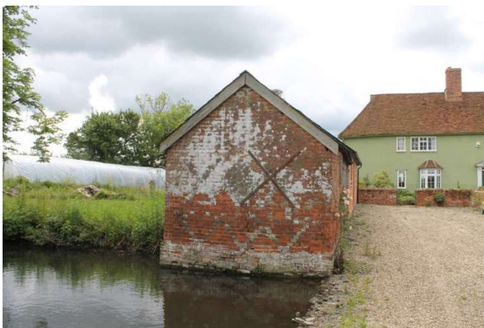
Photo 12: The northern wall of the building.
