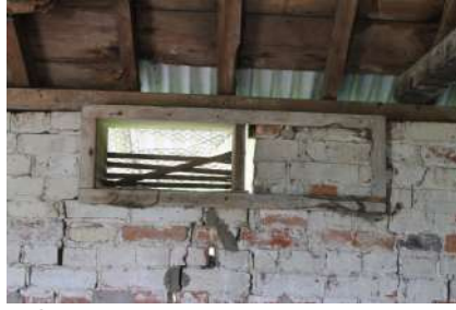
PLSB22_PhotoGraph_47Ventilation w indow in cattle barn
