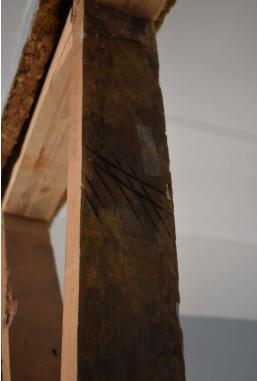
Photograph18 Detail of Baltic Timber marks in stud wall of room 16 and 17 (1st floor of no 63). Photograph taken facing east.
