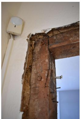
Photograph 19 Detail of timber pegs in doorway in room 17 (1st floor of no 63). Photograph taken facing south-east.
