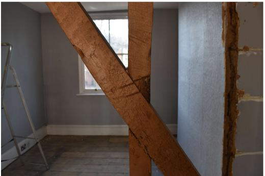
**Photograph 17** Detail of carpenters marks 'll' on stud and brace of stud wall of room 16 and 17 (1st floor of no 63). Photograph taken facing south-east.
