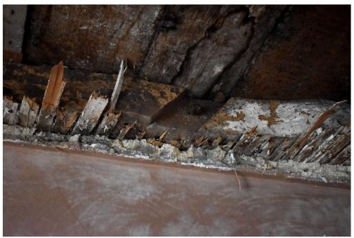
**Photograph 13** Detail of reused timber wall plate in Sitting Room. Photograph taken facing north-west.
