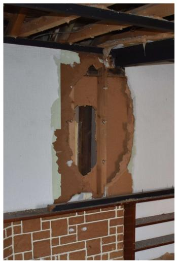
**Photograph 18** Detail of exposed stud wall in Bedroom 1. Photograph taken facing south-east.
