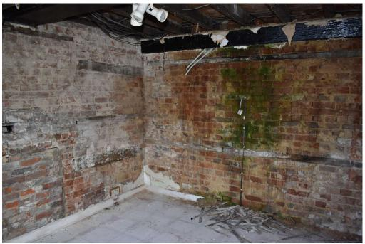
**Photograph 12** Interior shot of Study showing bond timbers. Photograph taken facing north
