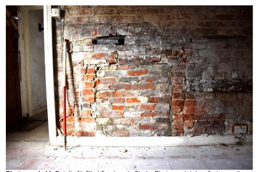
**Photograph 11** Detail of infilled fireplace in Study. Photograph taken facing northwest.
