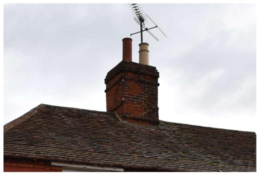
Photograph 3 Detail of original chimney. Photograph taken facing south-west.
