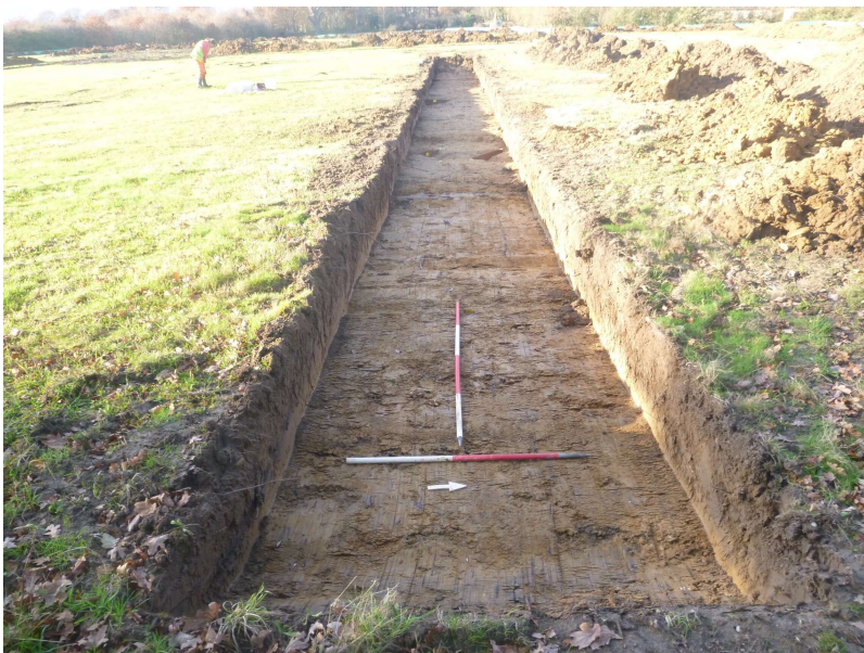
Photograph 1 T9 trench shot – looking west
