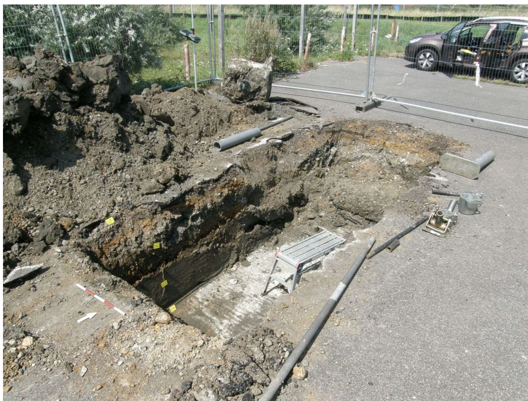
Photograph 3 Trench shot – view north-west
