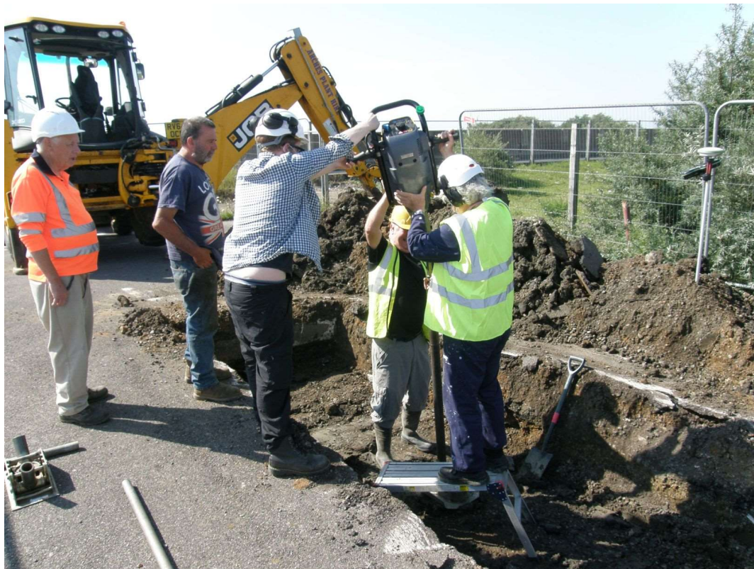
Photograph 2 Working shot – view south-west
