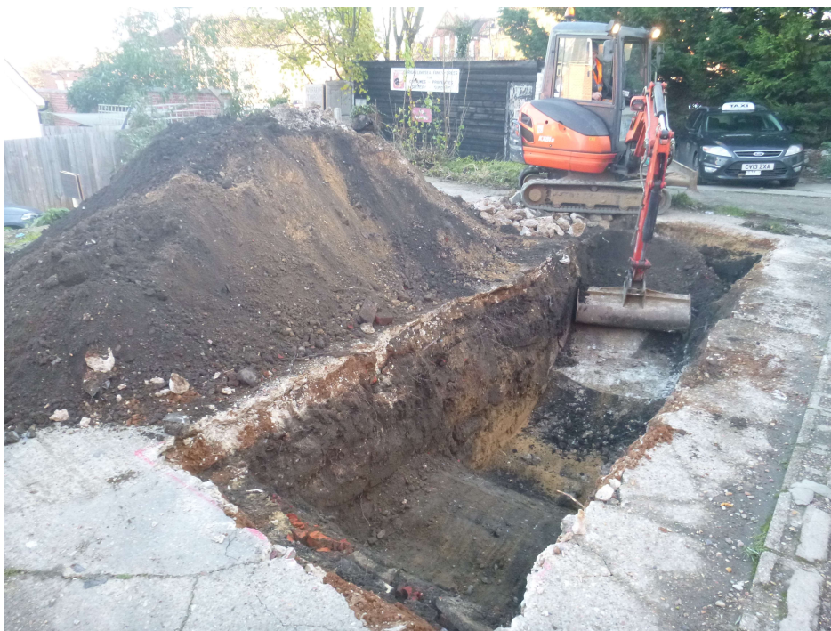
Photograph 1 Shot of trench during excavation, looking northeast.
