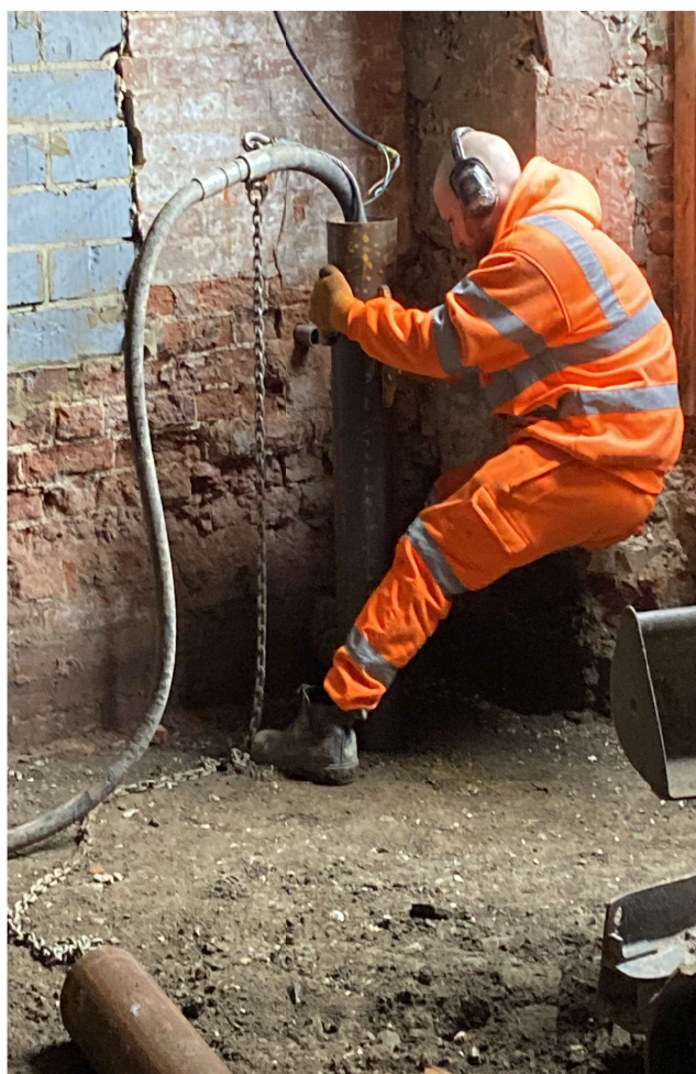
Photograph 4 Method of creating piles with pneumatic mole.
