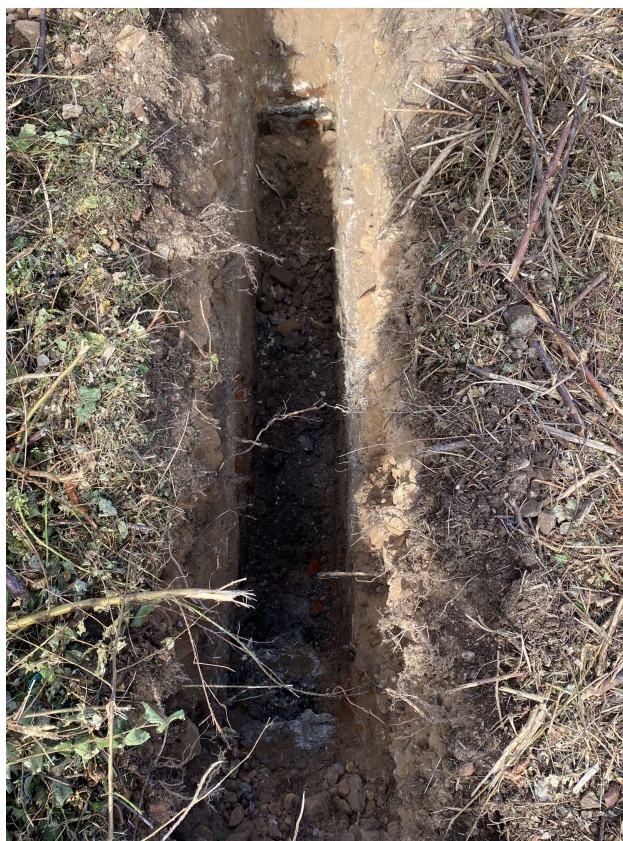
Photograph 1 F1 in TP02 – looking north
