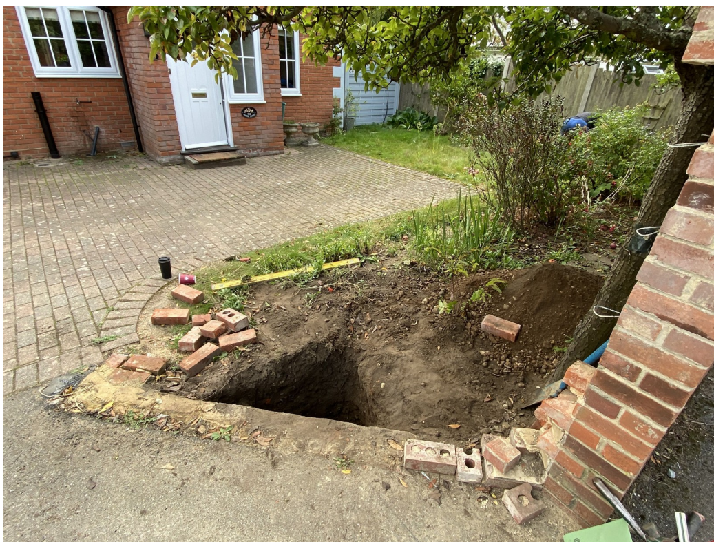
Photograph 2 South trench, looking south-east.
