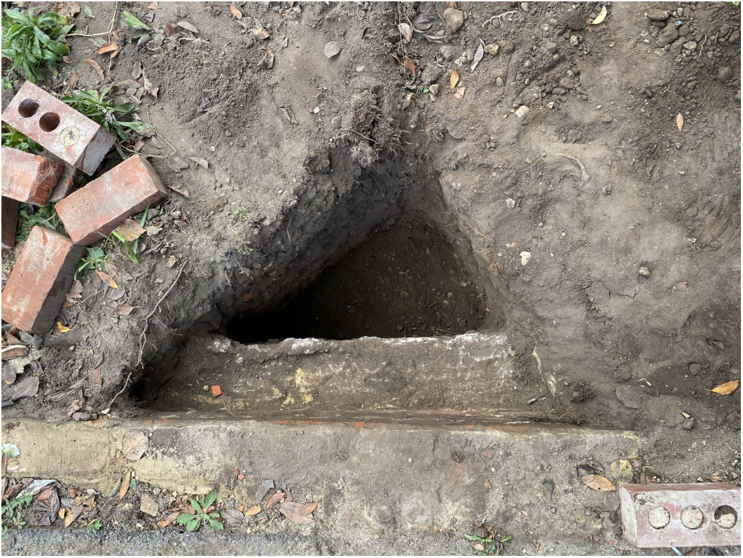
Photograph 4 South trench plan, showing concrete footing.
