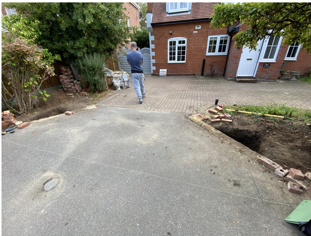
Photograph 1 General shot showing both trenches, looking east.
