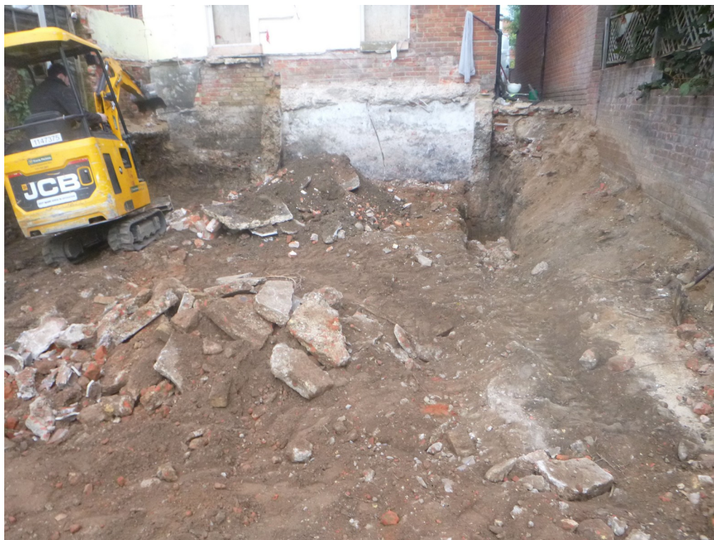
Photograph 1 General working shot, looking roughly west
