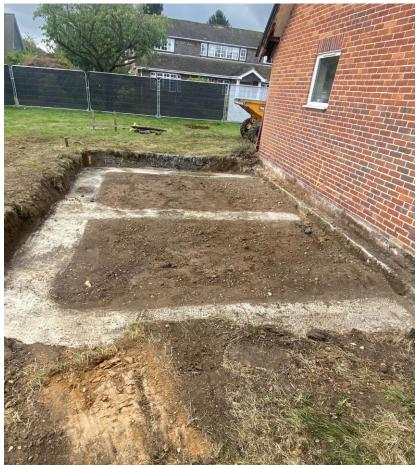
**Photograph 2** Completed excavation of footings on south-east side of property, with concrete, looking south
