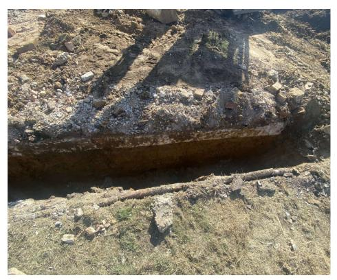
**Photograph 4** Excavation of footings on north-west side of property, showing concrete footings of former garage, looking west
