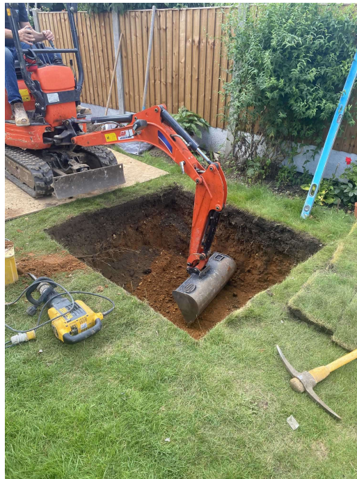
Photograph 3 Soakaway working shot, looking S
