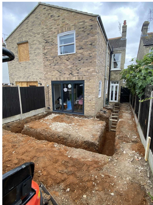
Photograph 1 Site shot showing completed foundation trench, looking east
