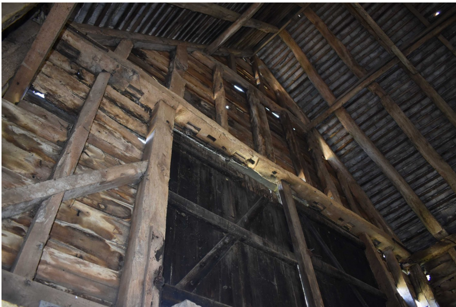
Photograph 12 Re-used timber wall-plate in midstrey. Photograph taken facing north-east.
