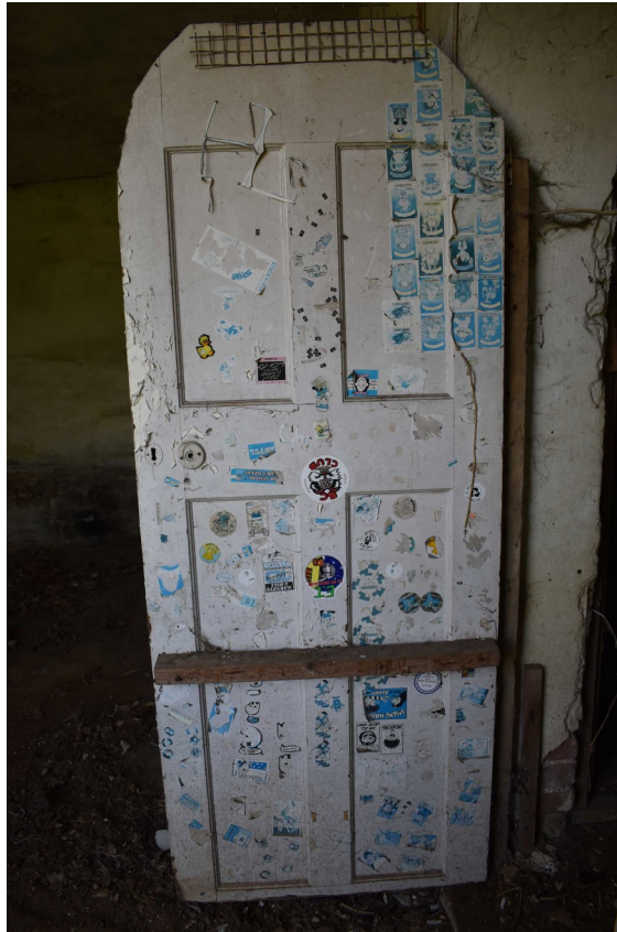
Photograph 22 Re-used door in garage. Photograph taken facing north-east.
