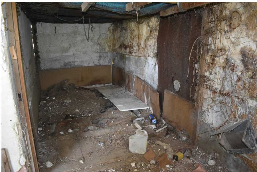
Photograph 23 Interior of lean-to. Photograph taken facing east.
