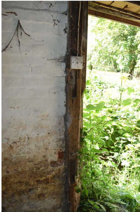
Photograph 24 Re-used timber in stable. Photograph taken facing south-west.
