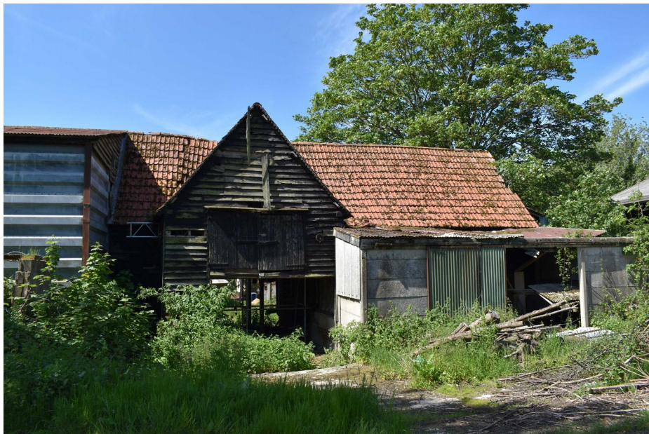
Photograph 3 North-east elevation of threshing barn. Photograph taken facing west south-west.
