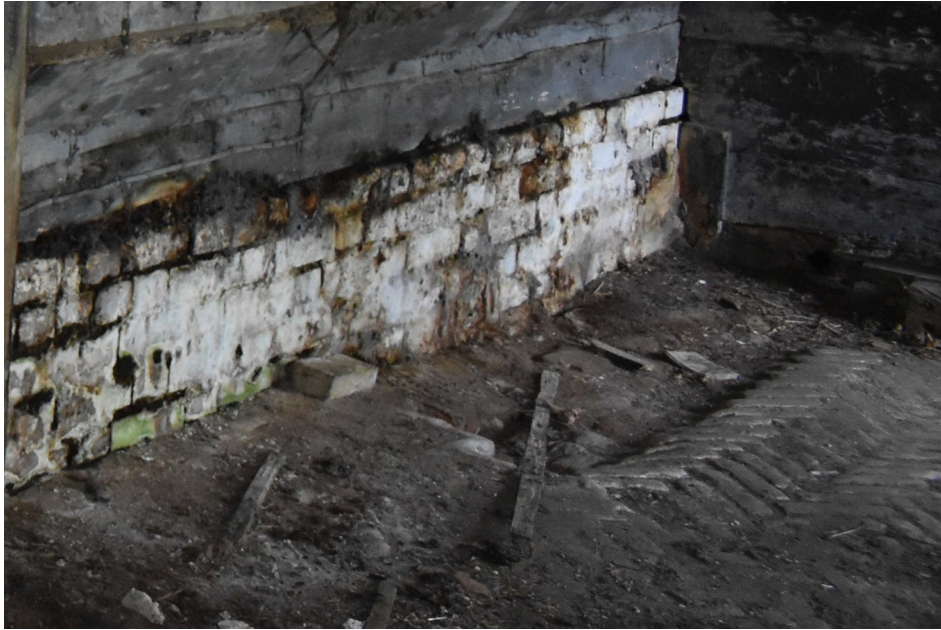
Photograph 18 Area of red brick flooring. Photograph taken facing east.
