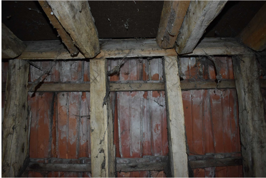
Photograph 16 carpenter's marks on rafters of coach house. Photograph taken facing north-east.
