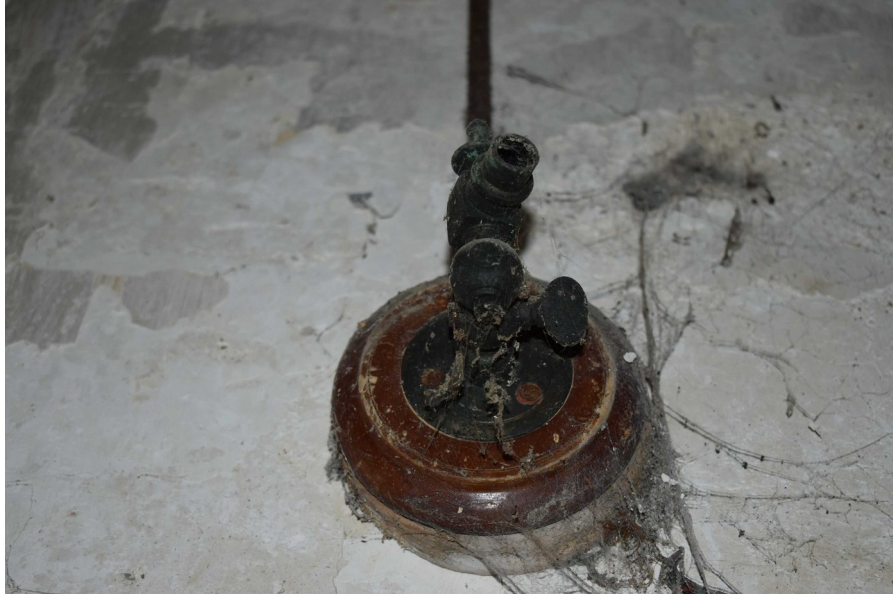
Photograph 20 Gas lamp mount in main room of coach house. Photograph taken facing south-west.
