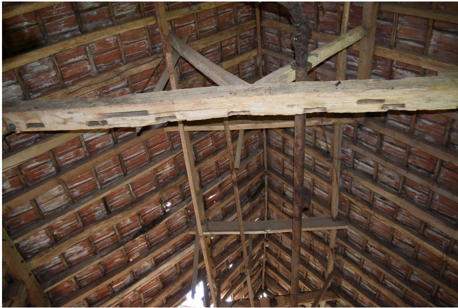
Photograph 4 Detail of tie-beam between bays 1 and 2. Photograph taken facing south-east.
