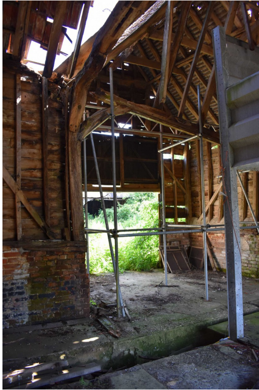
Photograph 8 Interior of threshing barn showing bay 3. Photograph taken facing east south-east.
