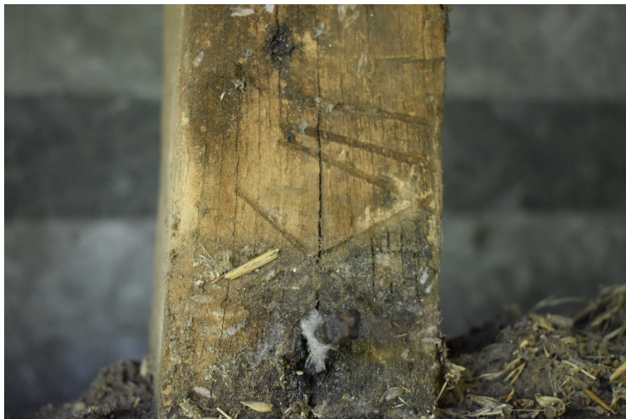
Photograph 11 Carpenter's marks on stud of bay 4. Photograph taken facing north-east.
