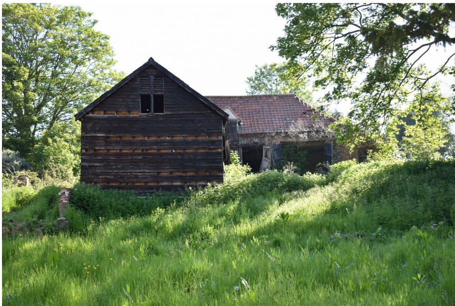
Photograph 14 South-west elevation of coach house. Photograph taken facing north-east.
