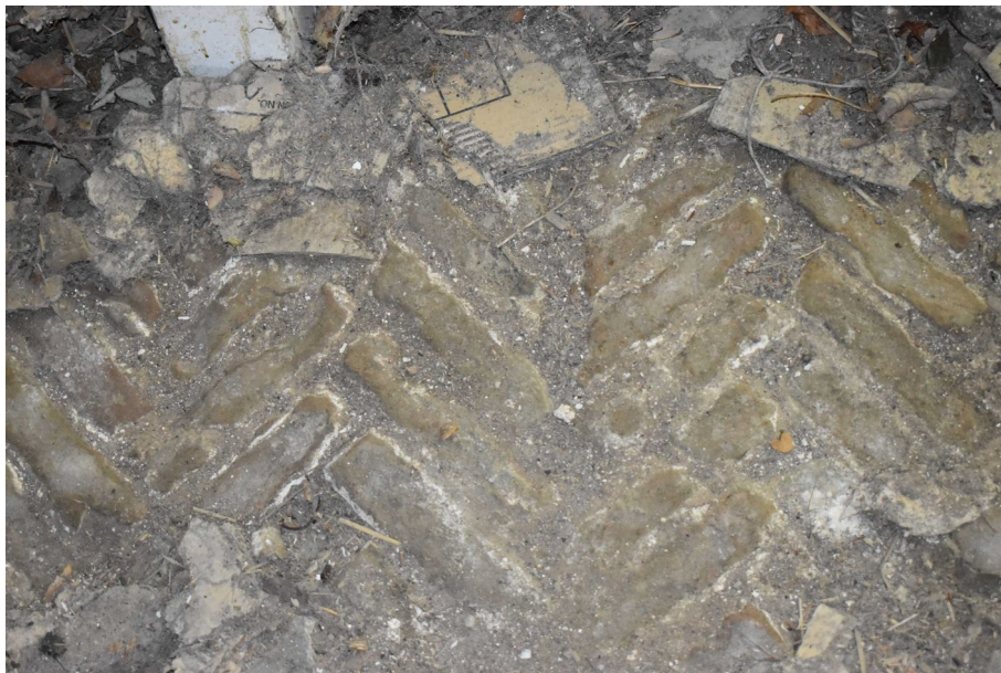
Photograph 17 Detail of herringbone brick floor in coach house. Photograph taken facing south-east.
